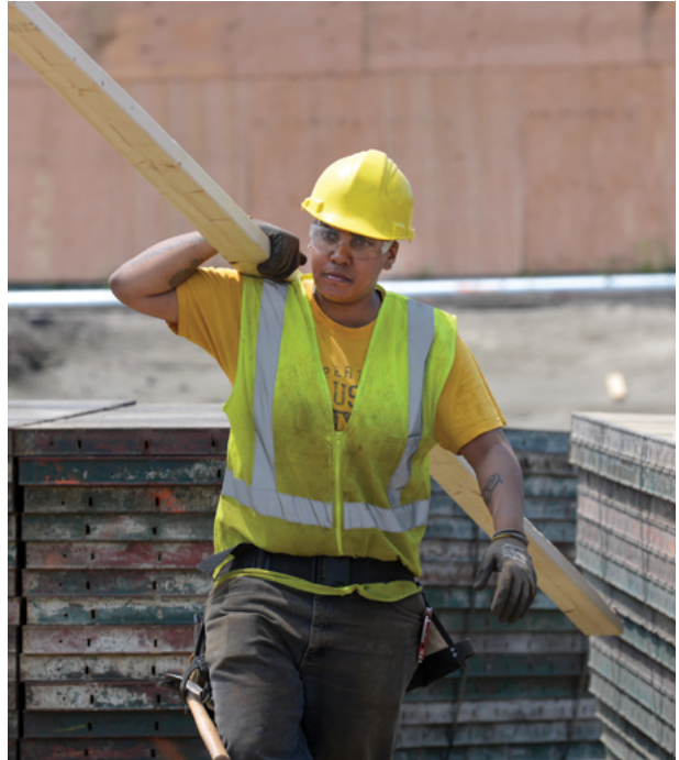
MGM Springfield construction.
