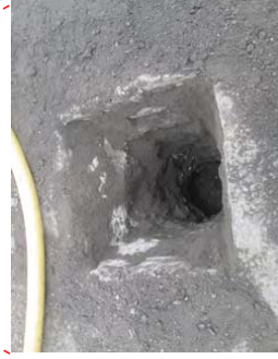
TEST PIT 8 450' N of Spruce St.; 6' off E curb
