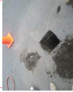
TEST PIT 6 100' N of Market St.; 7' off E curb
