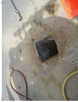
TEST PIT 2 350' N of Market St.; 12' off E curb
