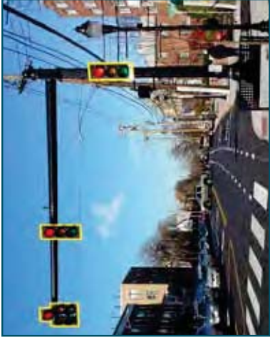
Retro-reflective Signal Head Backplate
