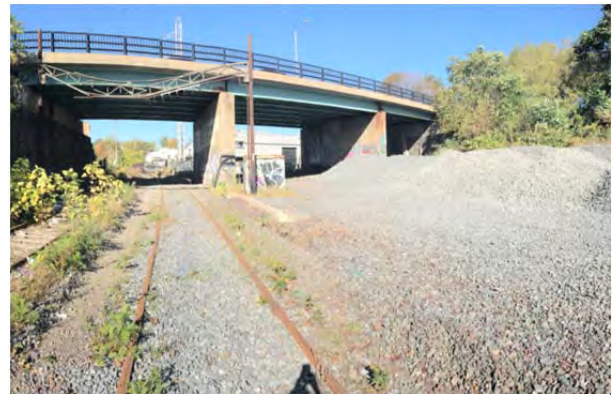
MBTA ballast storage under the Route 16 and Route Connector overpasses.
