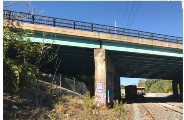
First and second span of Bridge E-12-005, looking
