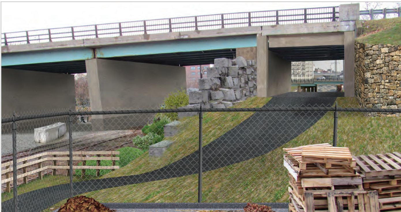
Option for the trail to pass through the second span of the bridge, requiring earthwork and a potential culvert.
