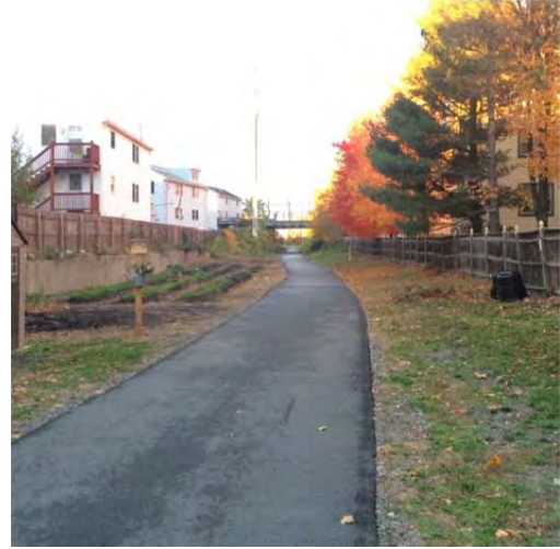
Existing paved portion of the Northern Strand Community Trail in Everett.
