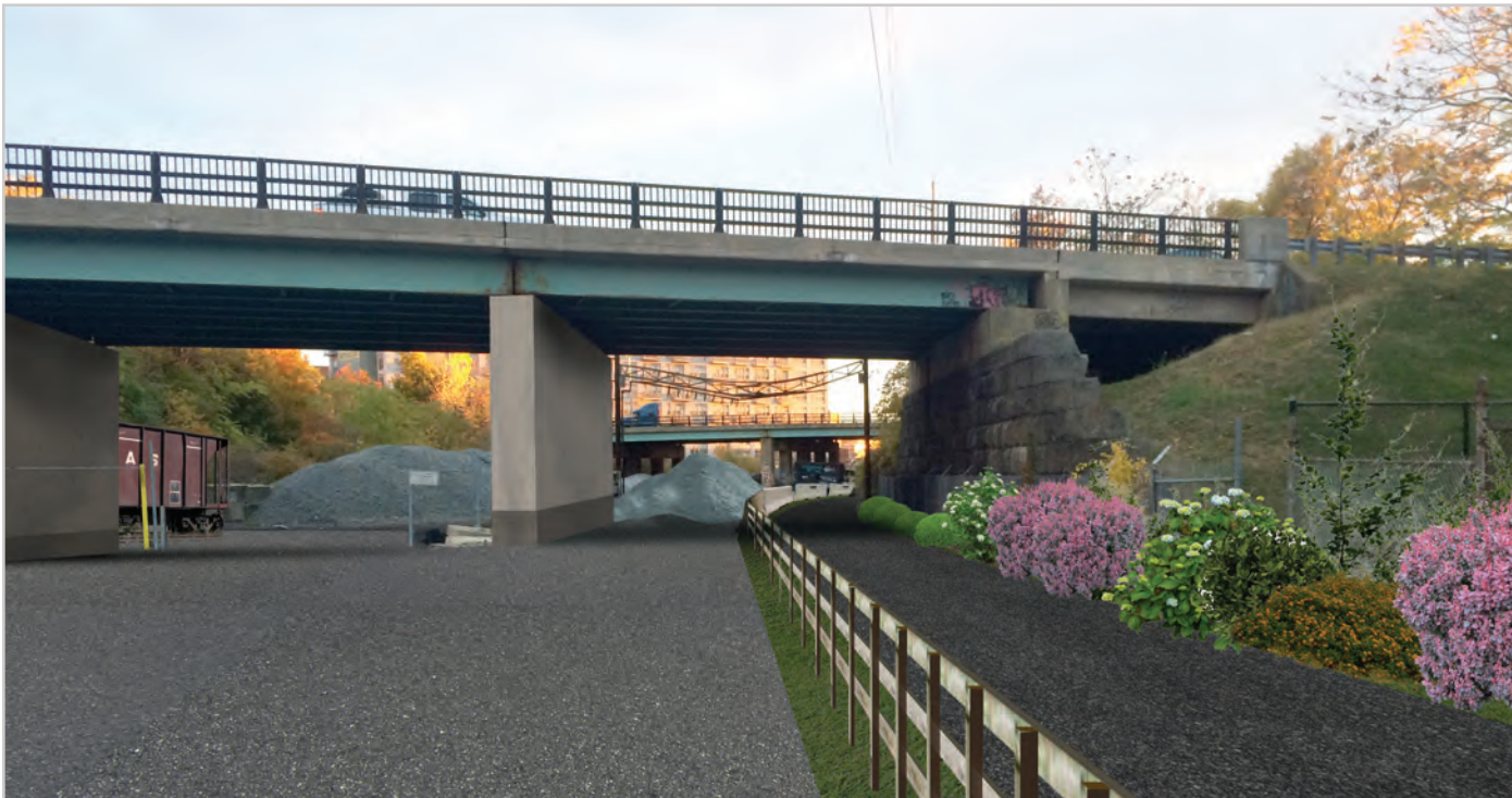
Option for the trail to pass through the second span of the bridge, shifting the existing tracks.
