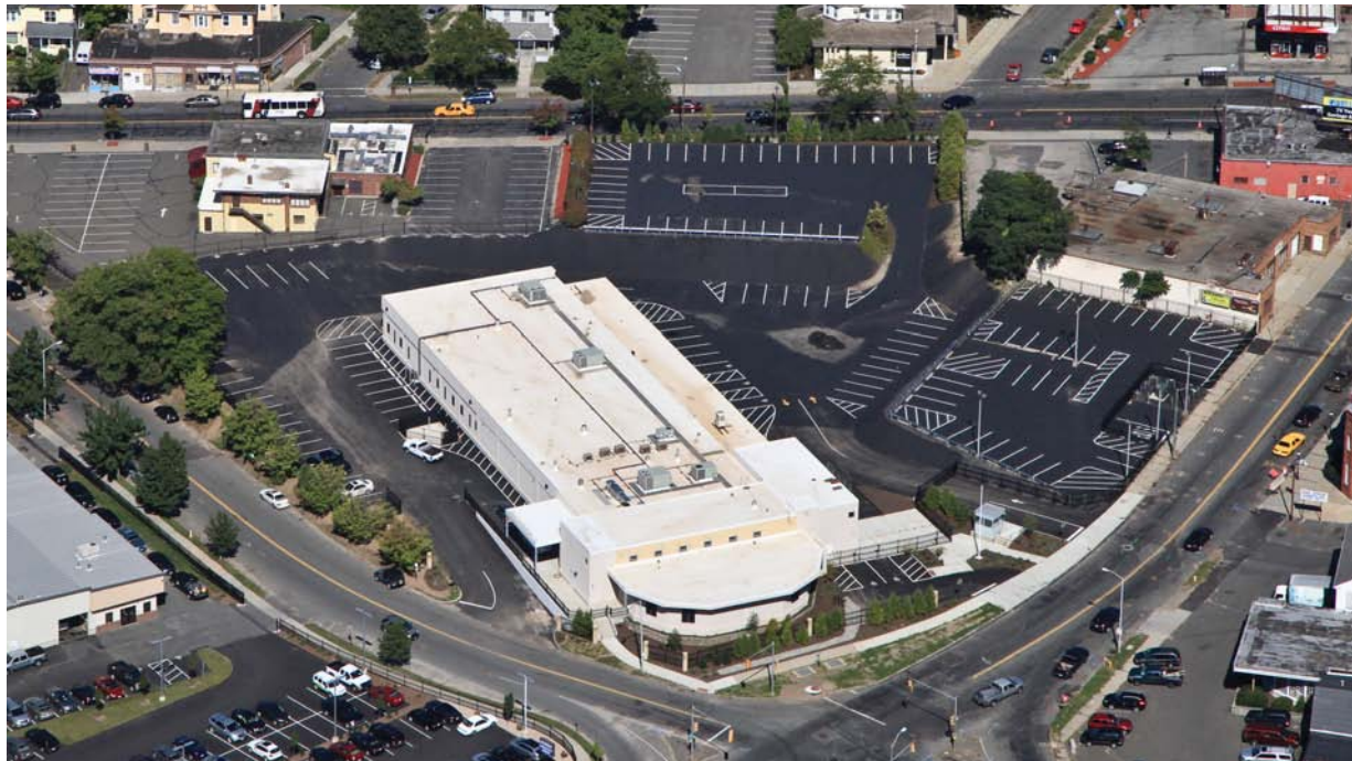
09-23-15 Aerial Over Completed Mission
