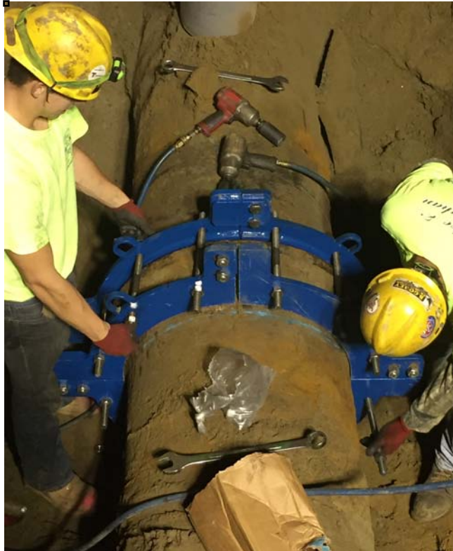
11/10/15 Offsite Utilities - Union Street
