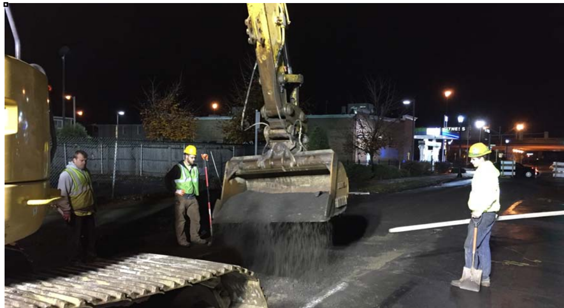
11/13/15 Offsite Utilities - Patching Union Street
