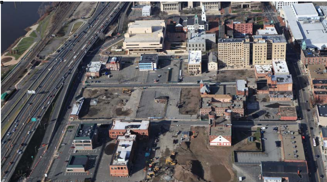
12/26/15 Site Aerial Showing Church Haul Road Progress.
