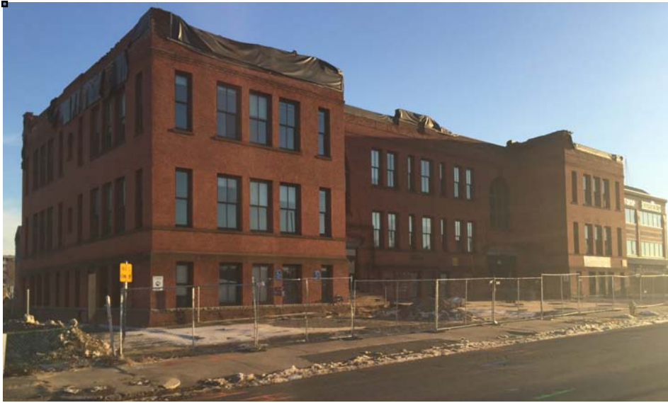
Zanetti School Ready for Demolition Planned for 1/11/16
