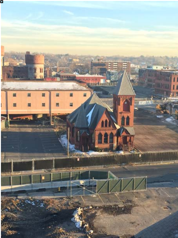
French Church Ready for Relocation
