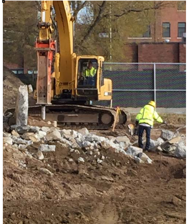
12/1/15 French Church Haul Road Construction
