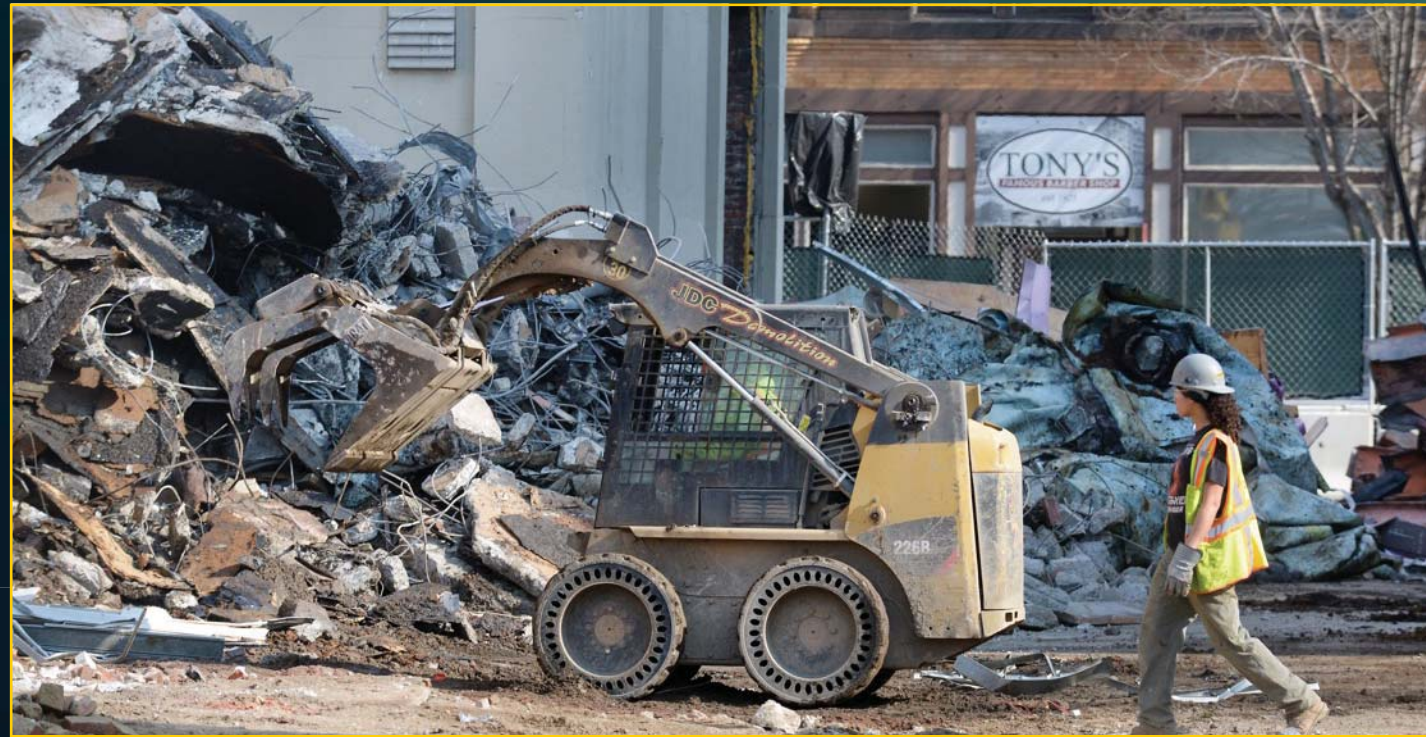
Main Street Demolition and Recycling - March 8, 2016
