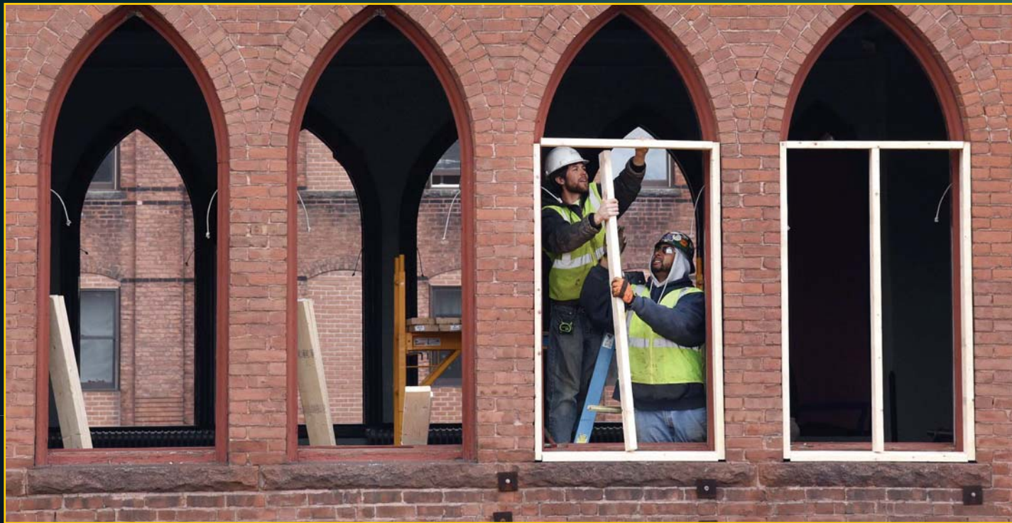
Workers bracing Church for move - March 18, 2016
