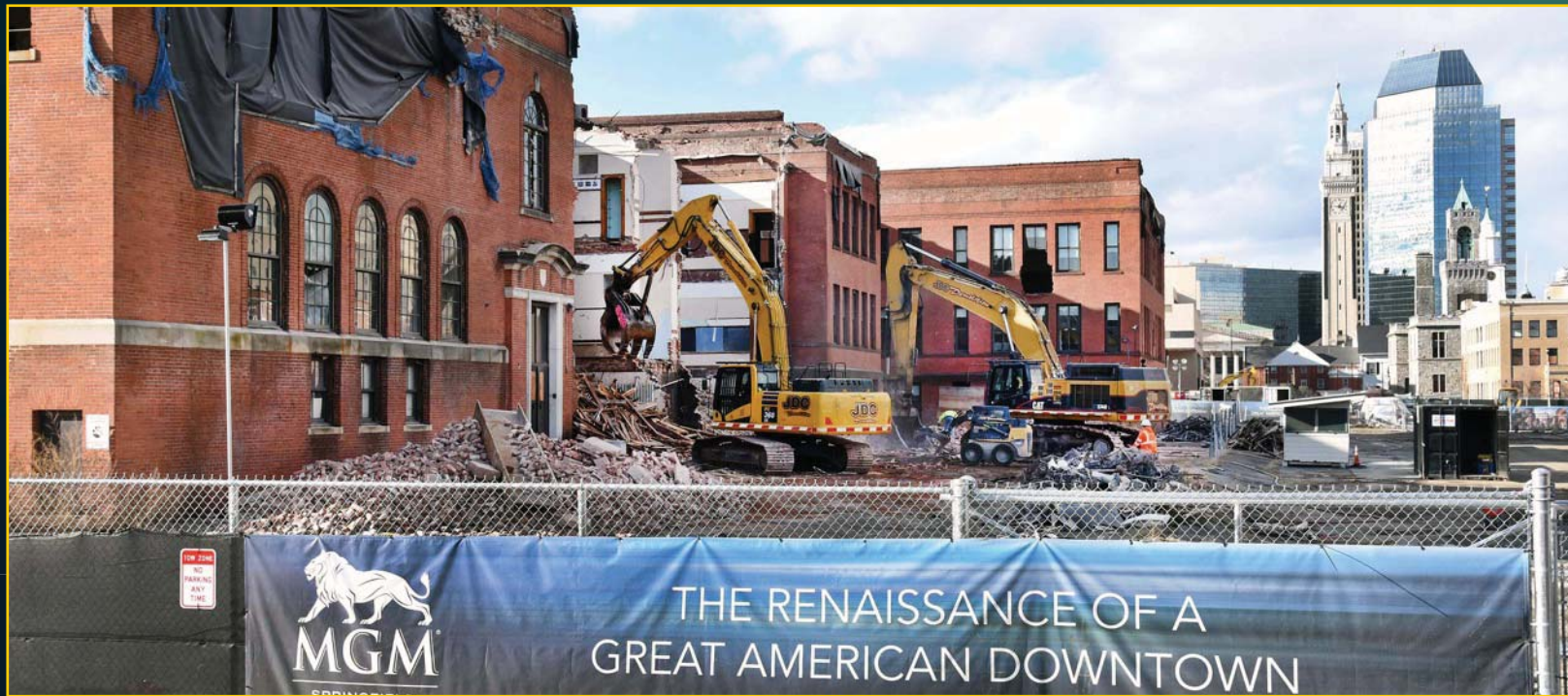
Howard Street School Demolition - January 11, 2016
