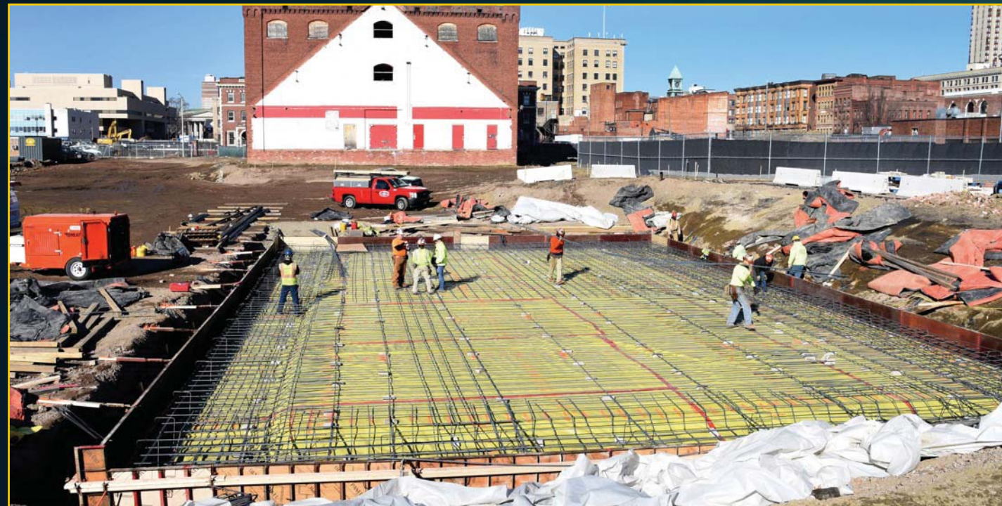
Preparing new Church foundation - January 28, 2016
