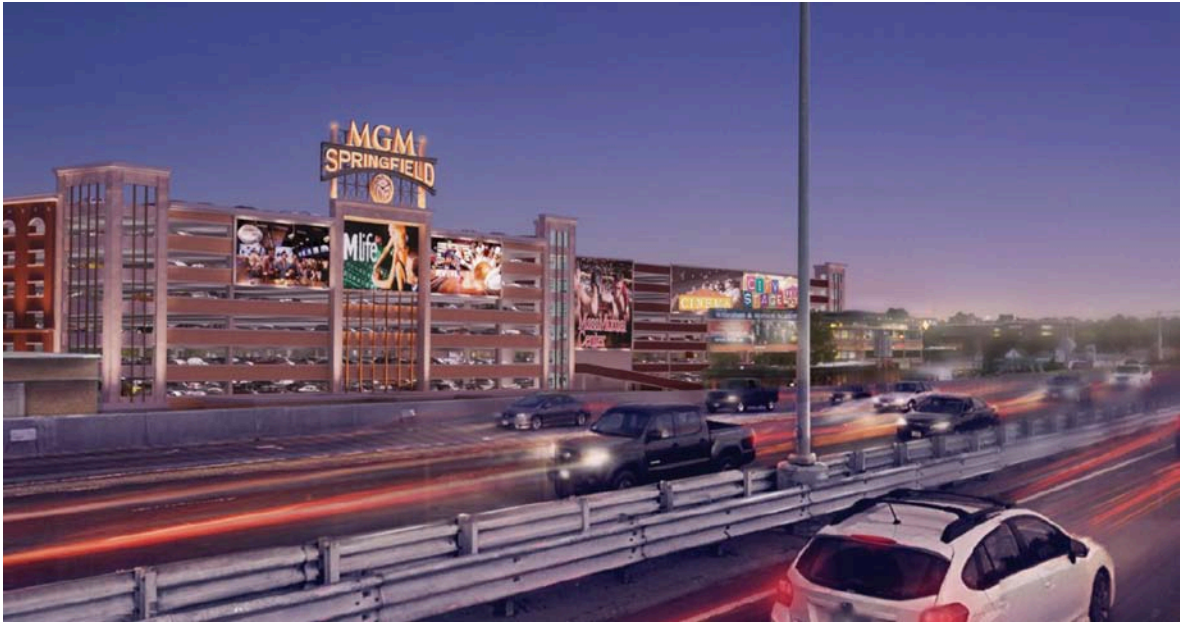
View of Garage and Signage from I-91
