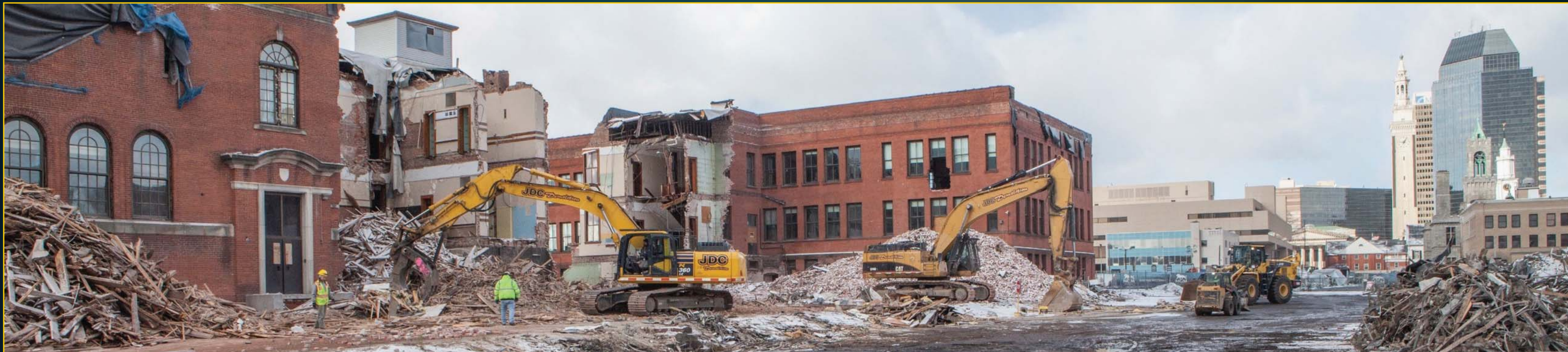
Howard Street School Demolition - January 21, 2016
