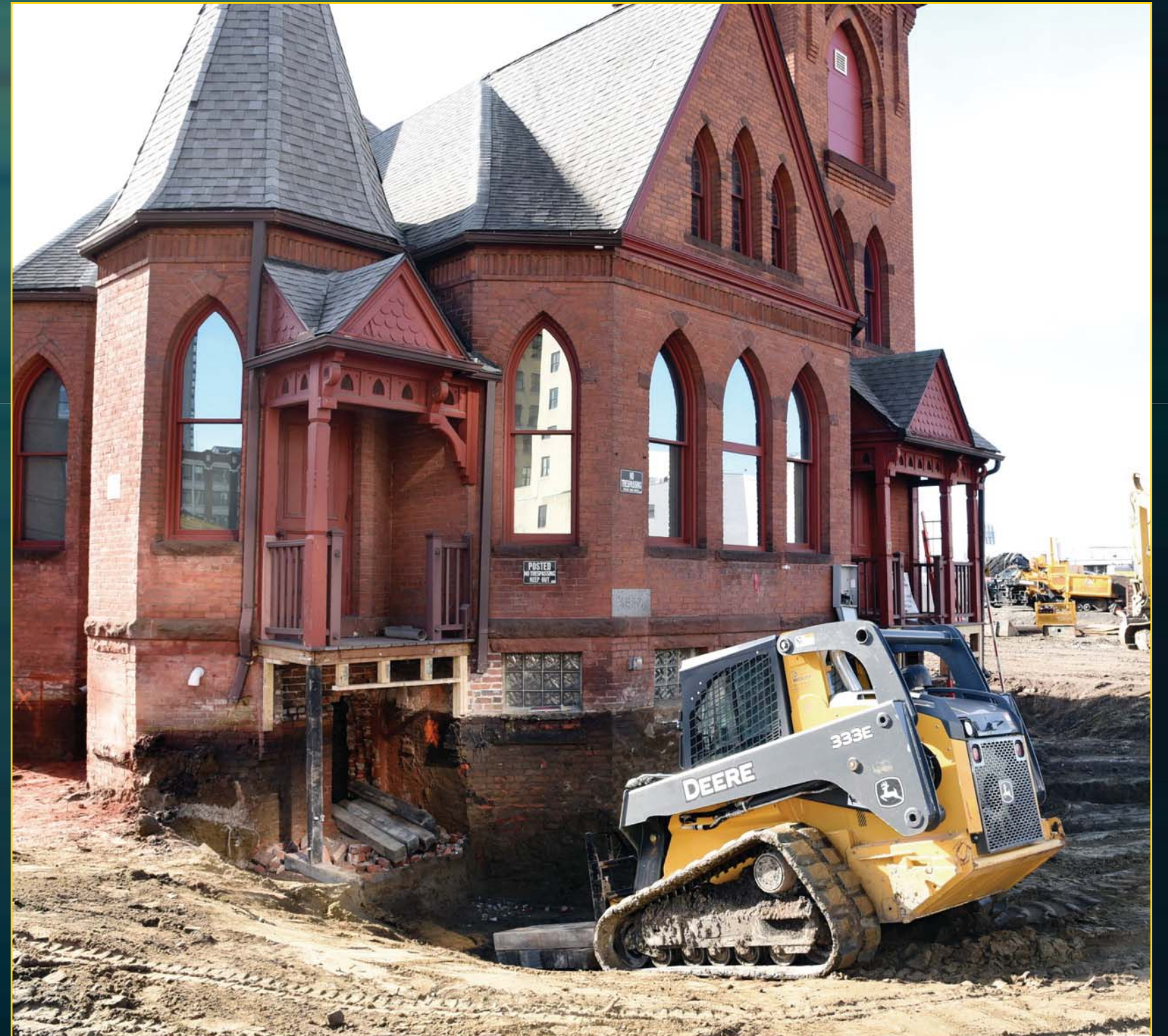
Clearing soil from Church foundations - March 16, 2016
