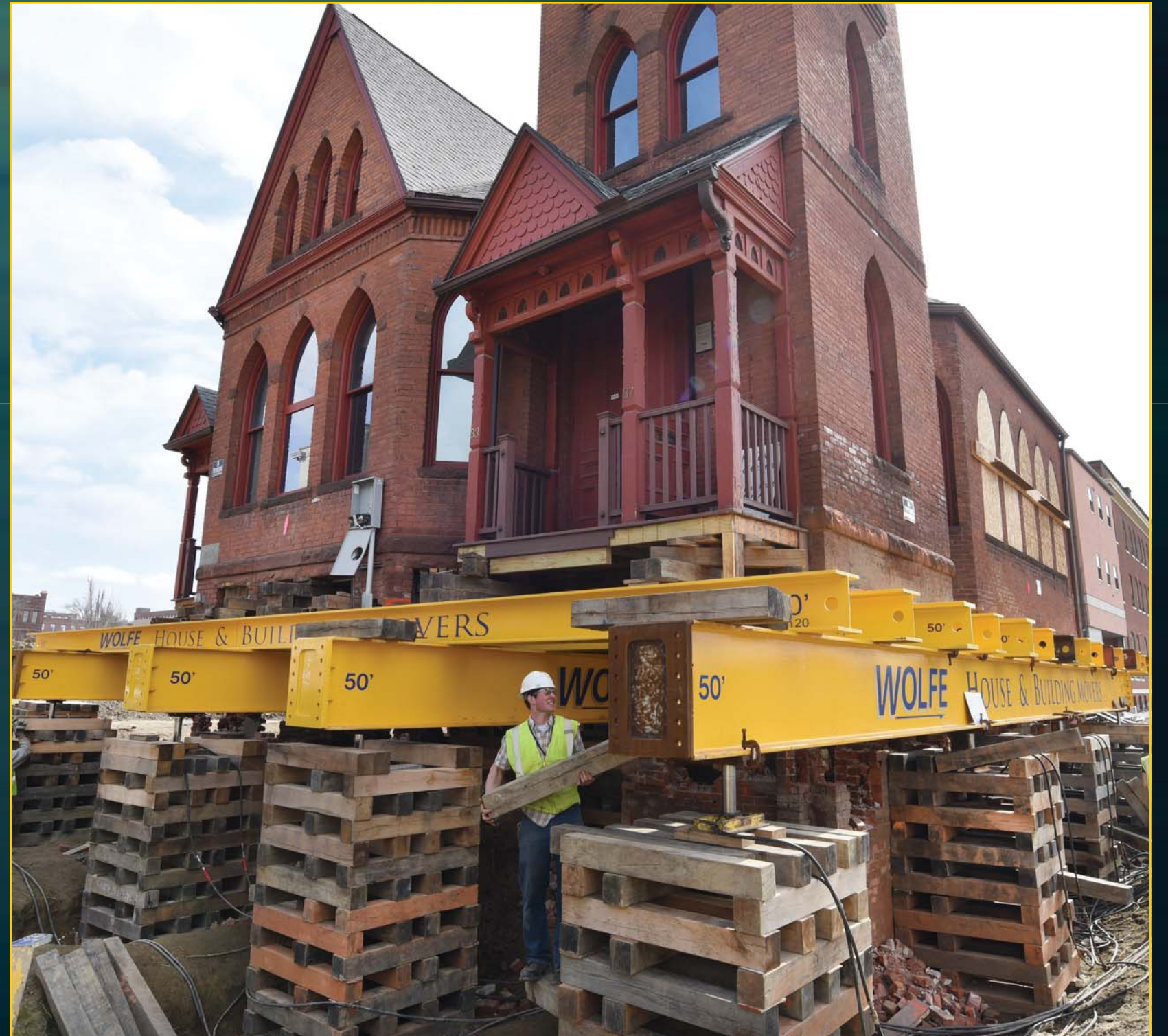
Lifting Church for relocation - March 31, 2016
