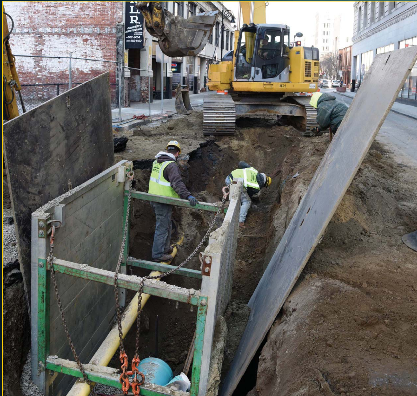
Offsite Utility Work - January 14, 2016
