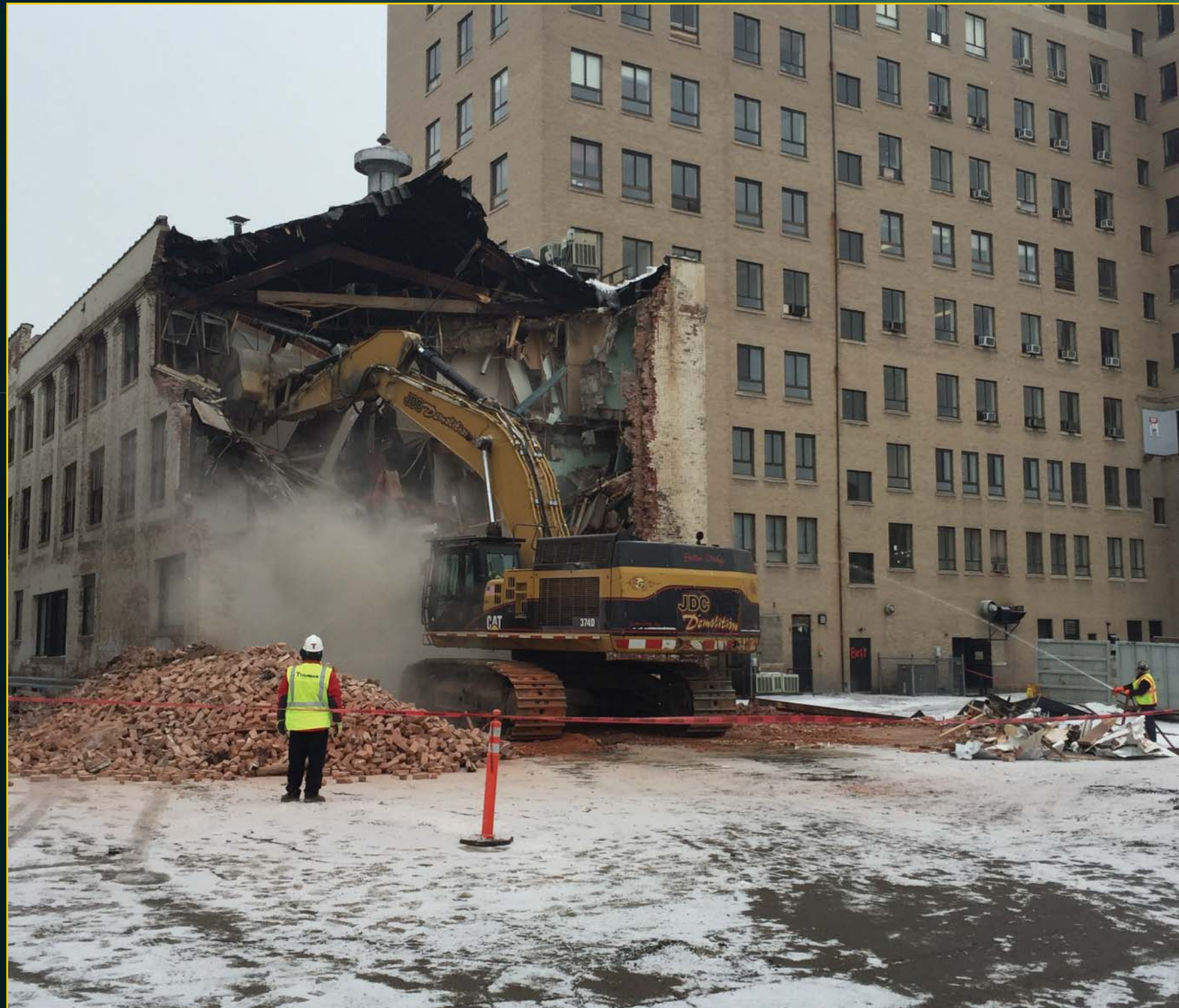
79 State Street Demolition - February 15, 2016
