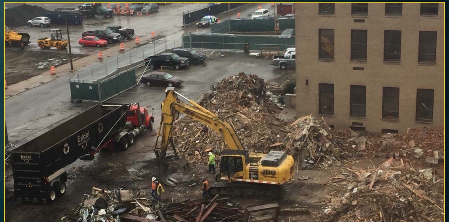
79 State Street Demolition - February 24, 2016
