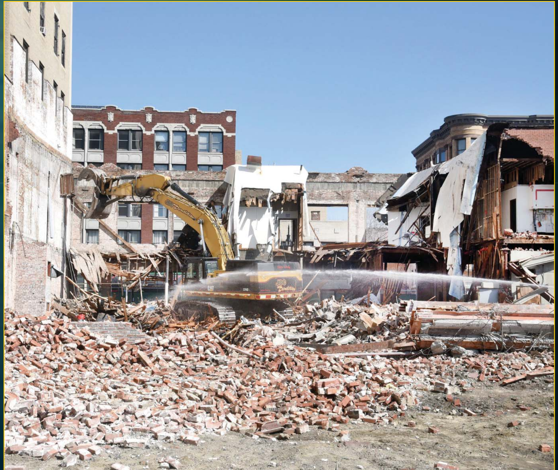
Edisonia Block Demolition - March 9, 2016
