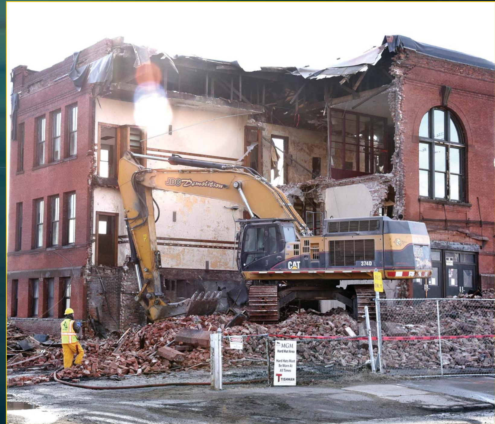
Howard Street School Demolition - January 27, 2016
