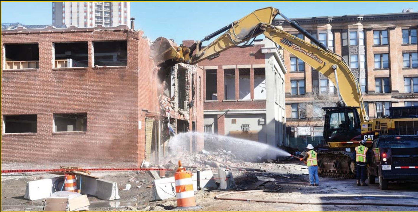
Bliss Street Demolition - March 3, 2016
