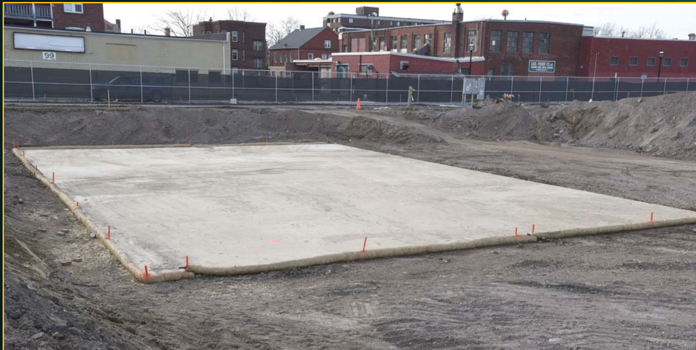
New foundation pad for Church - March 24, 2016
