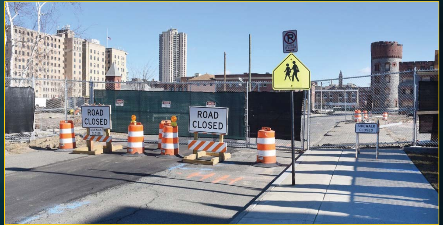
Howard Street Closure - March 3, 2016
