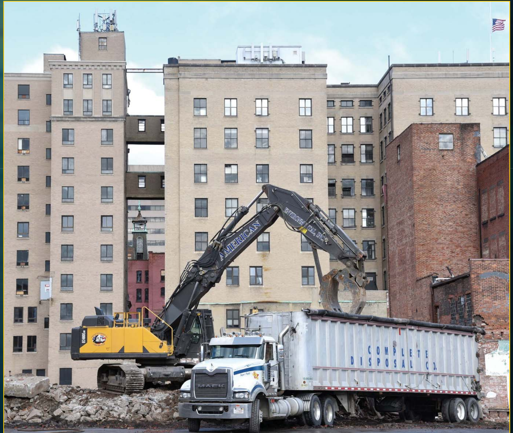
Bliss Street Demolition - March 18, 2016
