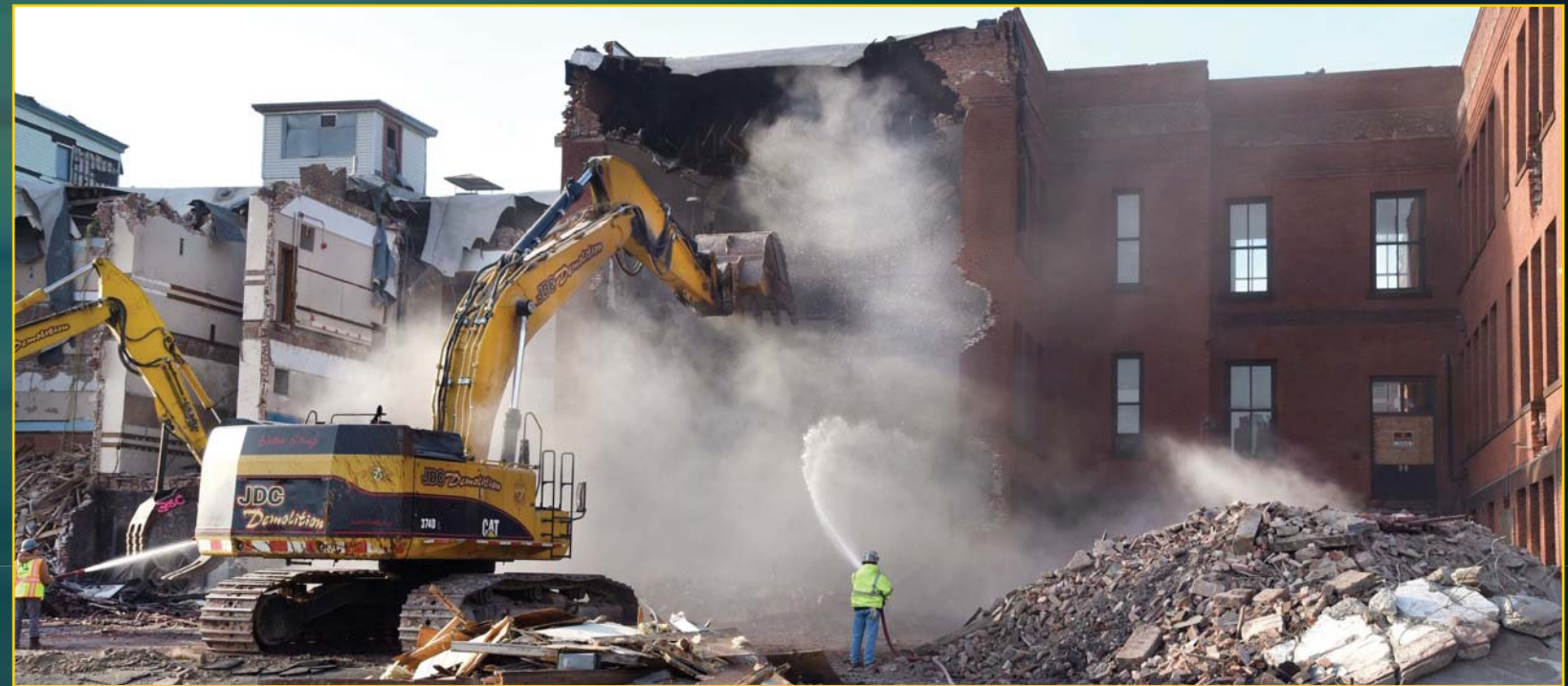
Howard Street School Demolition - January 12, 2016
