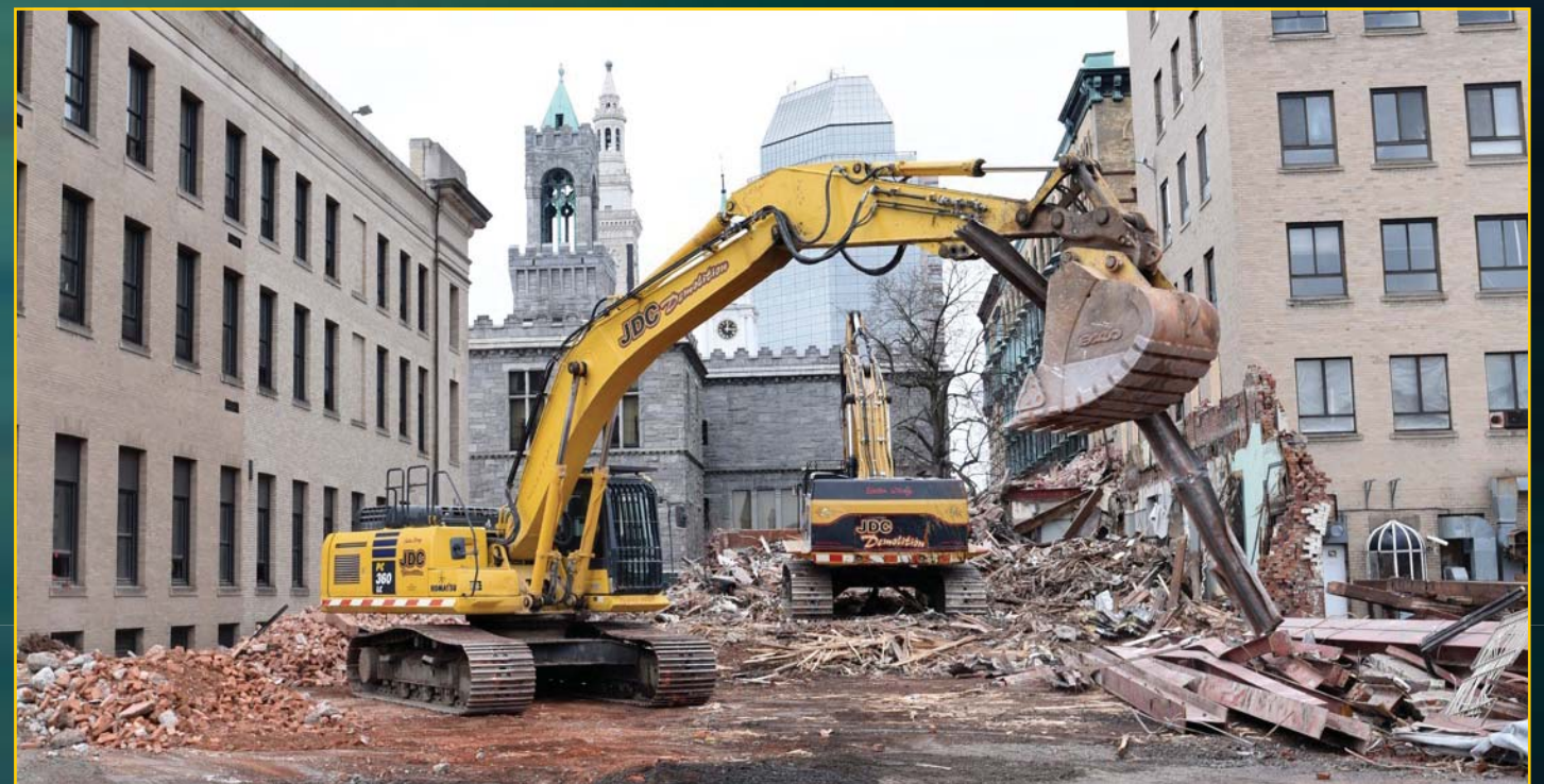
81 State Street Demolition - February 17, 2016
