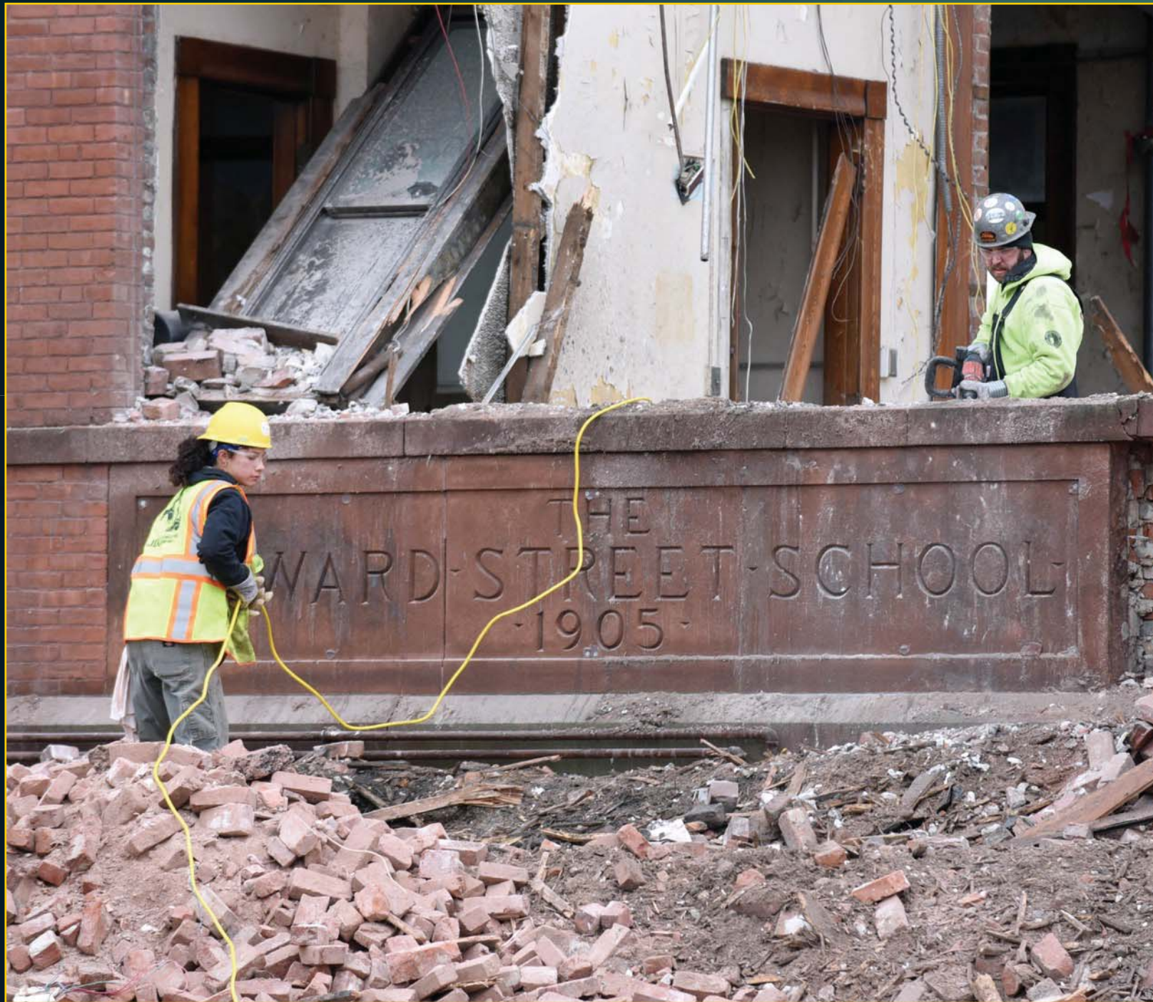
Howard Street School Demolition - January 26, 2016
