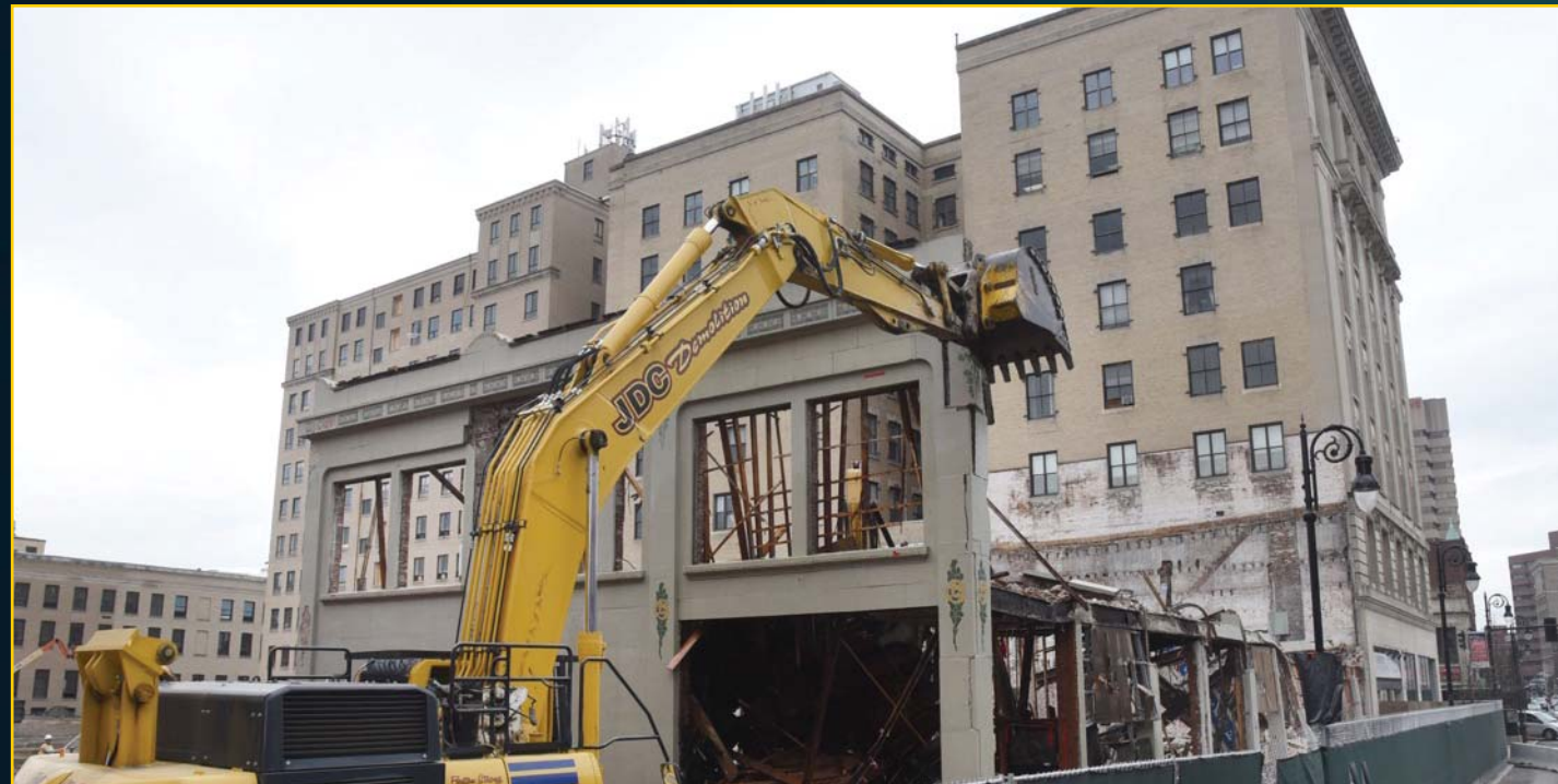
1156 Main Street Demolition - March 10, 2016
