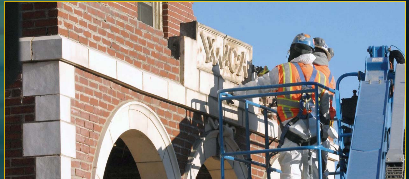
YWCA Building Salvage - January 25, 2016
