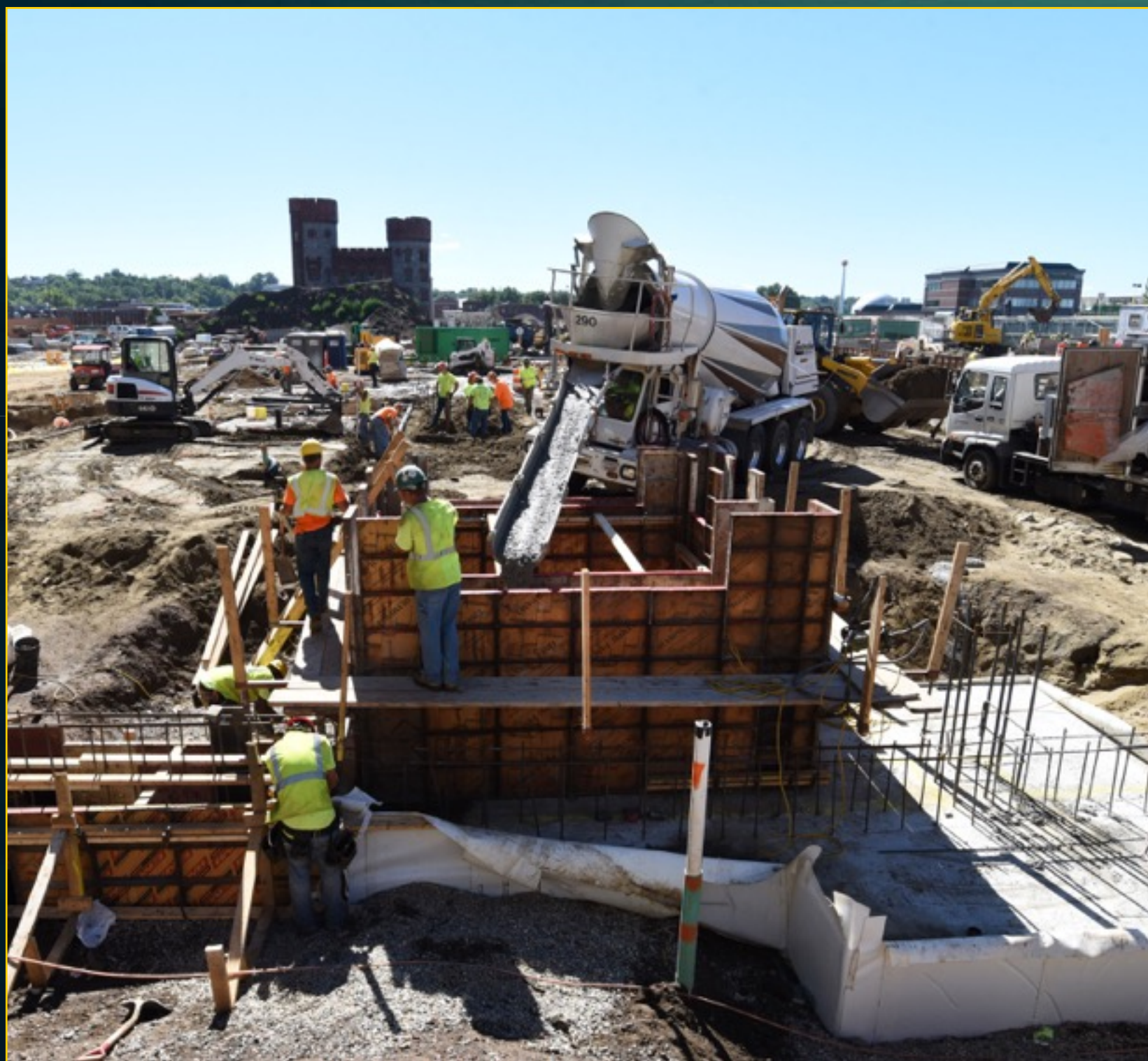
Podium Construction - August 22, 2016
