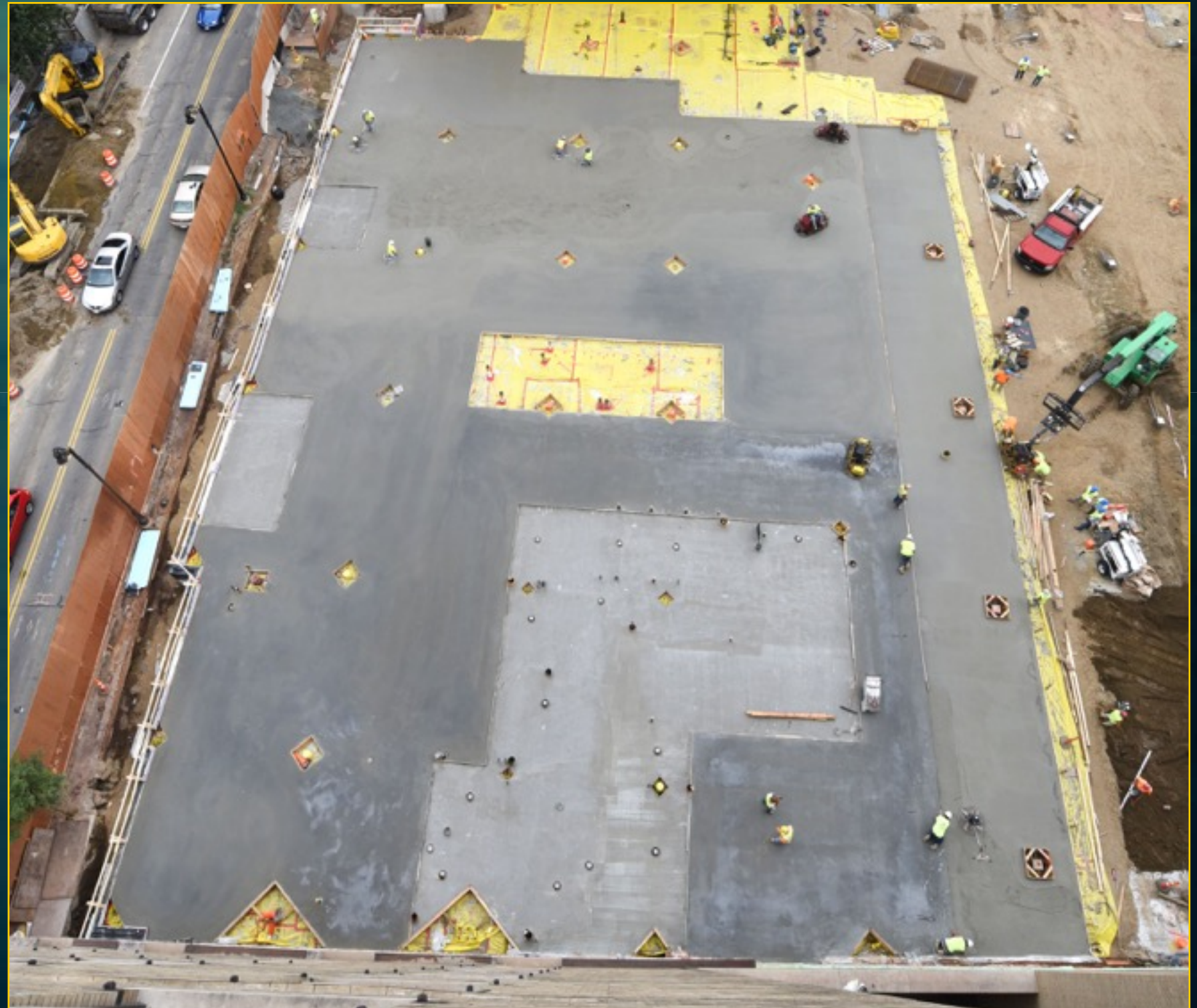
Hotel Foundation - August 17, 2016
