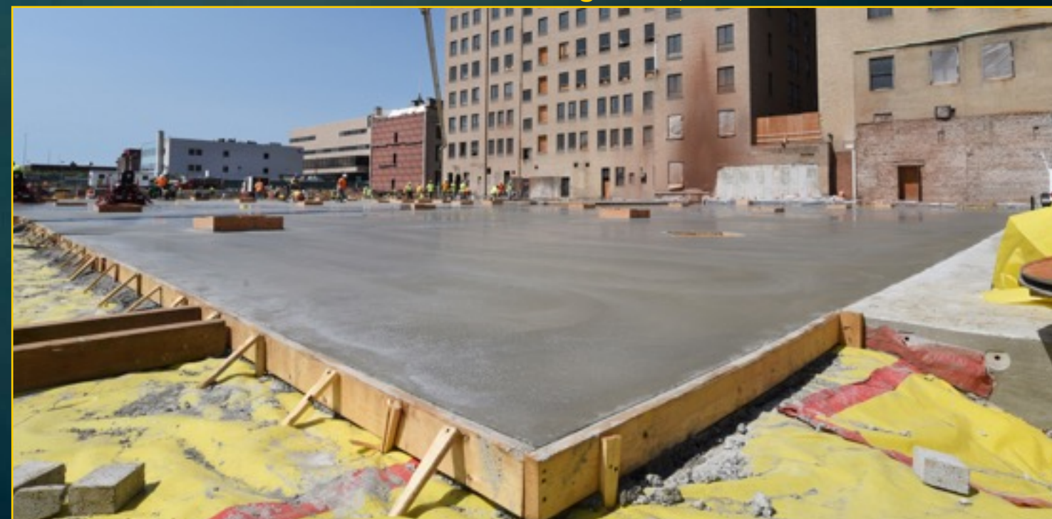
Podium Construction - August 24, 2016
