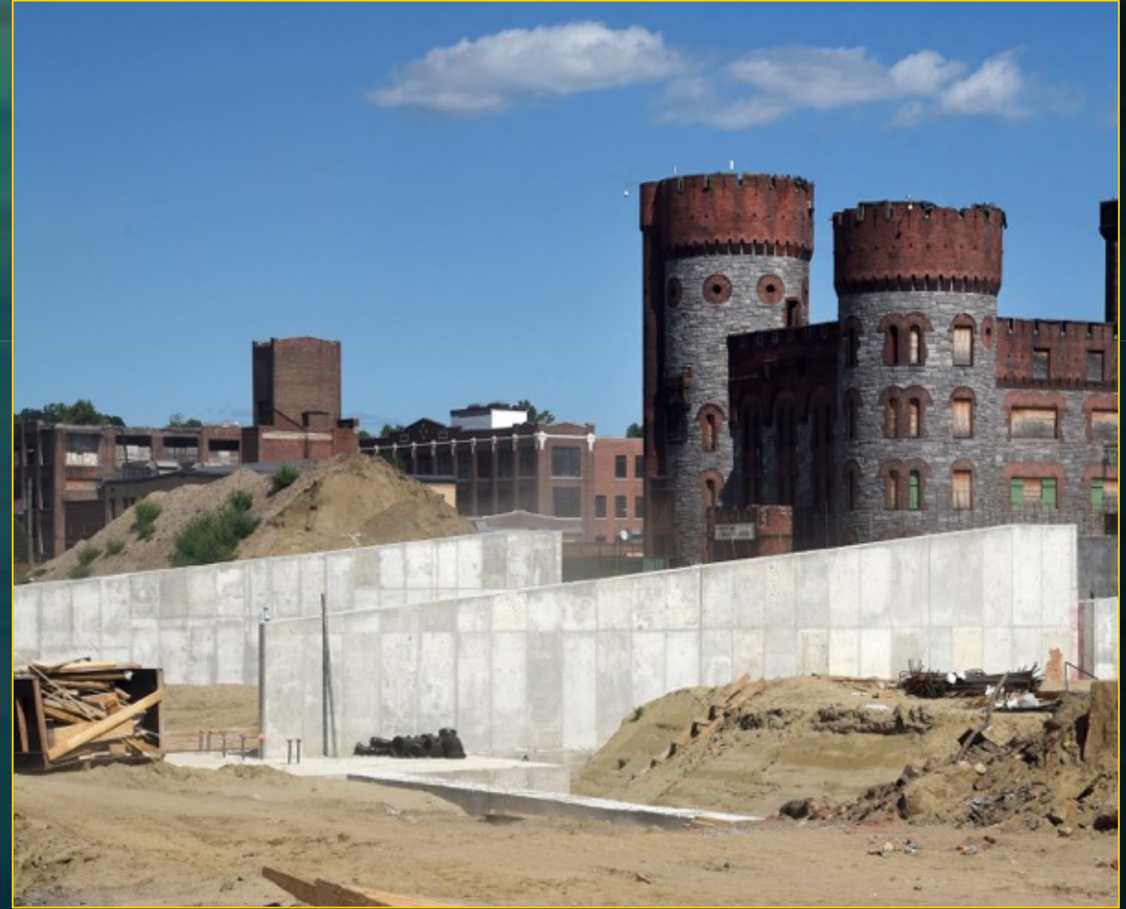
Garage Construction - August 29, 2016
