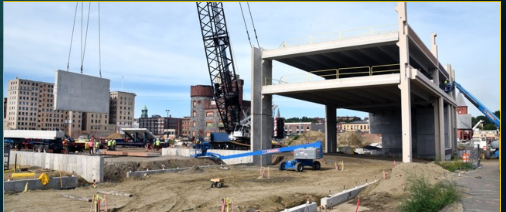
Garage Construction - September 22, 2016
