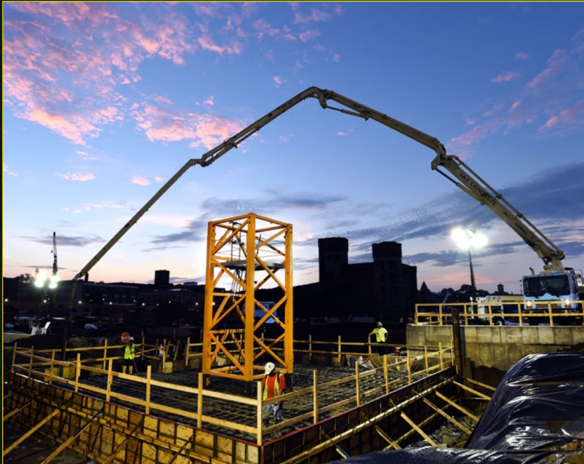
Foundation Construction - August 13, 2016
