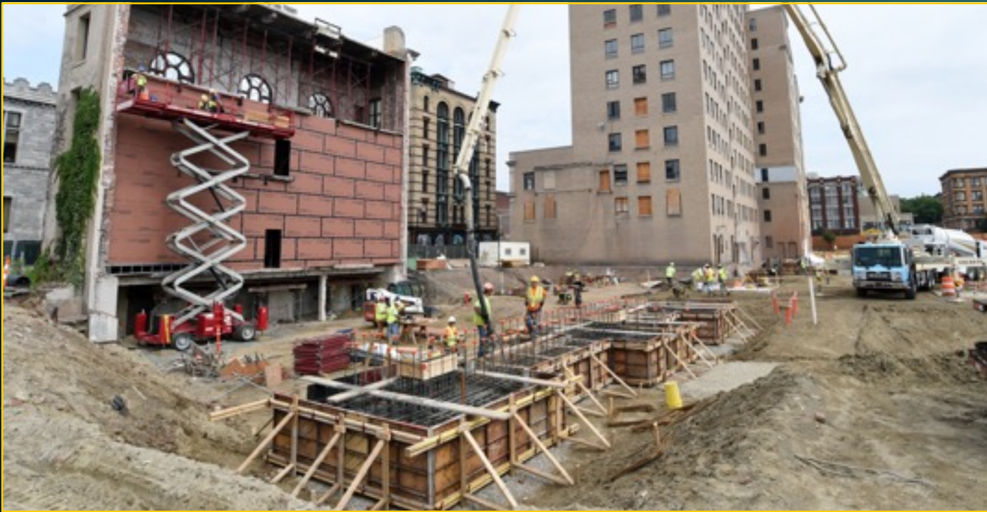
Podium Construction & 73 State Facade - August 16, 2016
