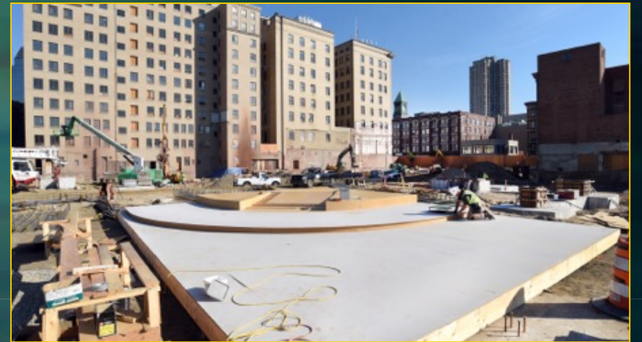
Podium Construction - July 28, 2016
