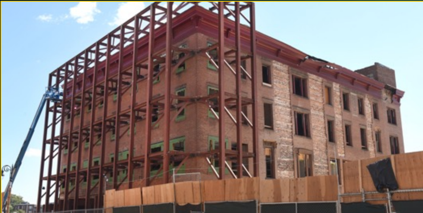
Union Chandler Facade Stabilization - August 29, 2016
