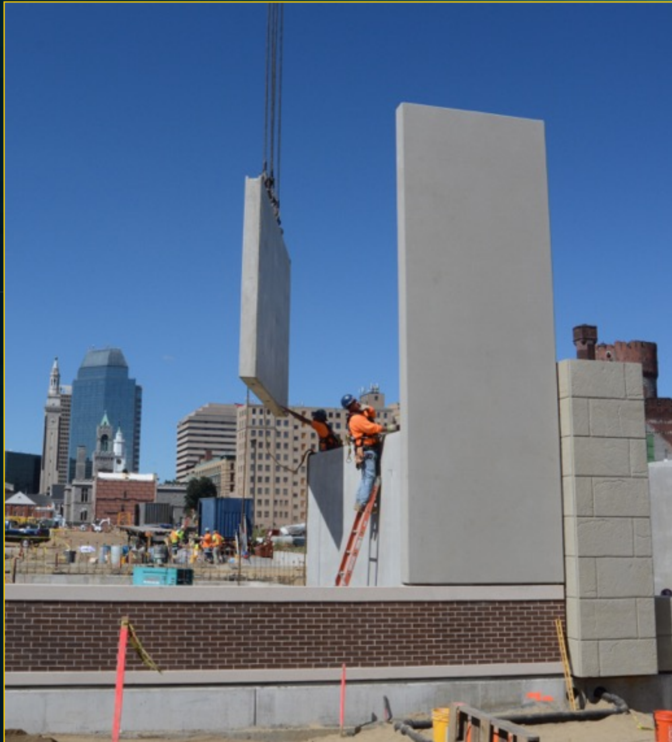
Garage Construction - September 15, 2016
