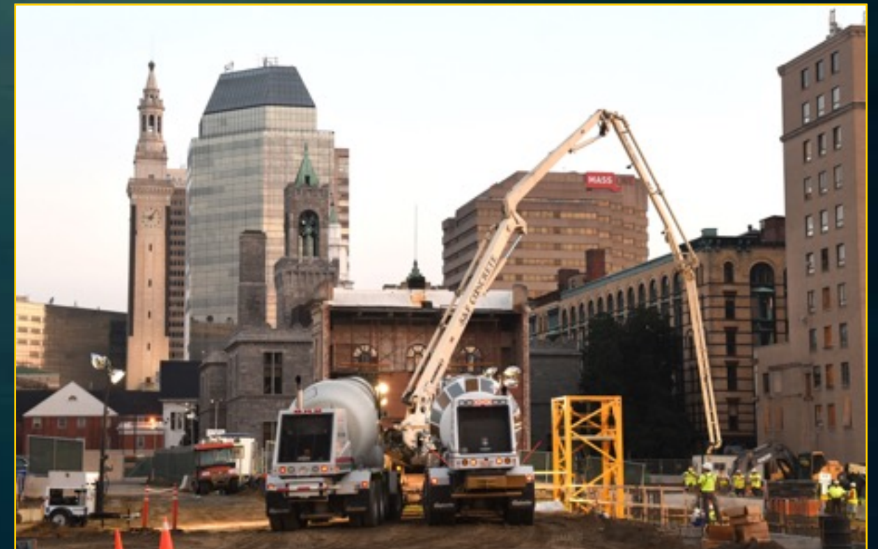
Foundation Construction - August 13, 2016
