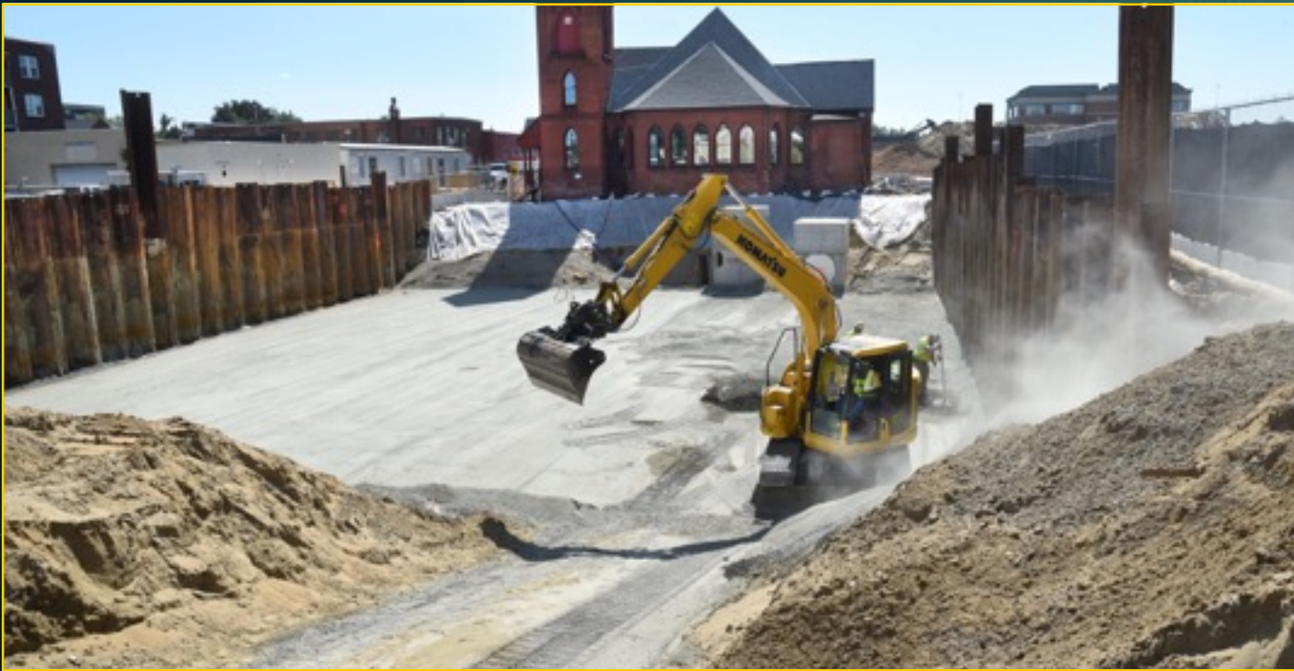
Excavation and Sub-Grading - August 29, 2016
