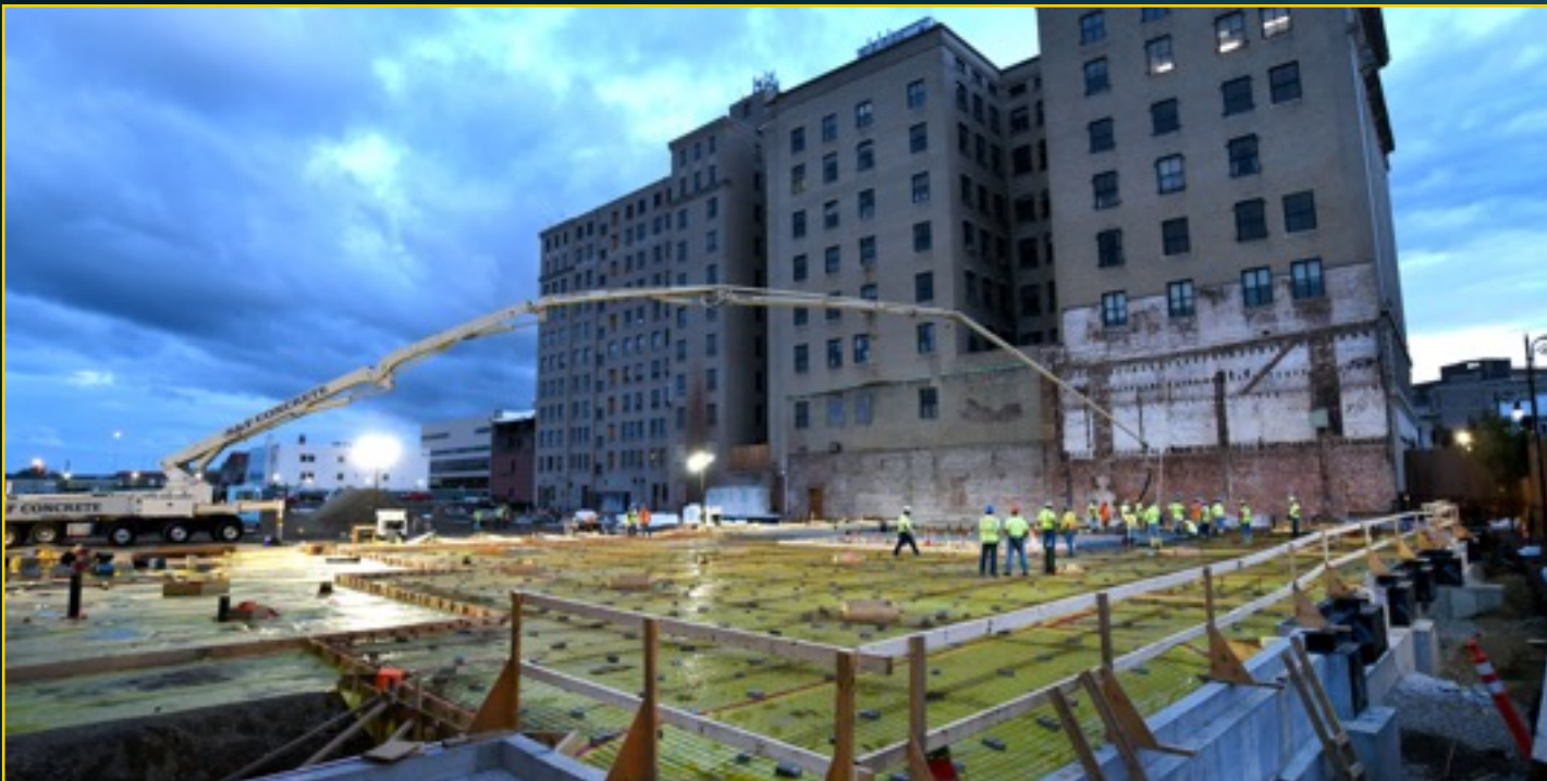
Foundation Construction - August 17, 2016
