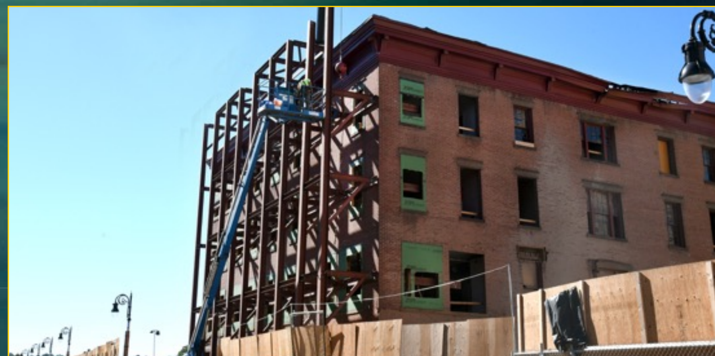
Union Chandler Facade Stabilization - August 22, 2016
