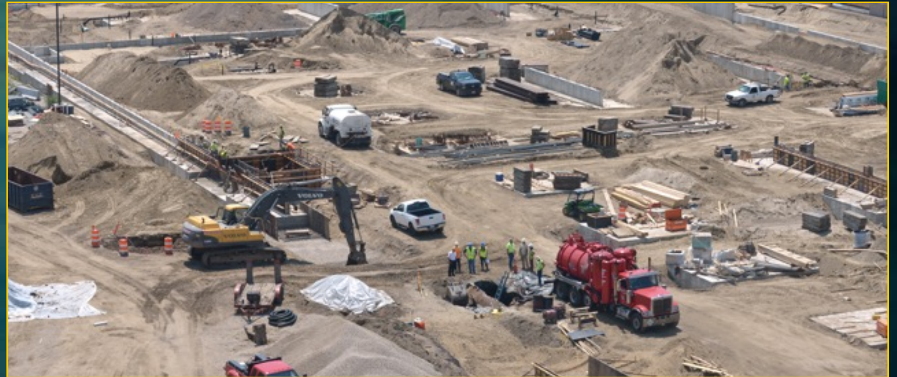
Oil Tank Removal - July 13, 2016
