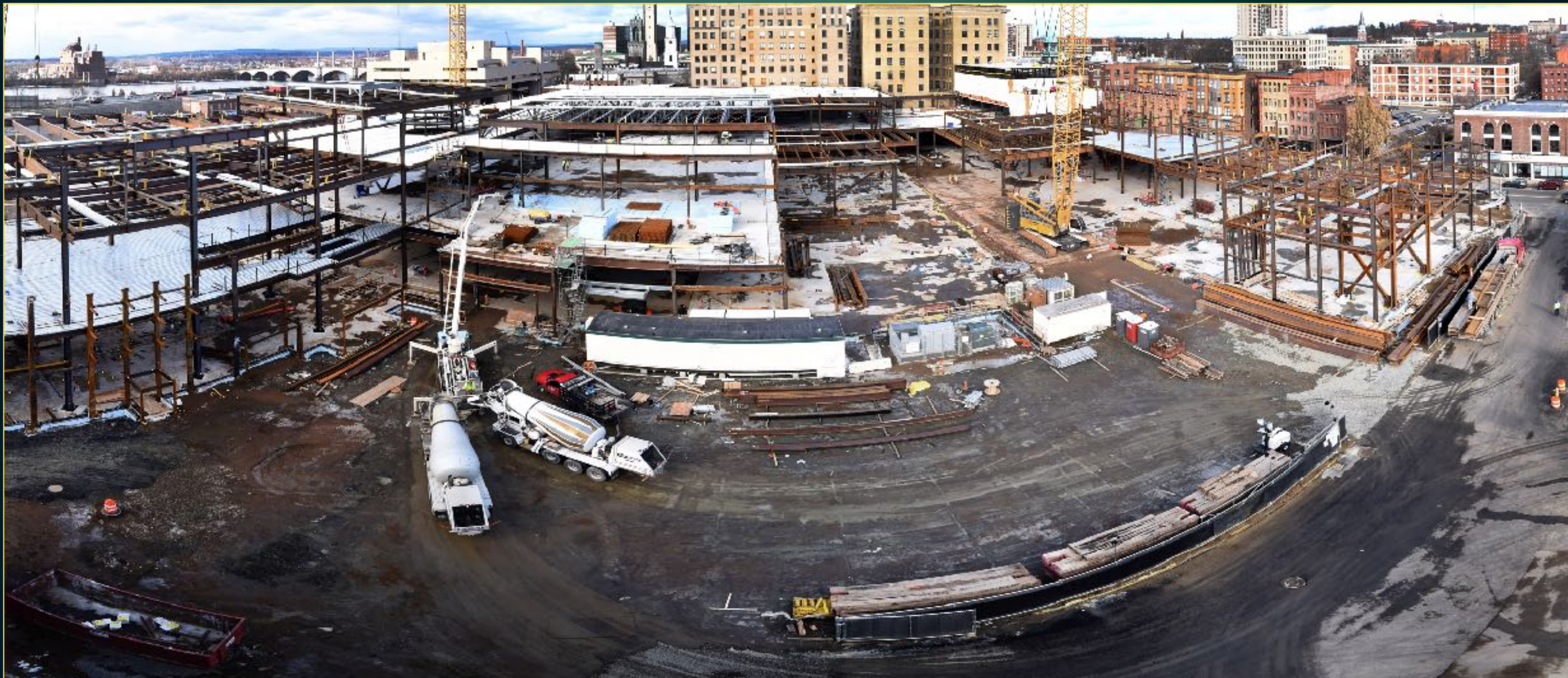
Overall Site Activity from Armory - December 28, 2016
