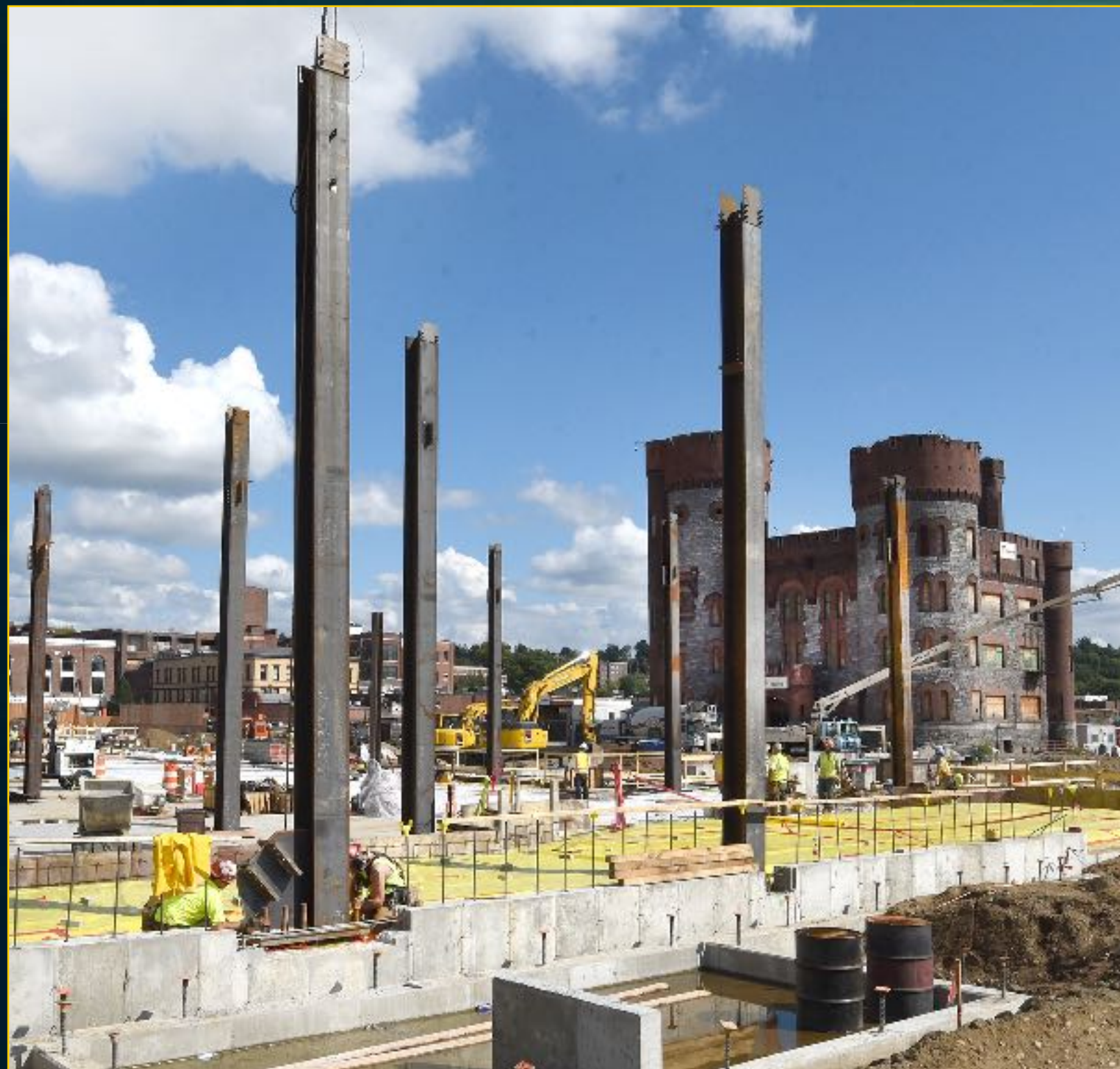
First Steel - October 3, 2016
