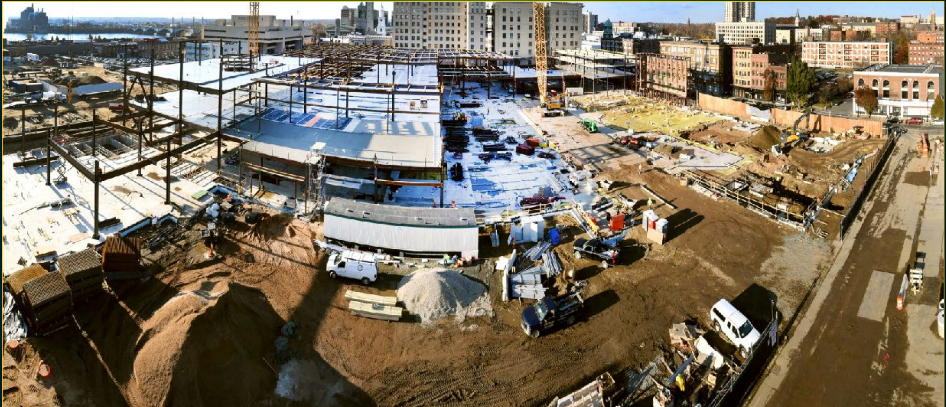
Overall Site Activity from Armory - November 17, 2016
