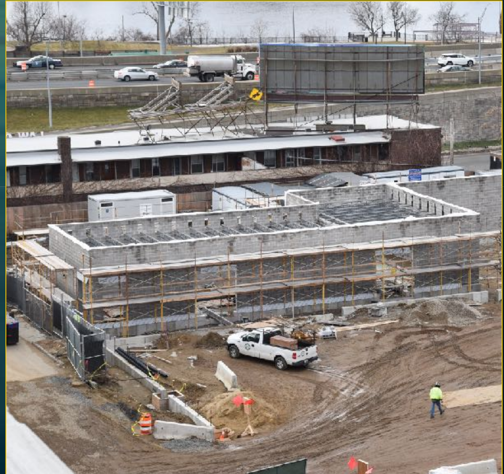
CEF Building - December 28, 2016
