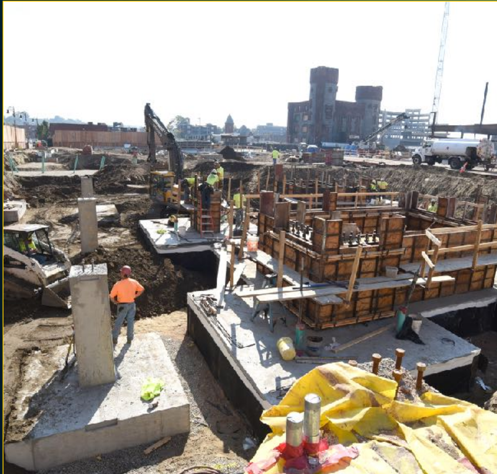
Hotel Construction - October 18, 2016
