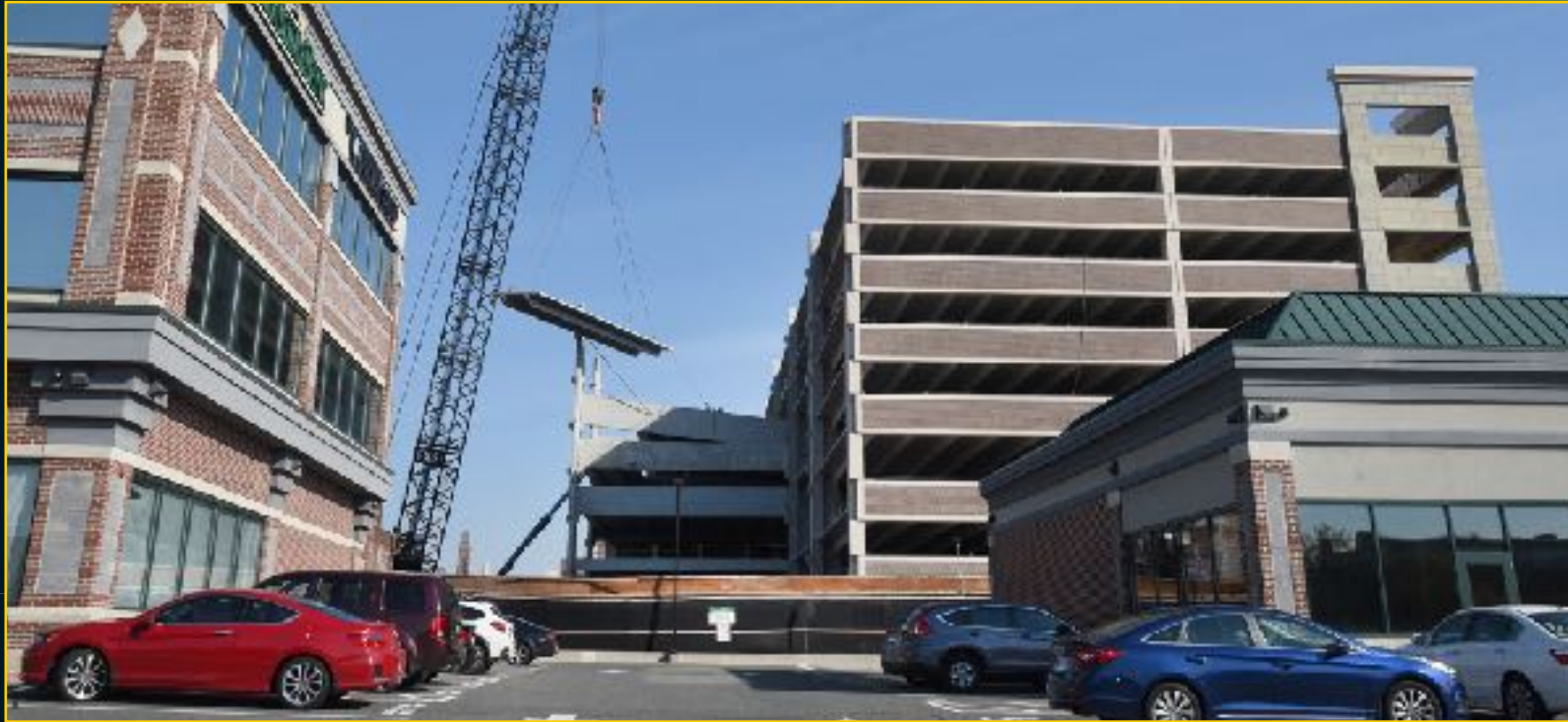
Garage Construction - November 2, 2016
