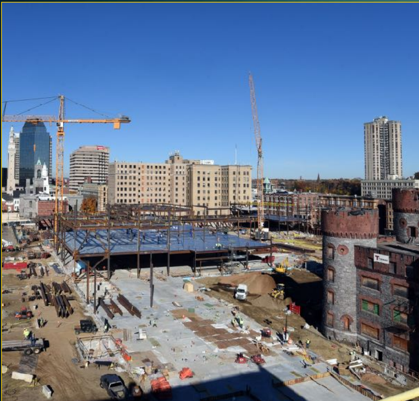
Podium Steel Erection - November 8, 2016
