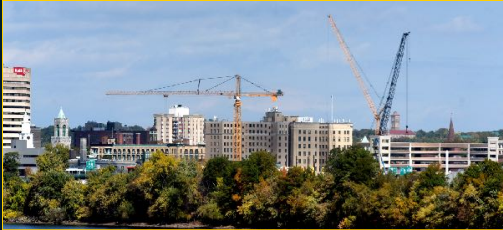
Crane Erection - October 17, 2016
