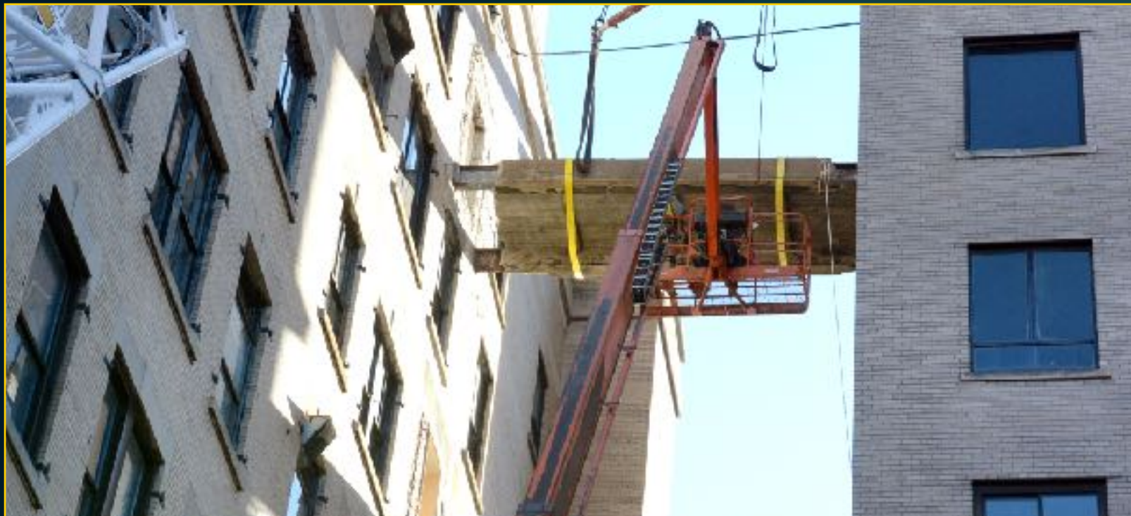
Pedestrian Bridge Demolition - November 19, 2016
