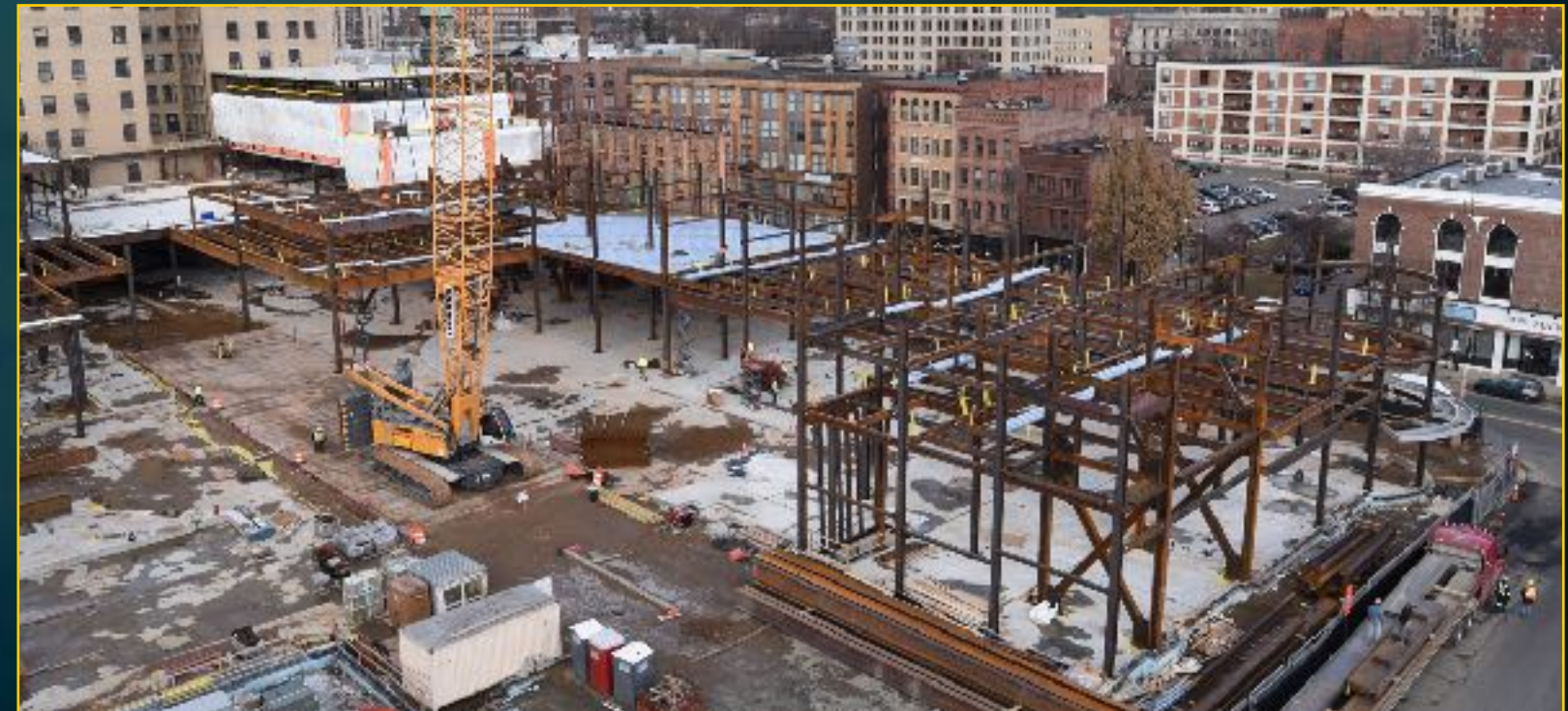
Hotel Construction - December 28, 2016
