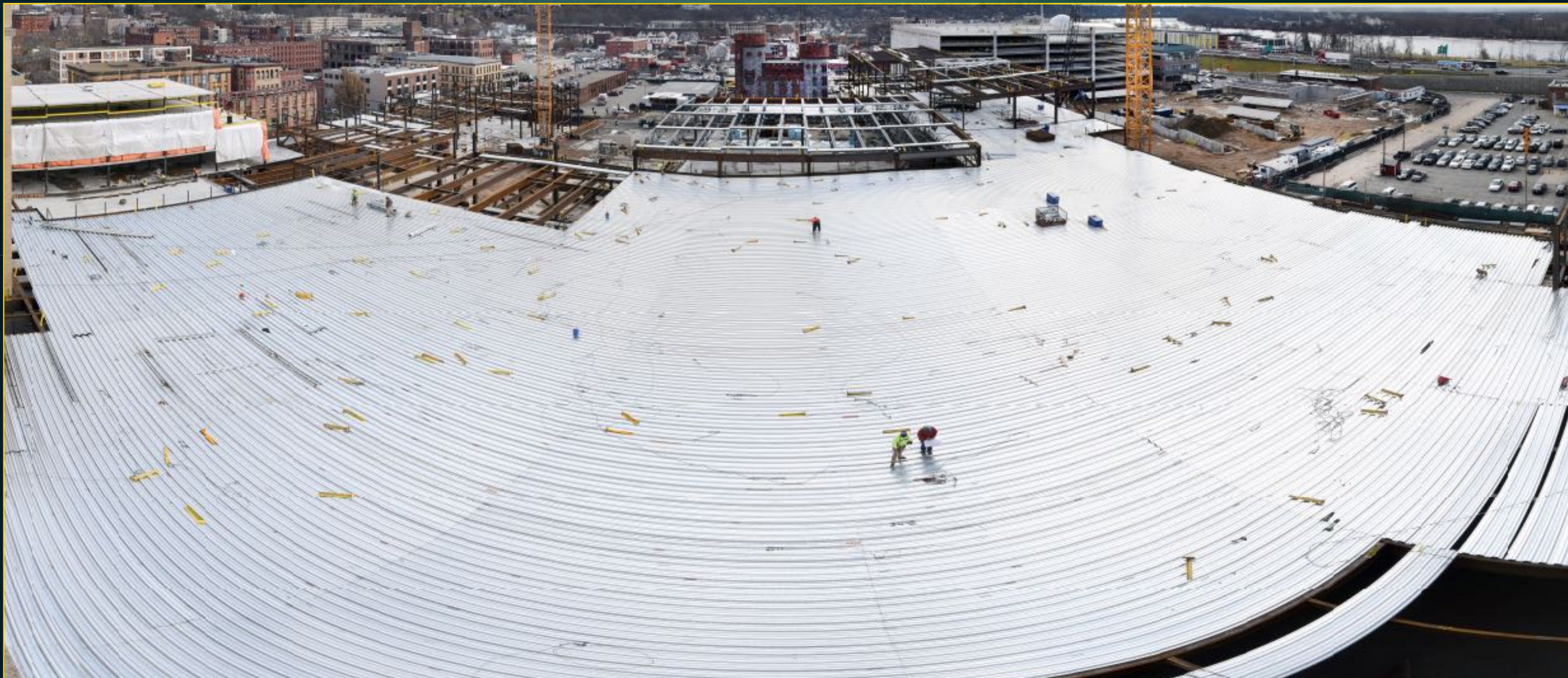
Overall Site Activity from 95 State - December 28, 2016
