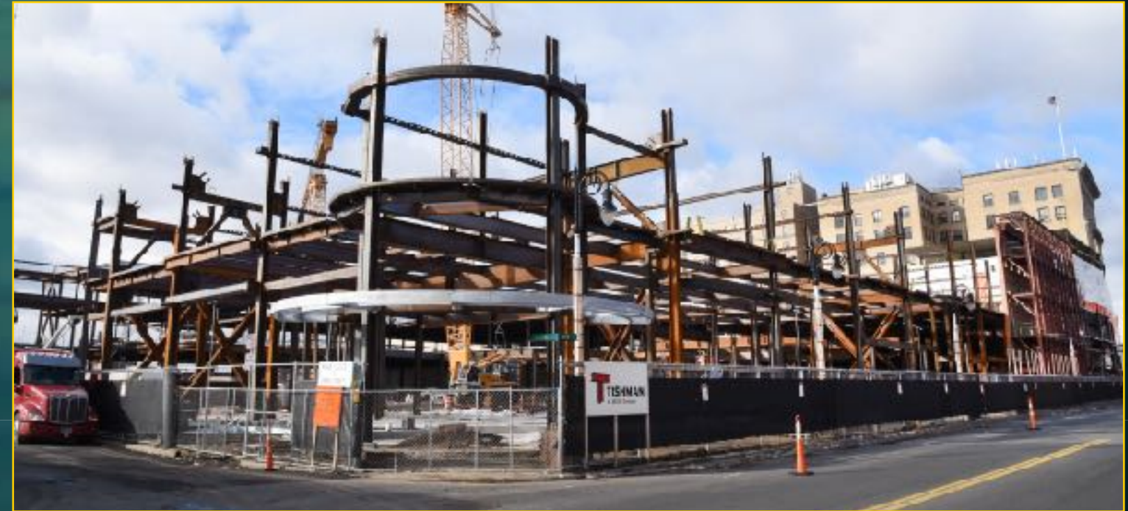
Hotel Construction - December 28, 2016
