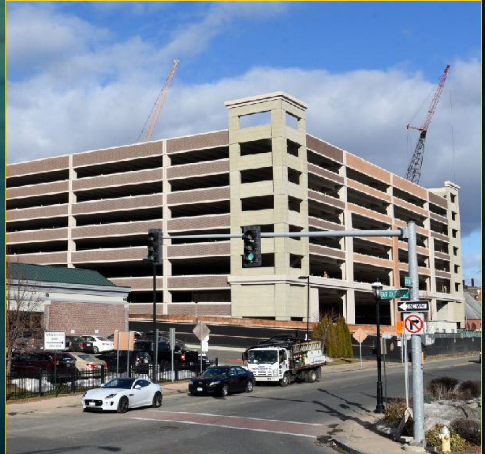
Garage Construction - December 28, 2016
