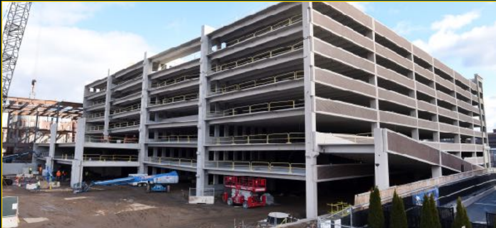
Garage Construction - December 28, 2016
