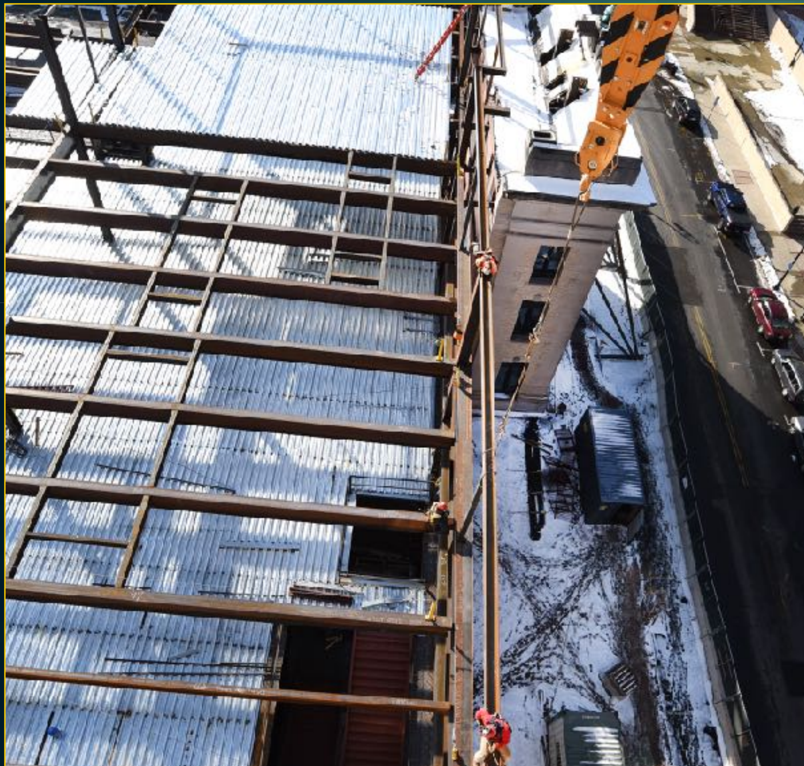
Podium Steel Erection - December 13, 2016
