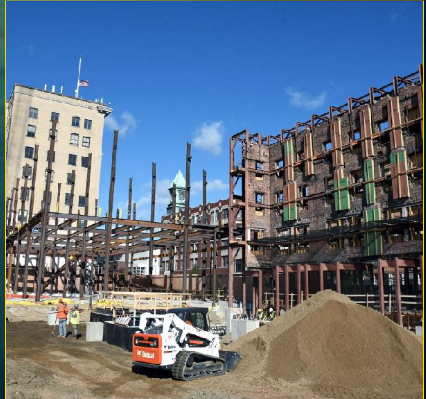
Hotel Construction - October 25, 2016
