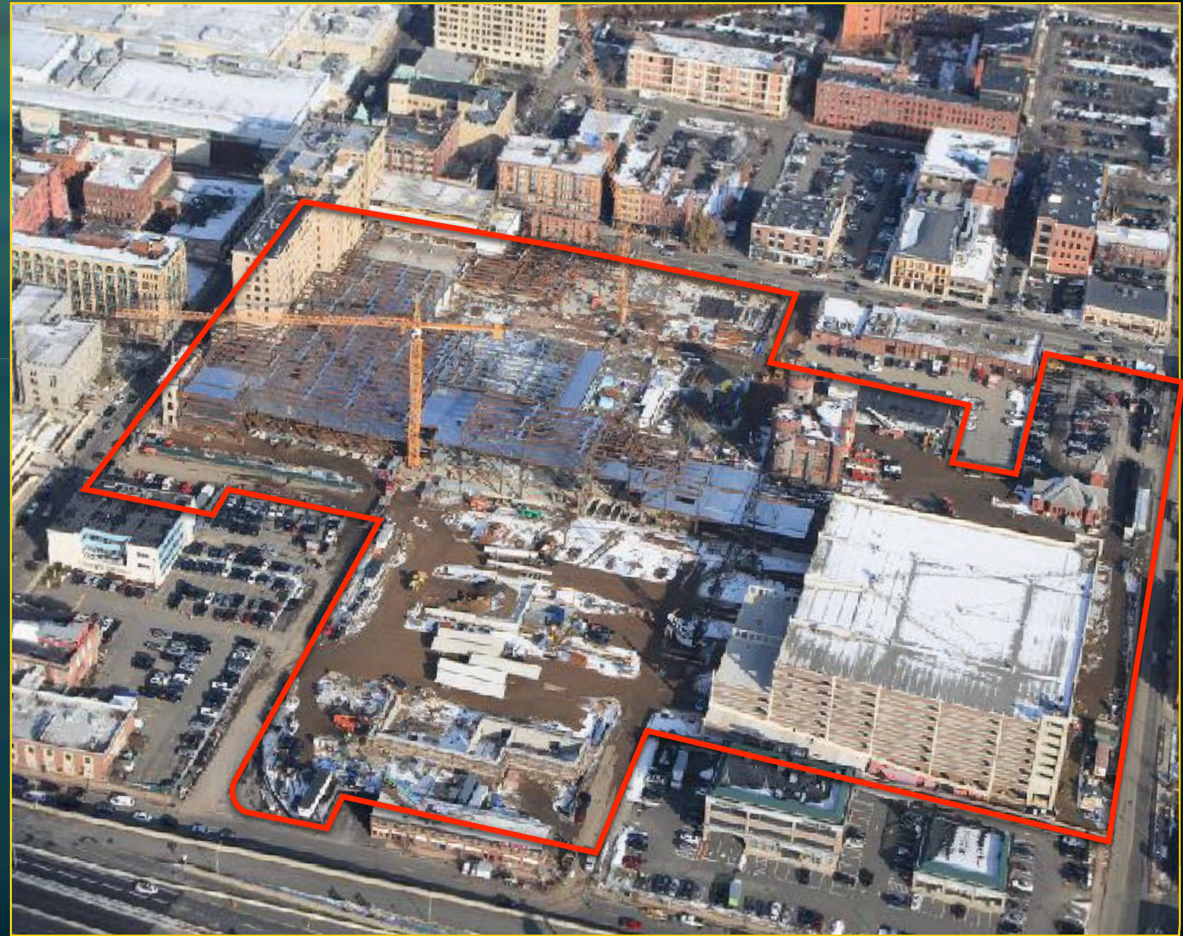
Aerial View - December 14, 2016
