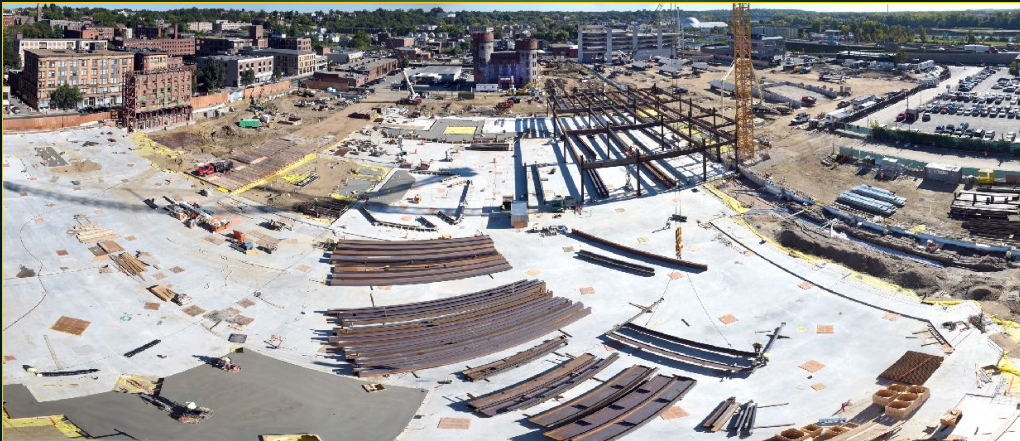
Overall Site Activity from 95 State - October 6, 2016
