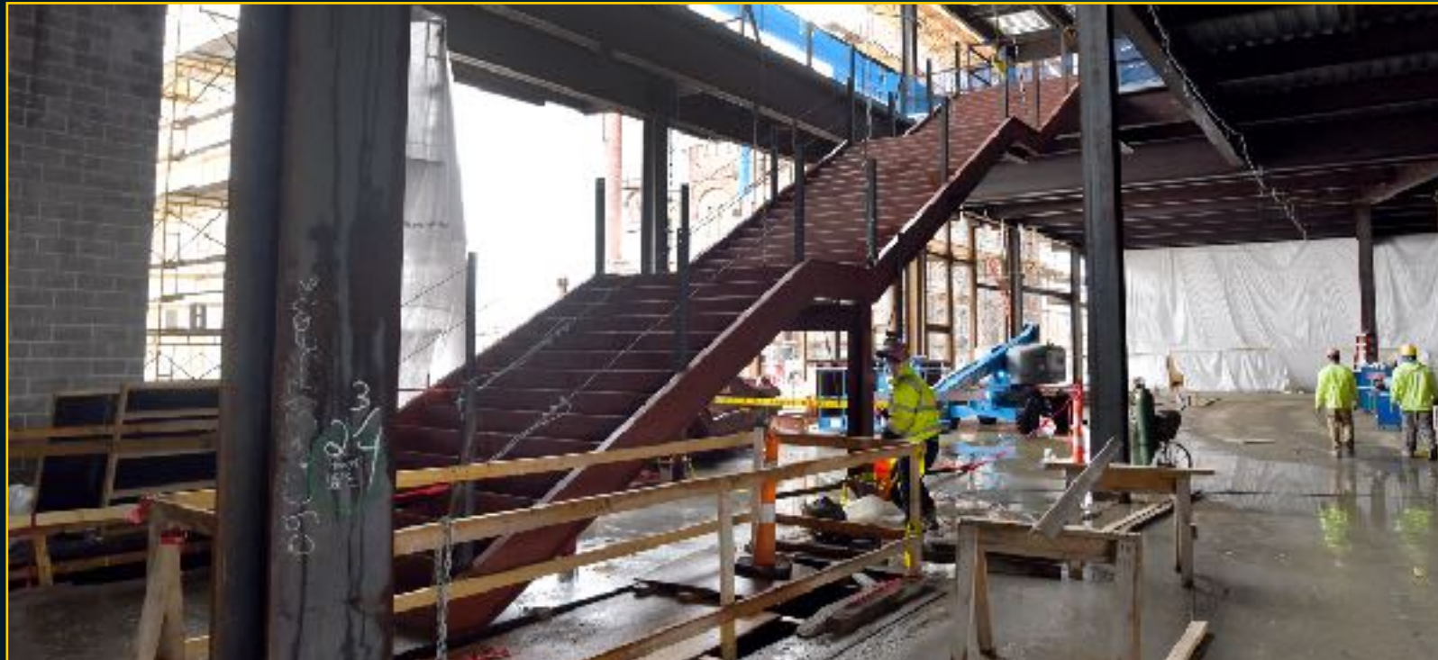
Podium Construction - March 8, 2017
