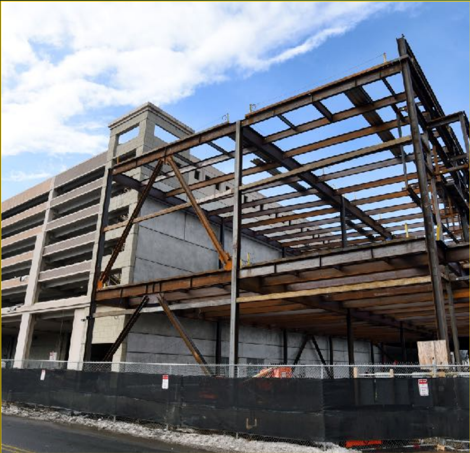
Entertainment Steel Erection - January 26, 2017
