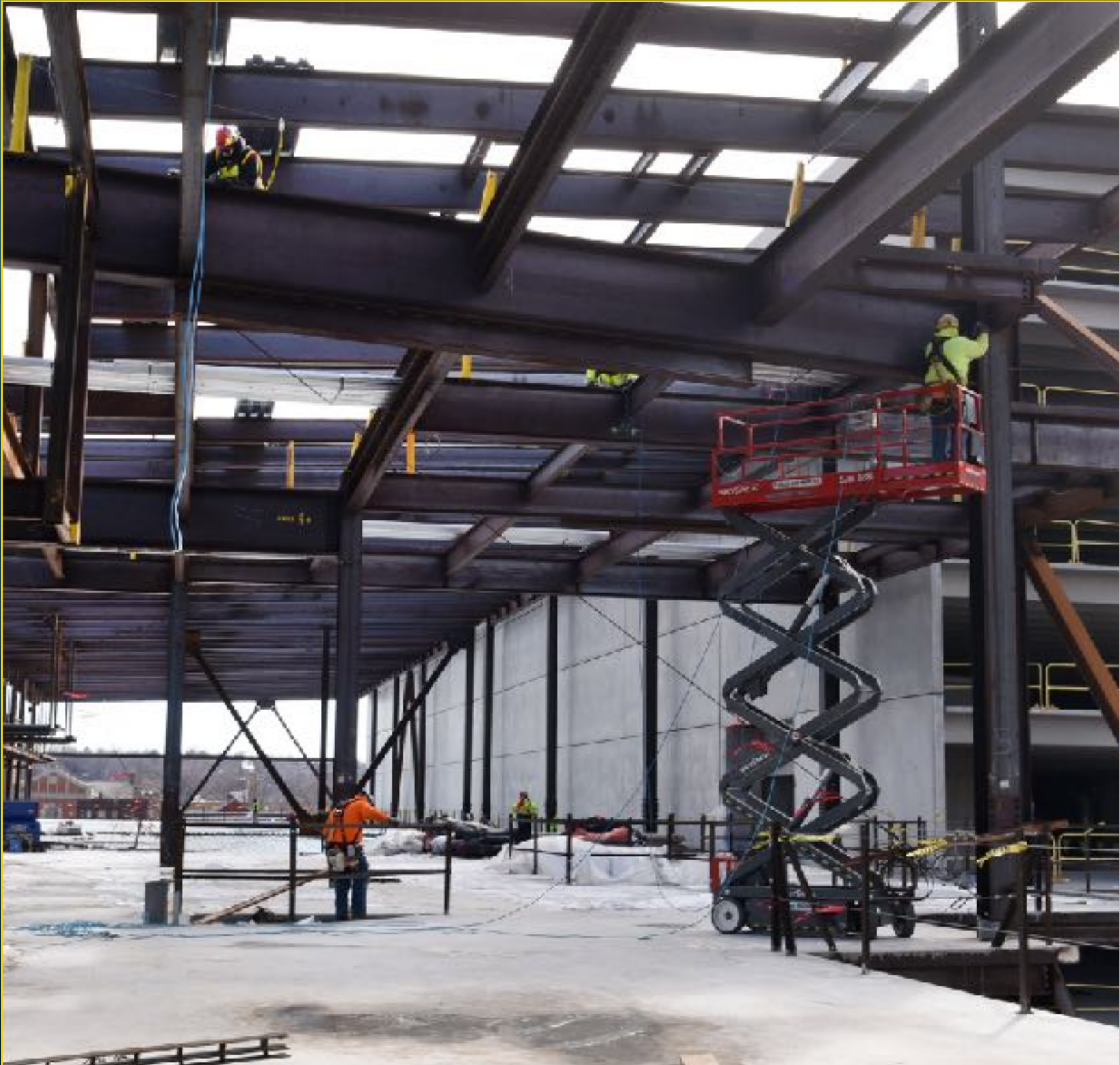
Entertainment Steel Erection - February 6, 2017
