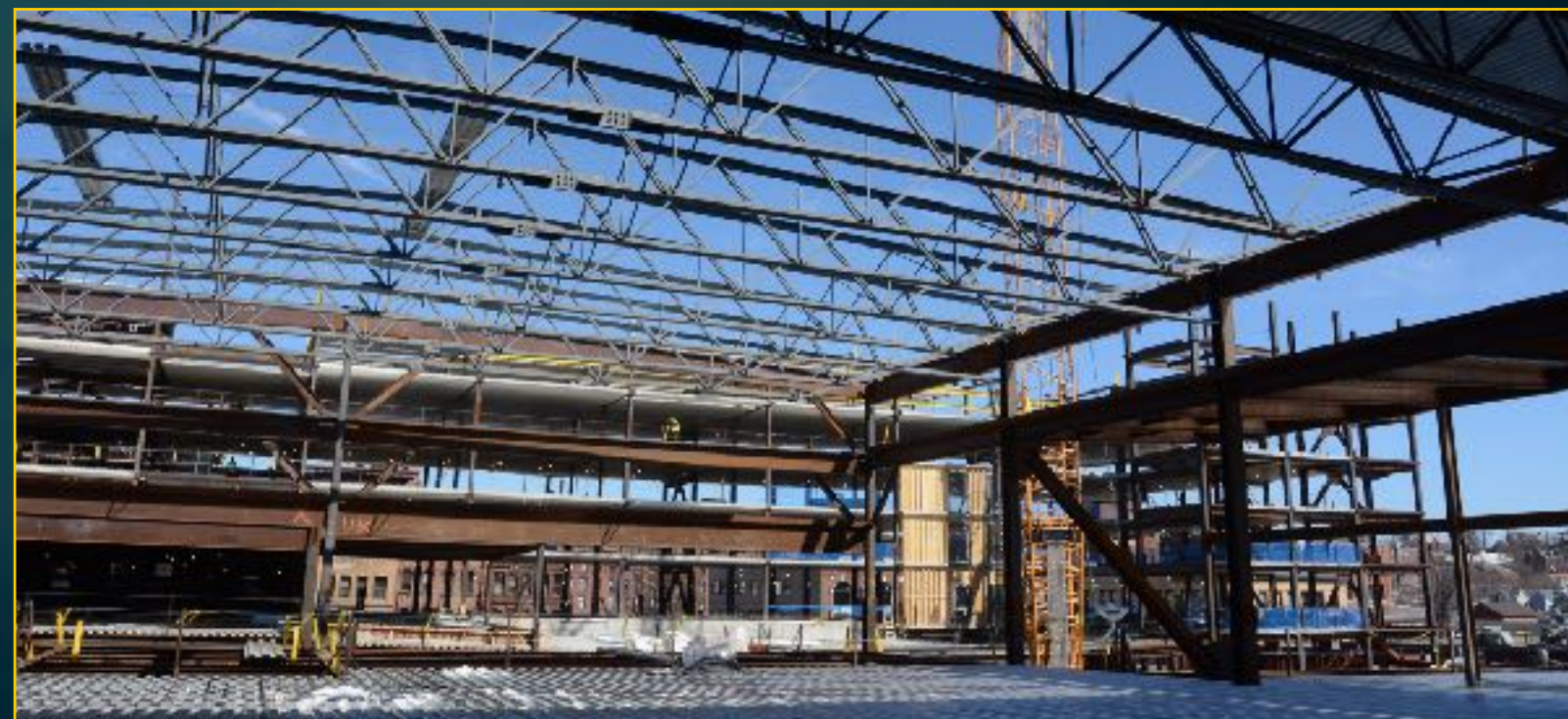
Podium Steel - March 28, 2017
