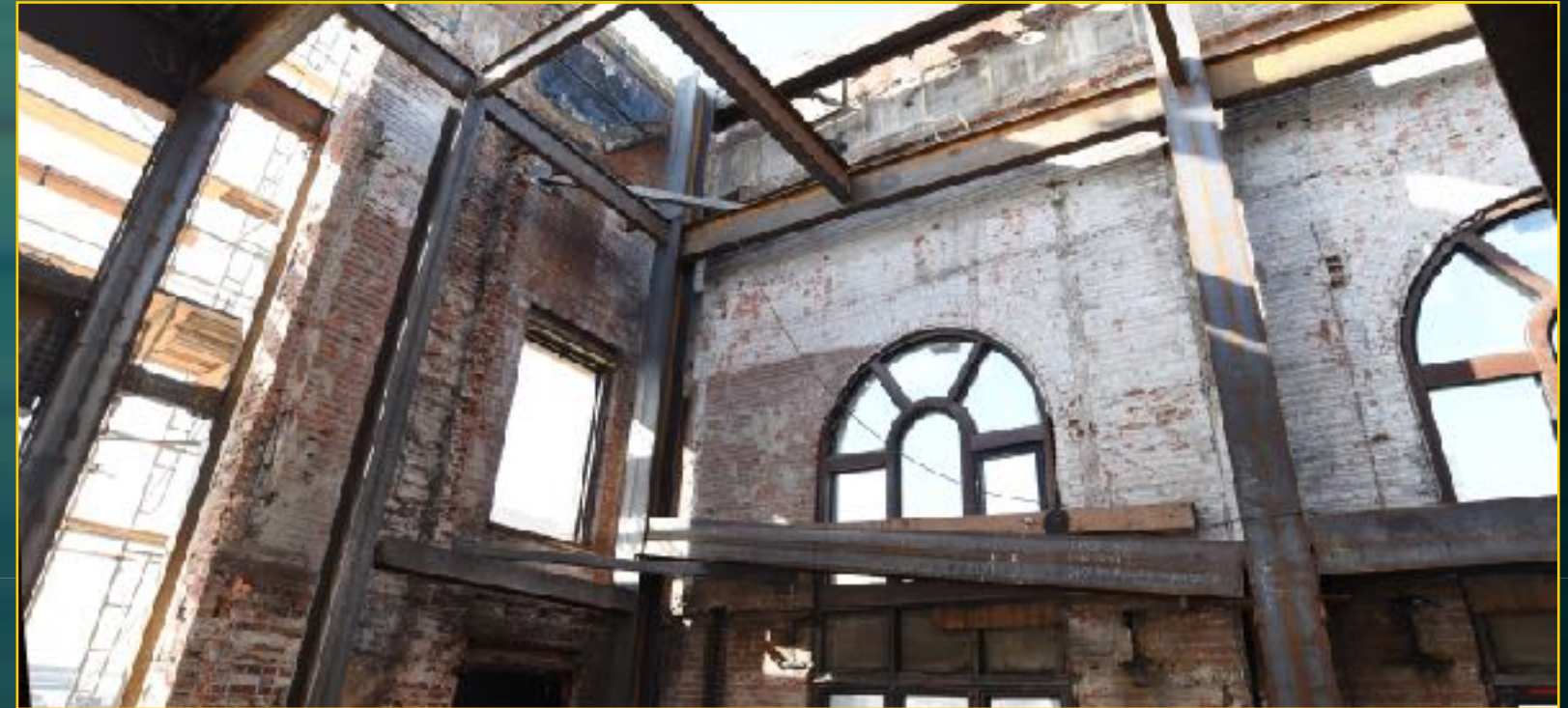
Hotel Construction - February 8, 2017
