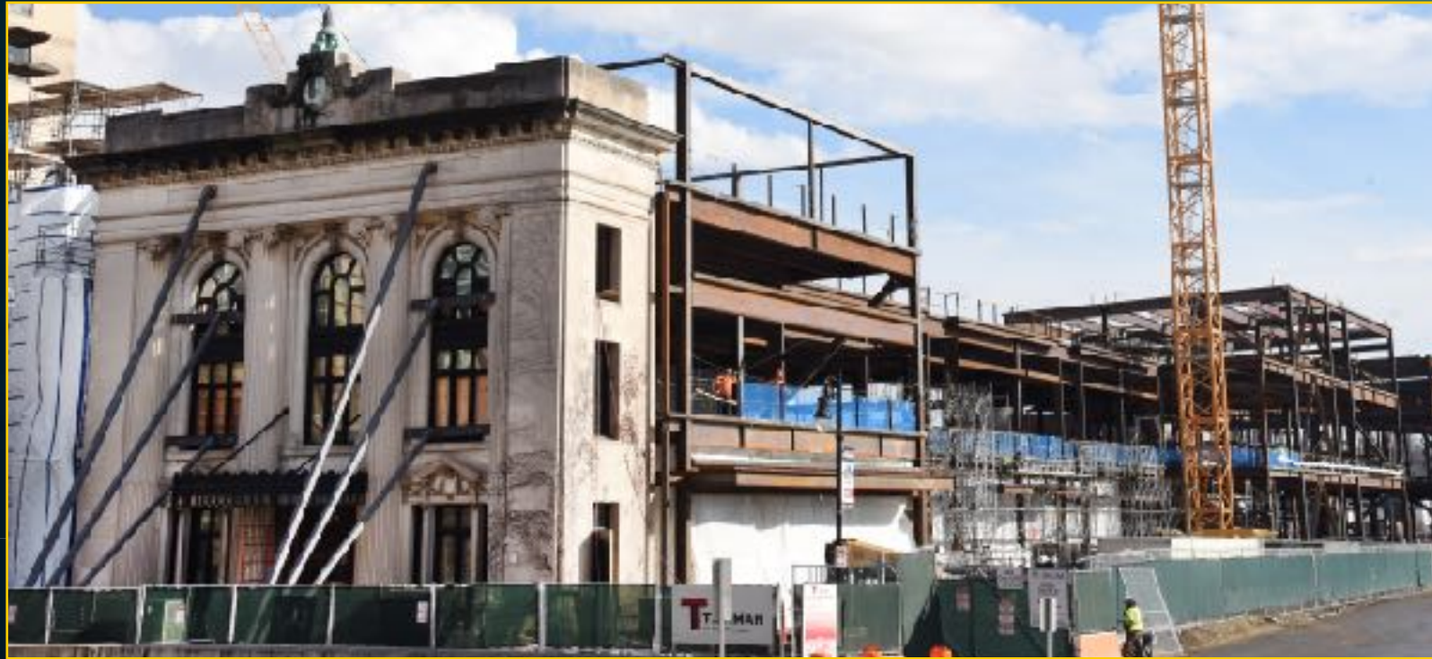
73 State Construction - January 26, 2017
