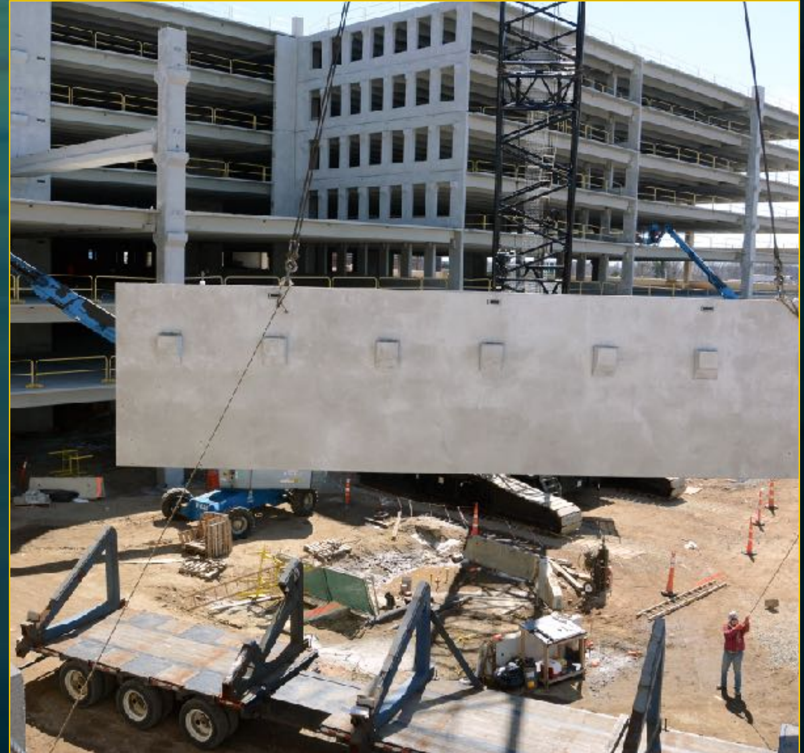
Garage Construction - March 28, 2017
