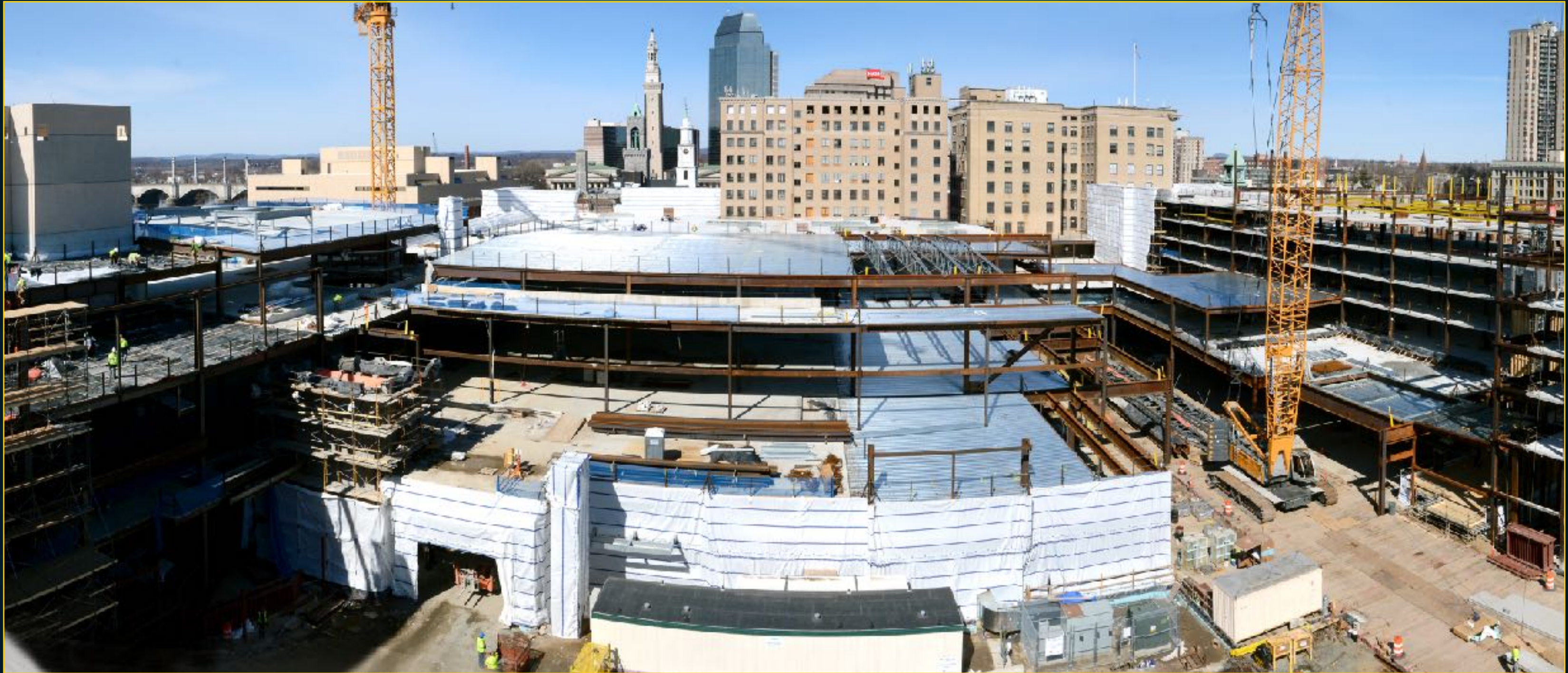
Overall Site Activity from Armory - March 13, 2017
