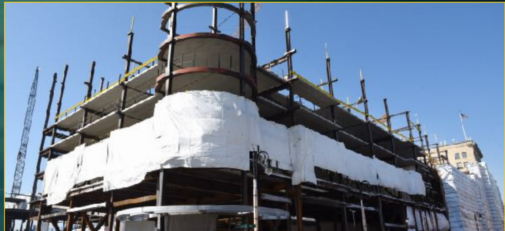
Hotel Entrance - February 24, 2017
