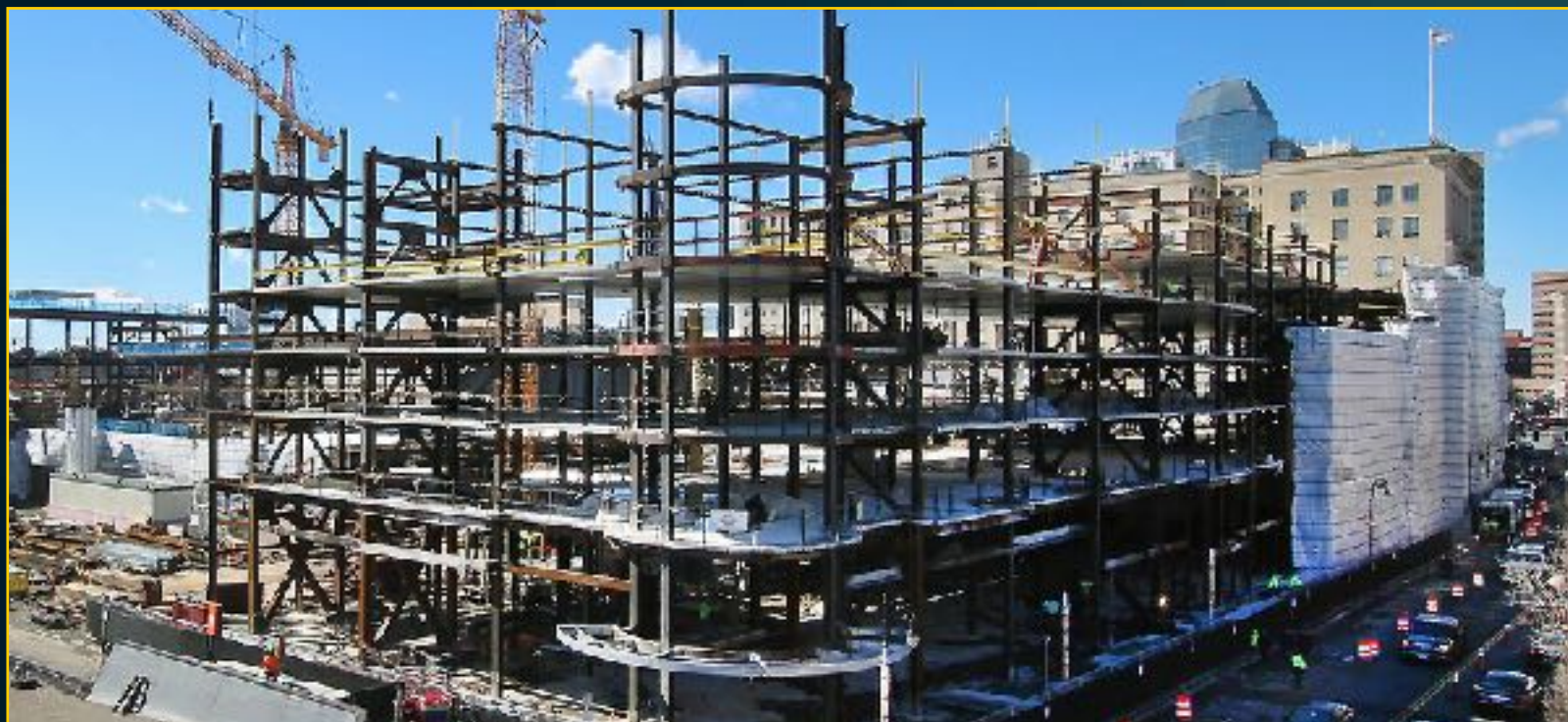
Hotel Entrance - March 8, 2017
