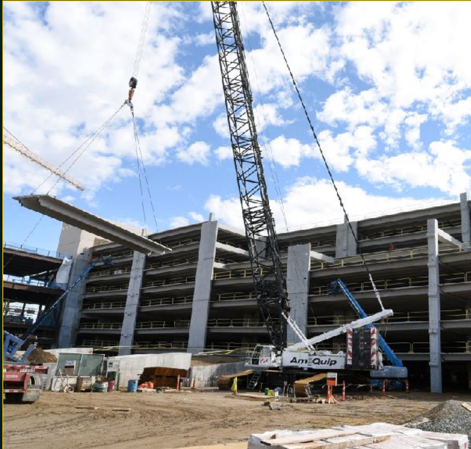
Garage Construction - March 8, 2017
