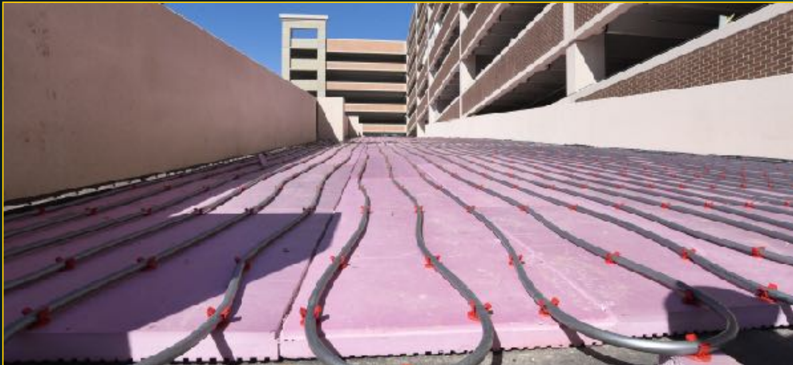
Garage Construction - March 3, 2017
