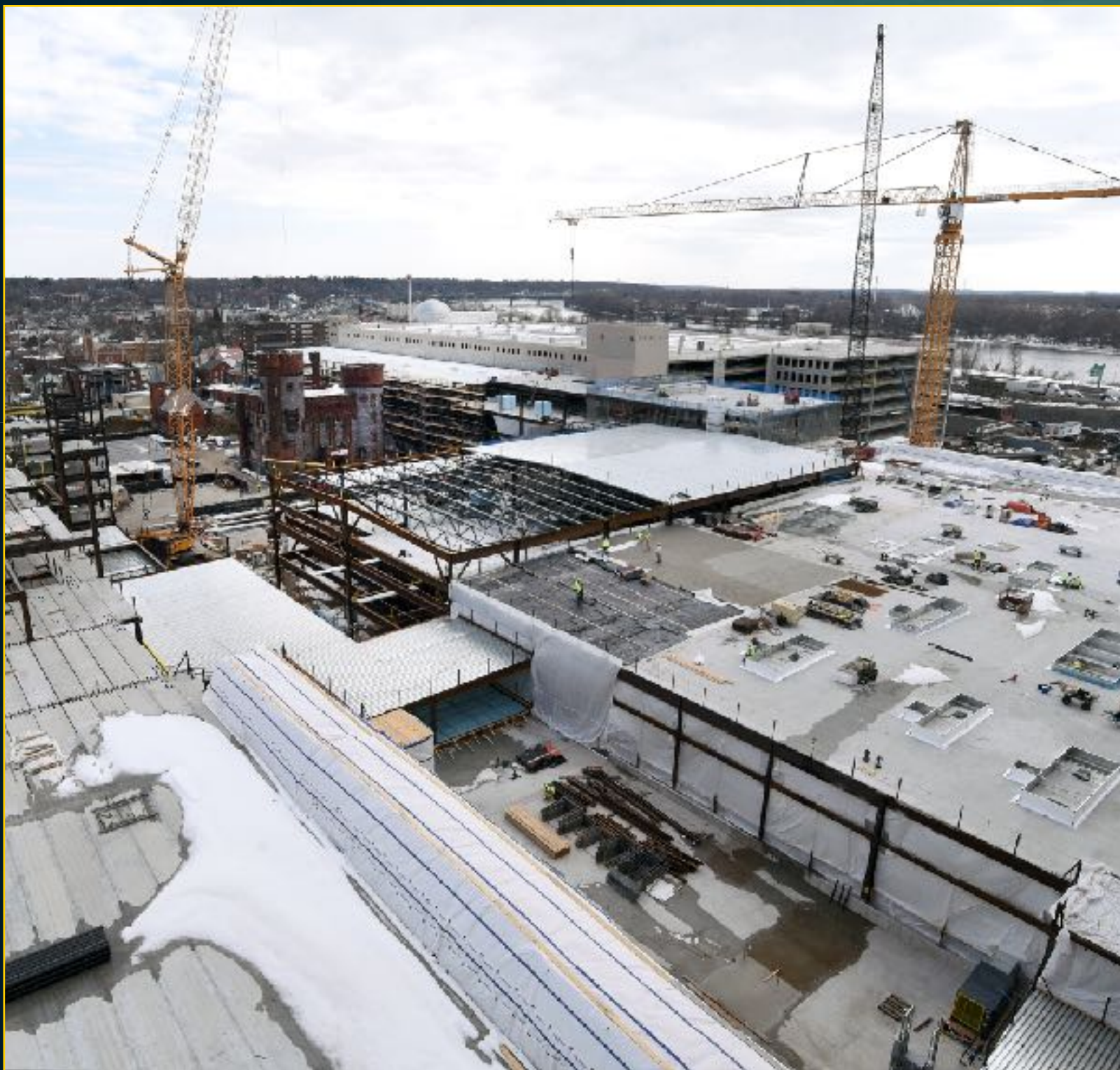
Podium Enclosure - March 21, 2017
