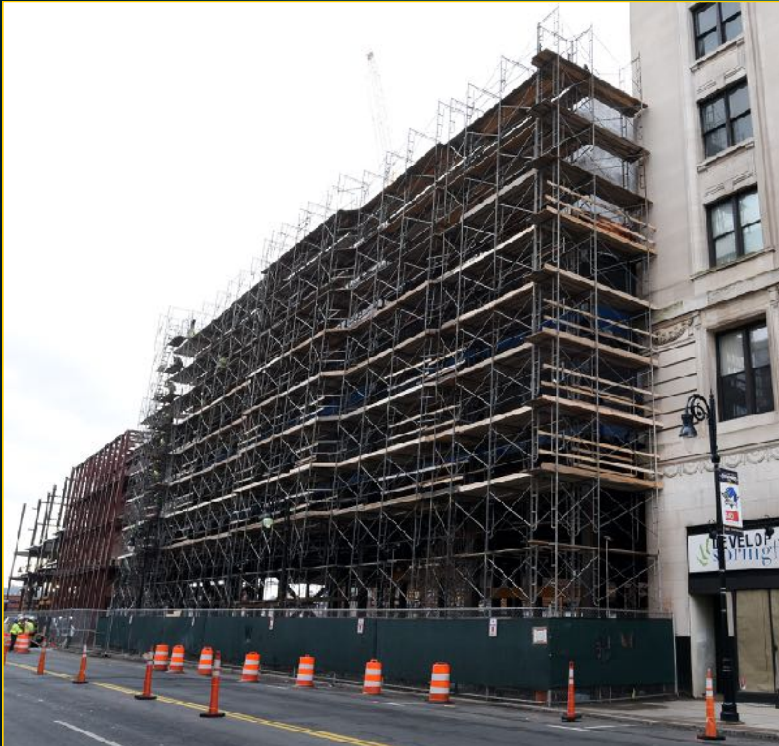
Main Street Scaffolding - January 19, 2017
