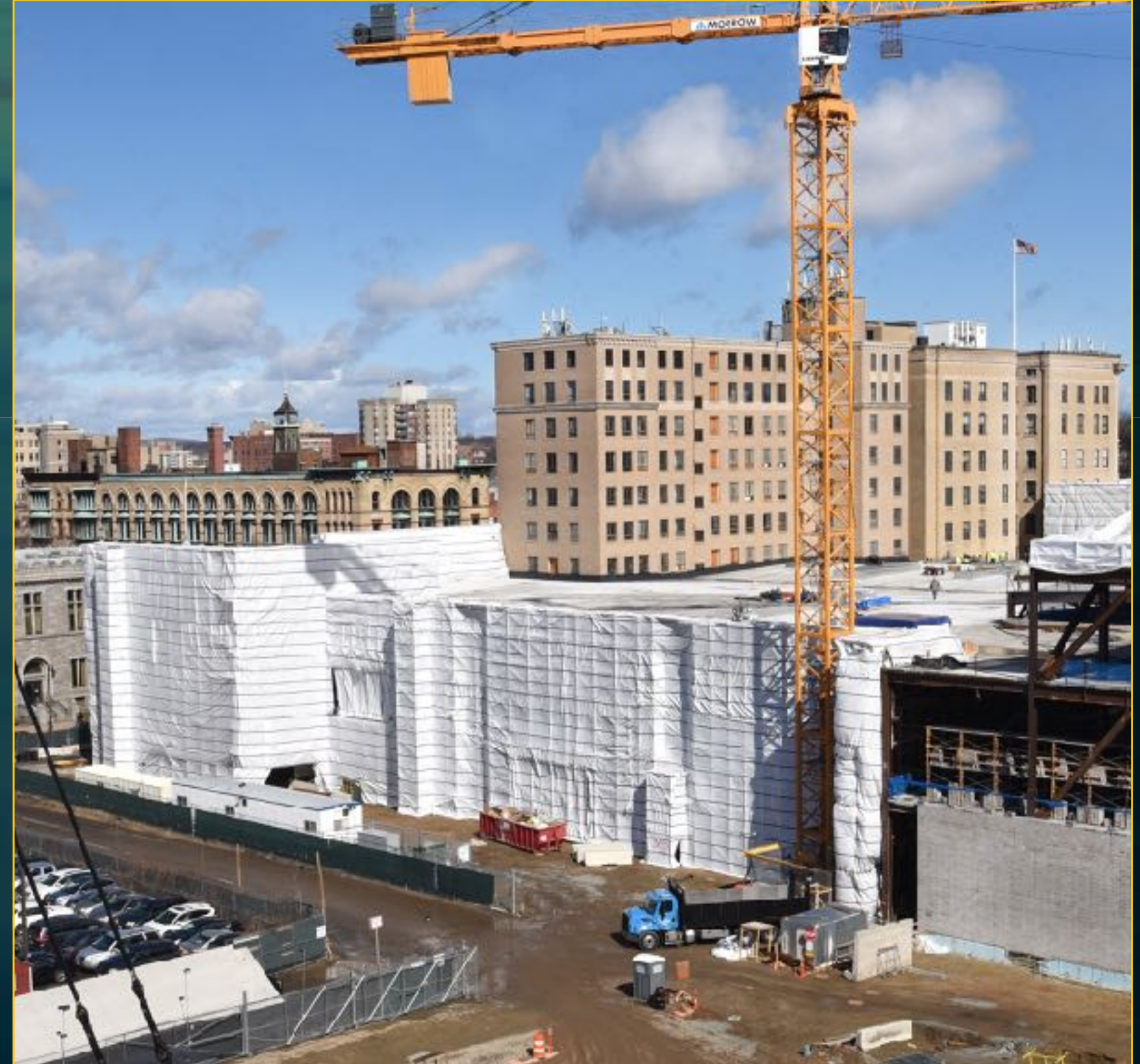
Podium Enclosure - March 8, 2017
