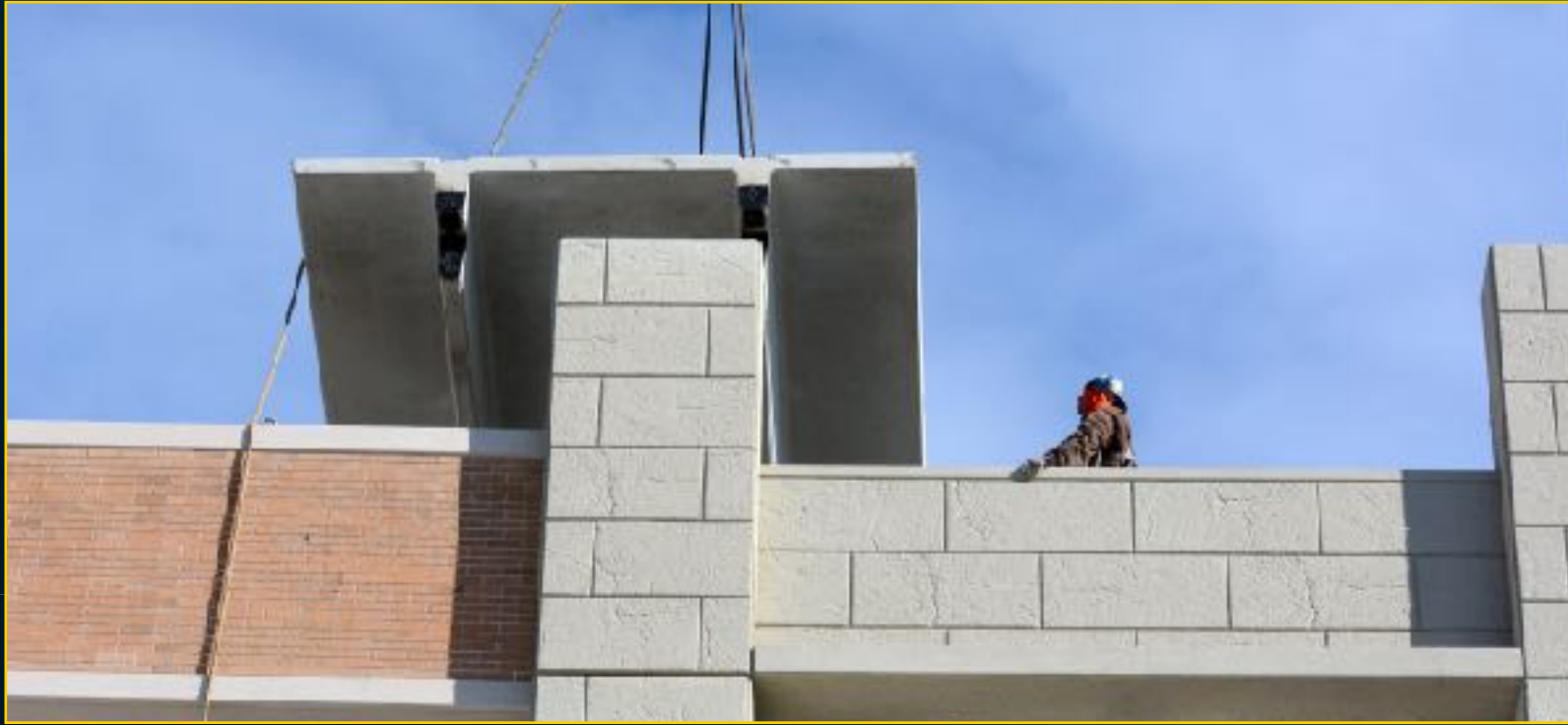
Garage Construction - February 6, 2017
