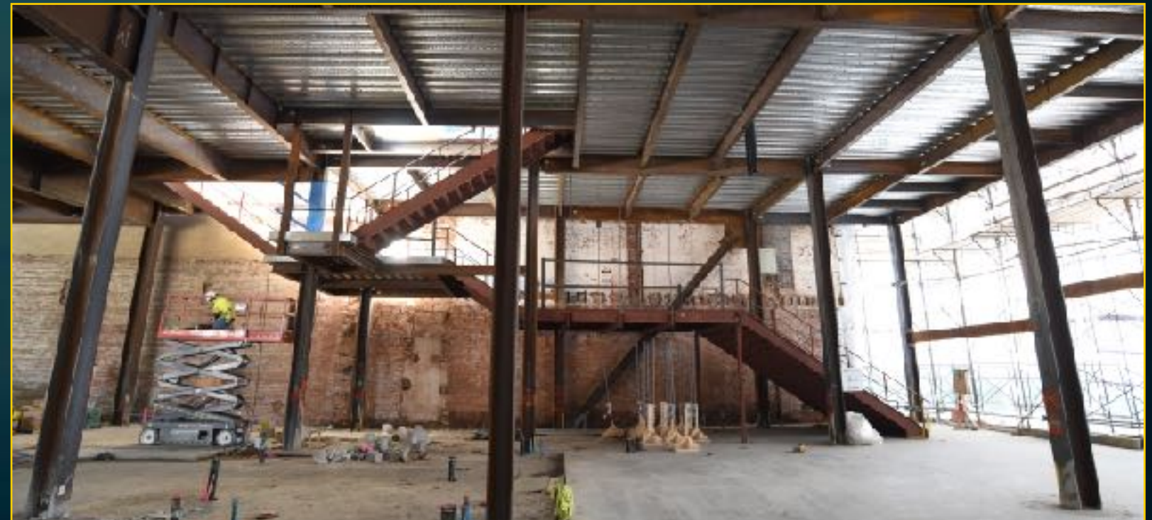
Hotel Construction - February 7, 2017
