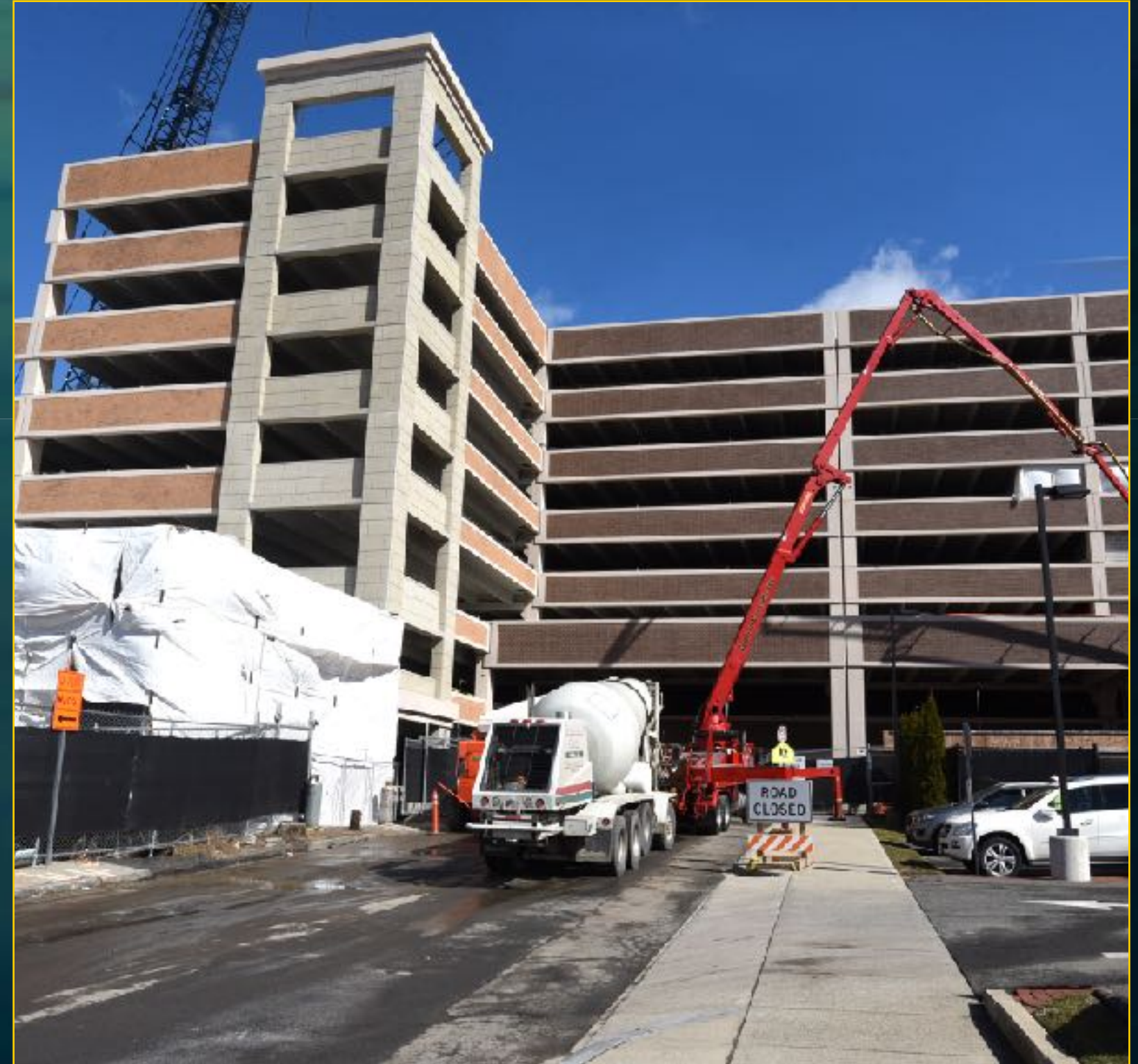
Garage Construction - March 8, 2017
