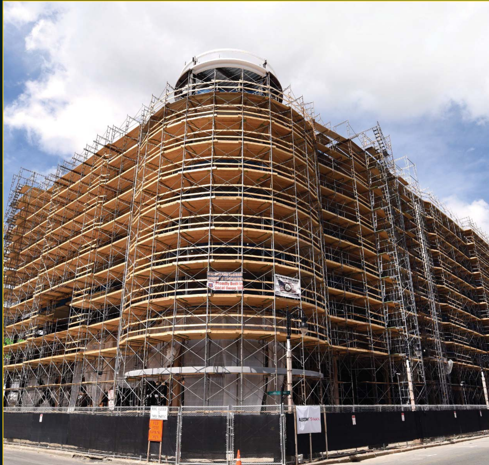
Hotel Entrance - May 11, 2017
