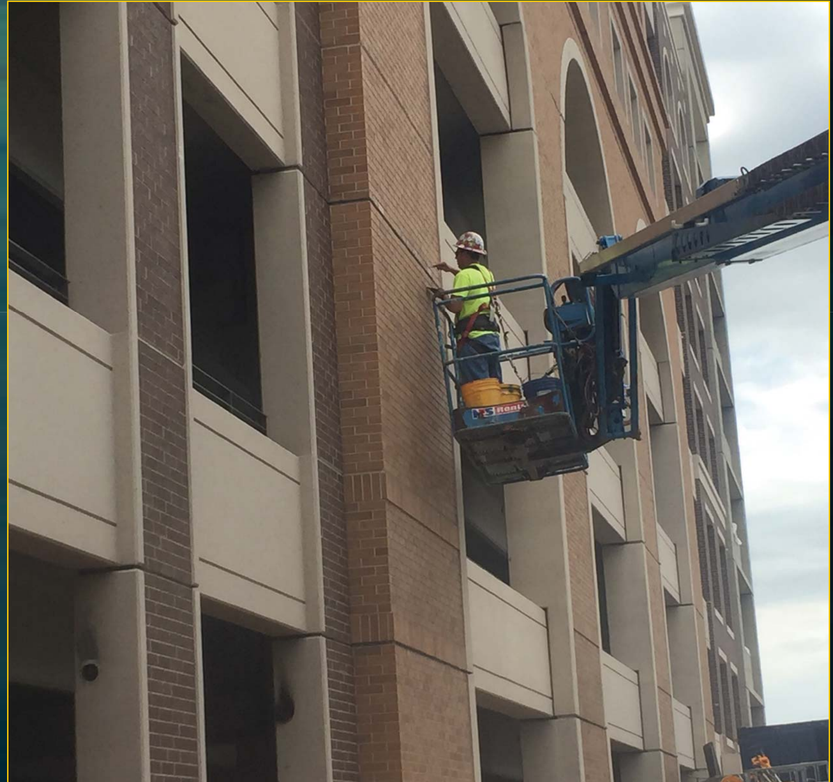
Parking Garage Facade - June 15, 2017
