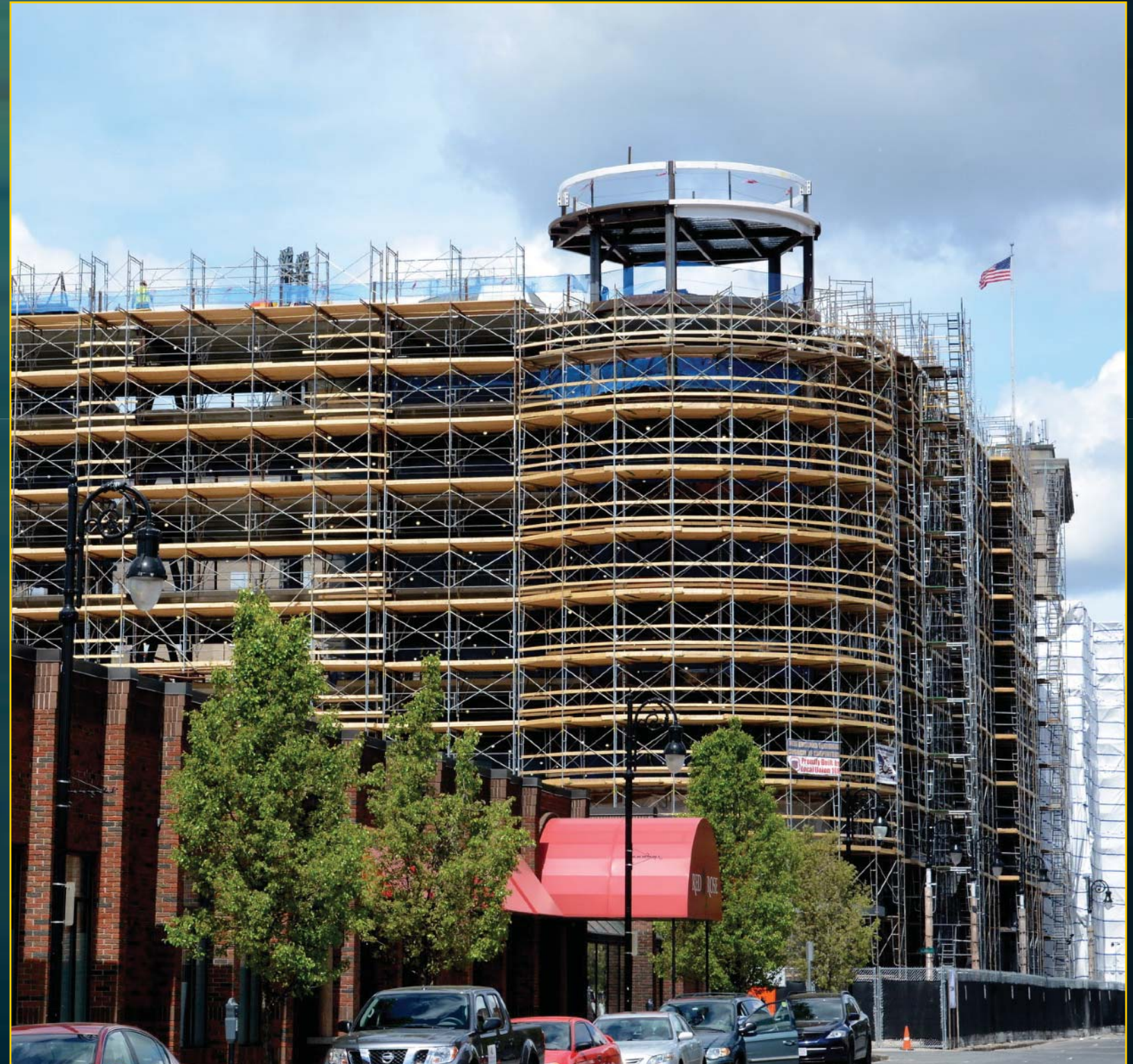
Hotel Entrance - May 11, 2017
