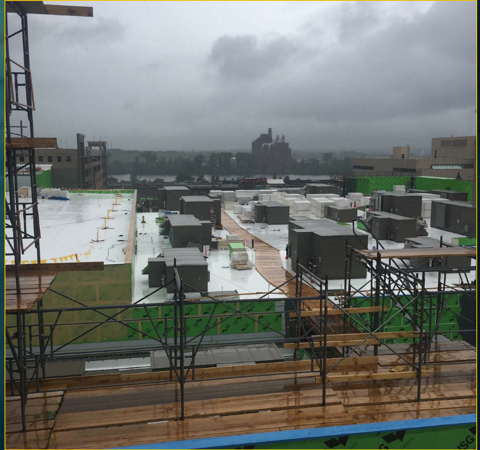
Podium Air Handlers Lifted in Place - June 6, 2017
