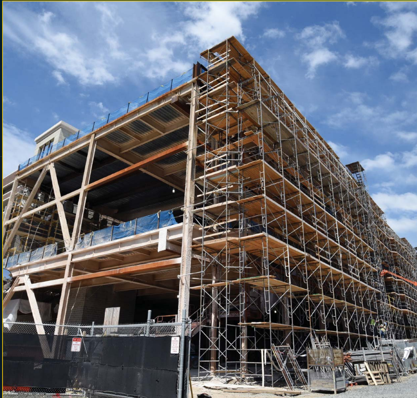
Entertainment Block Construction - June 15, 2017
