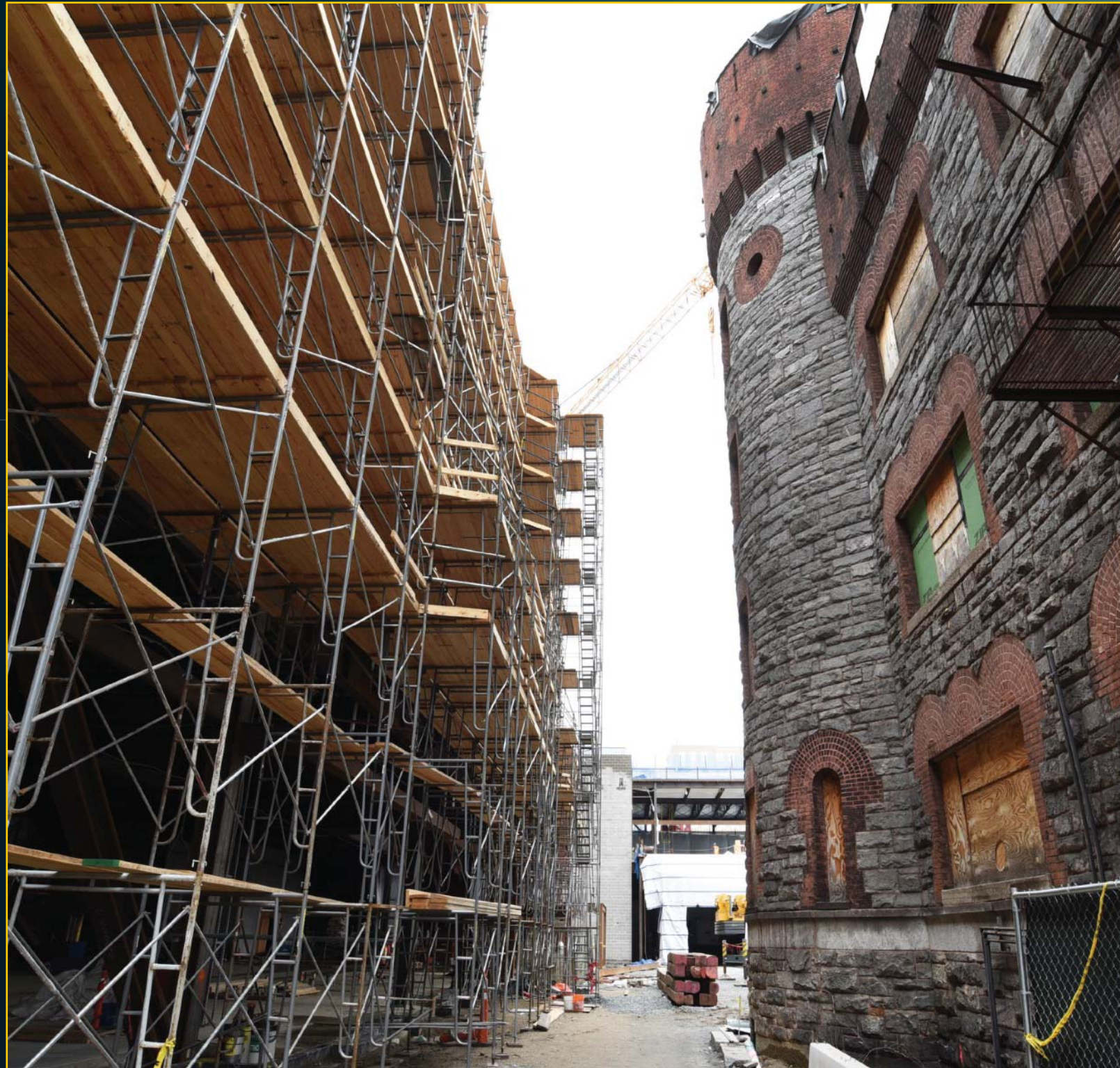
Entertainment Block Construction - April 5, 2017
