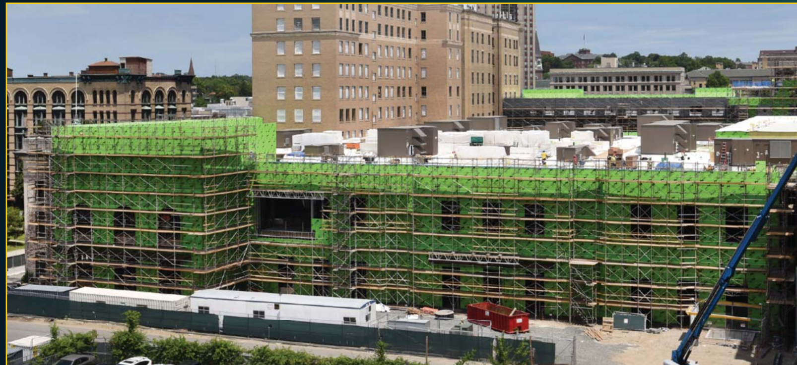
Podium Construction - June 15, 2017
