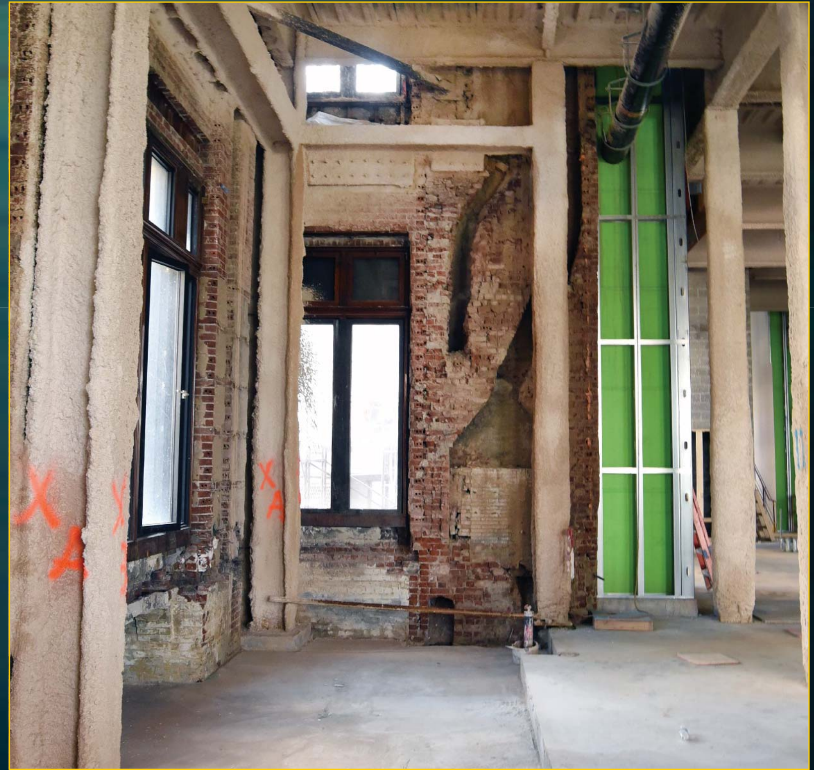
73 State Chimney - June 26, 2017
