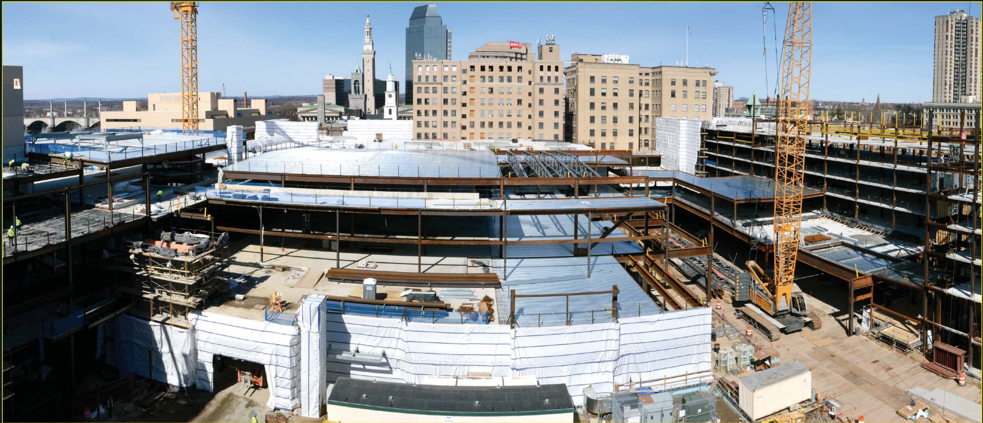
Overall Site Activity from Armory - March 13, 2017
