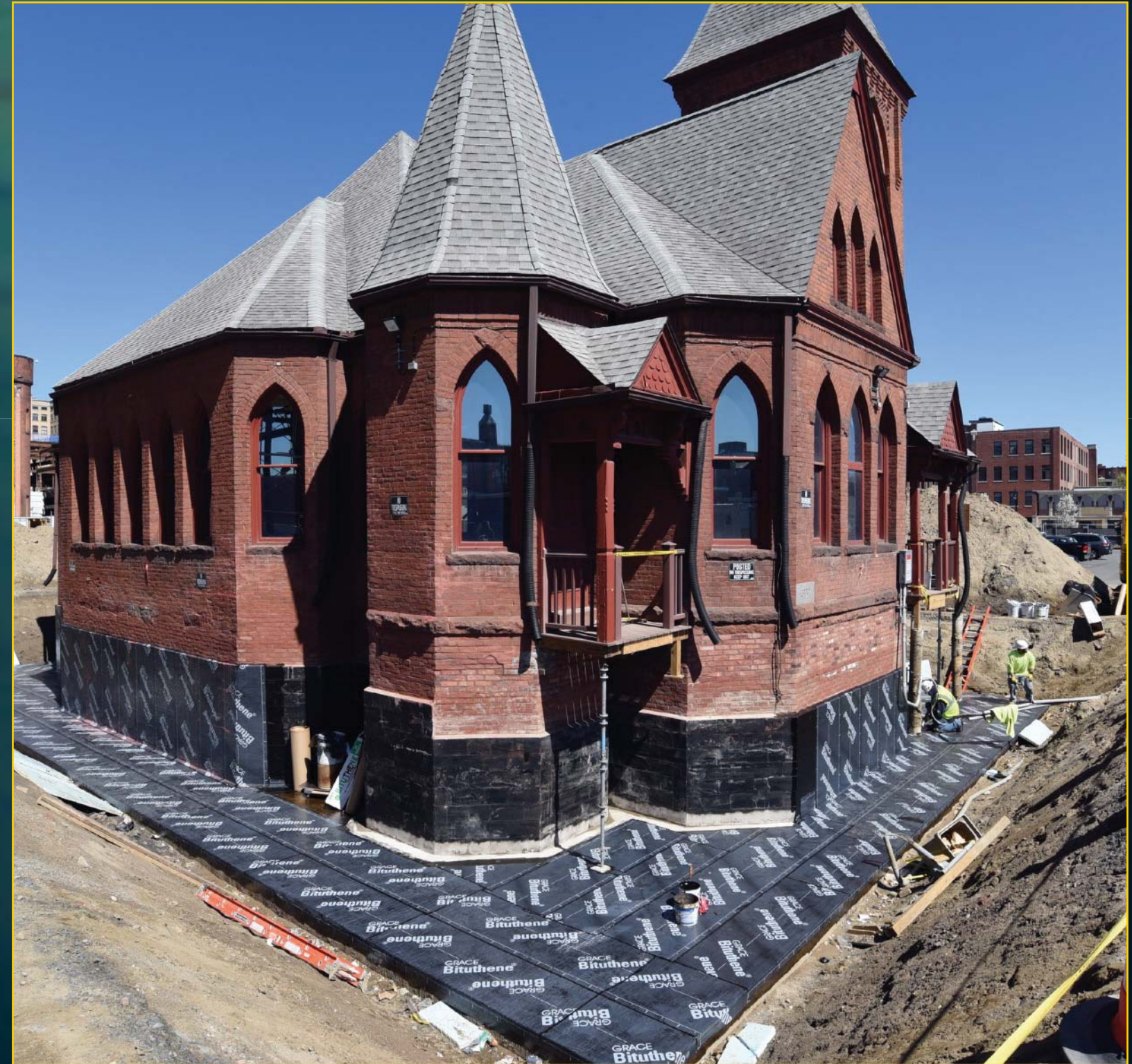
Church Construction - April 18, 2017
