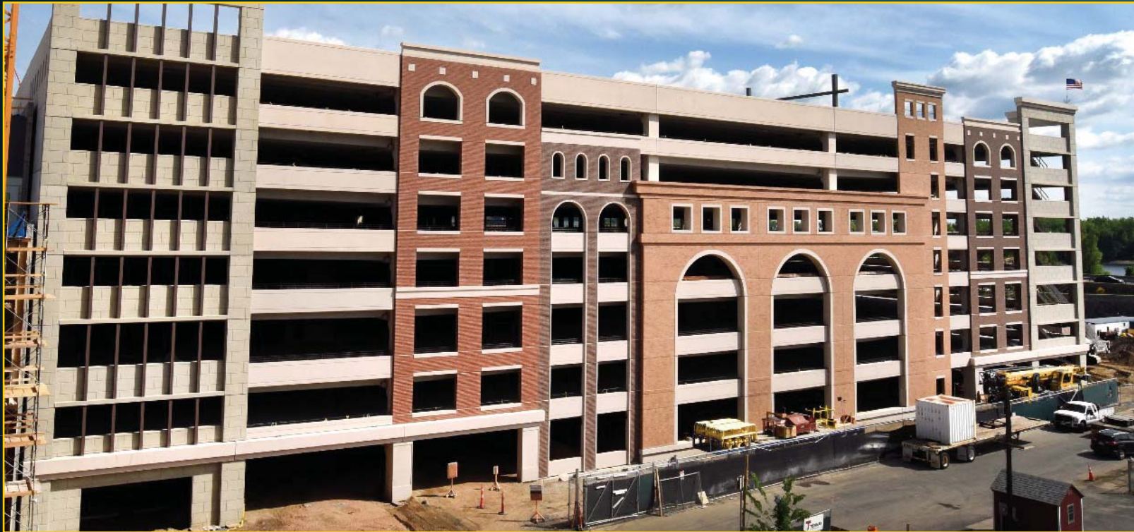
Parking Garage Facade - May 24, 2017
