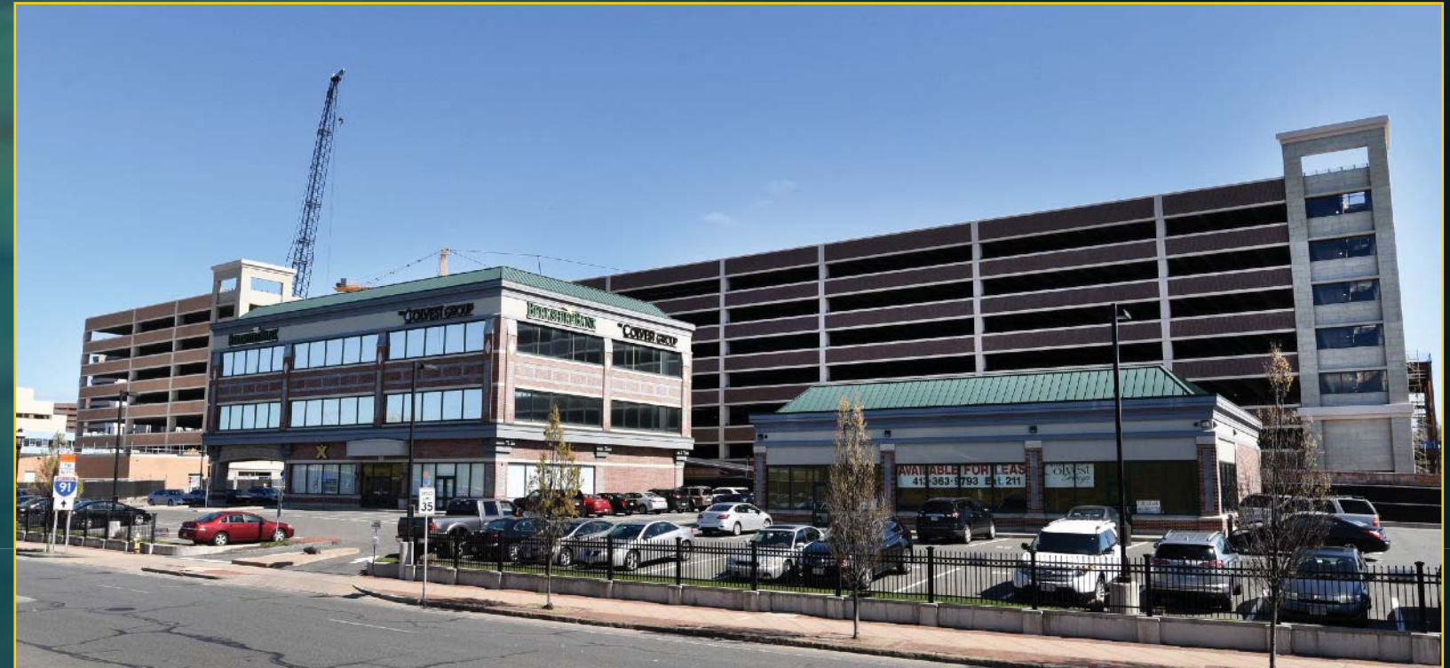
Garage Construction - April 18, 2017
