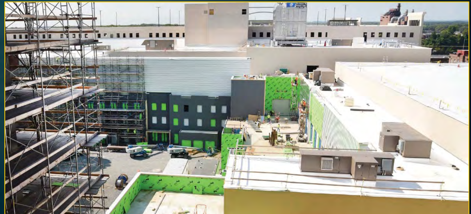
Podium Construction - September 13, 2017
