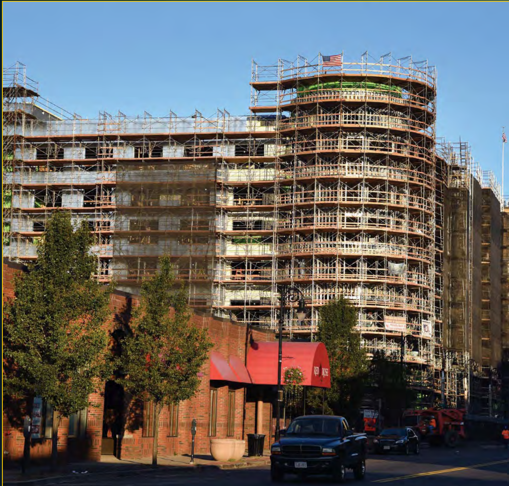
Hotel Construction - September 28, 2017
