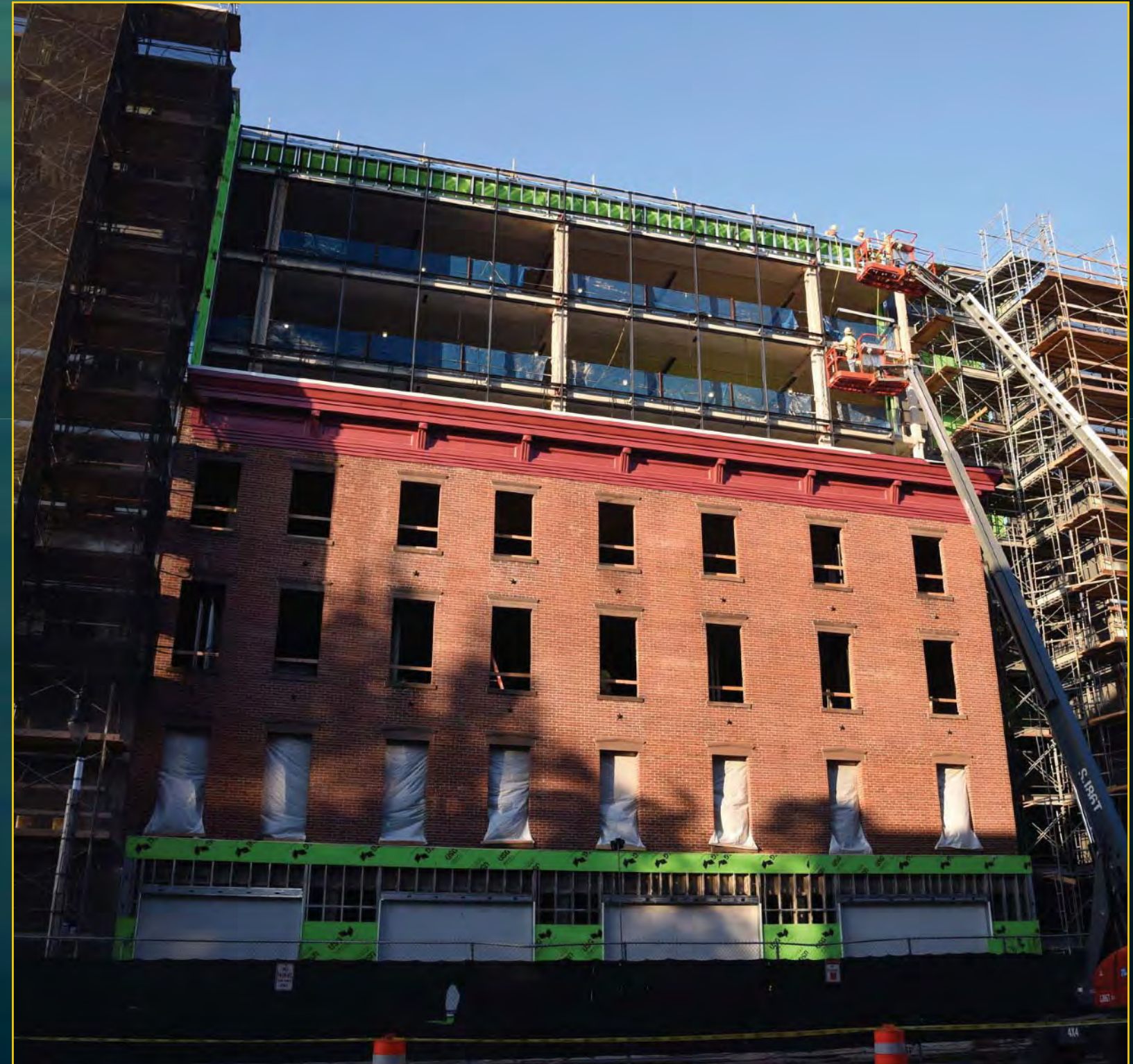
Union Chandler Construction - September 28, 2017
