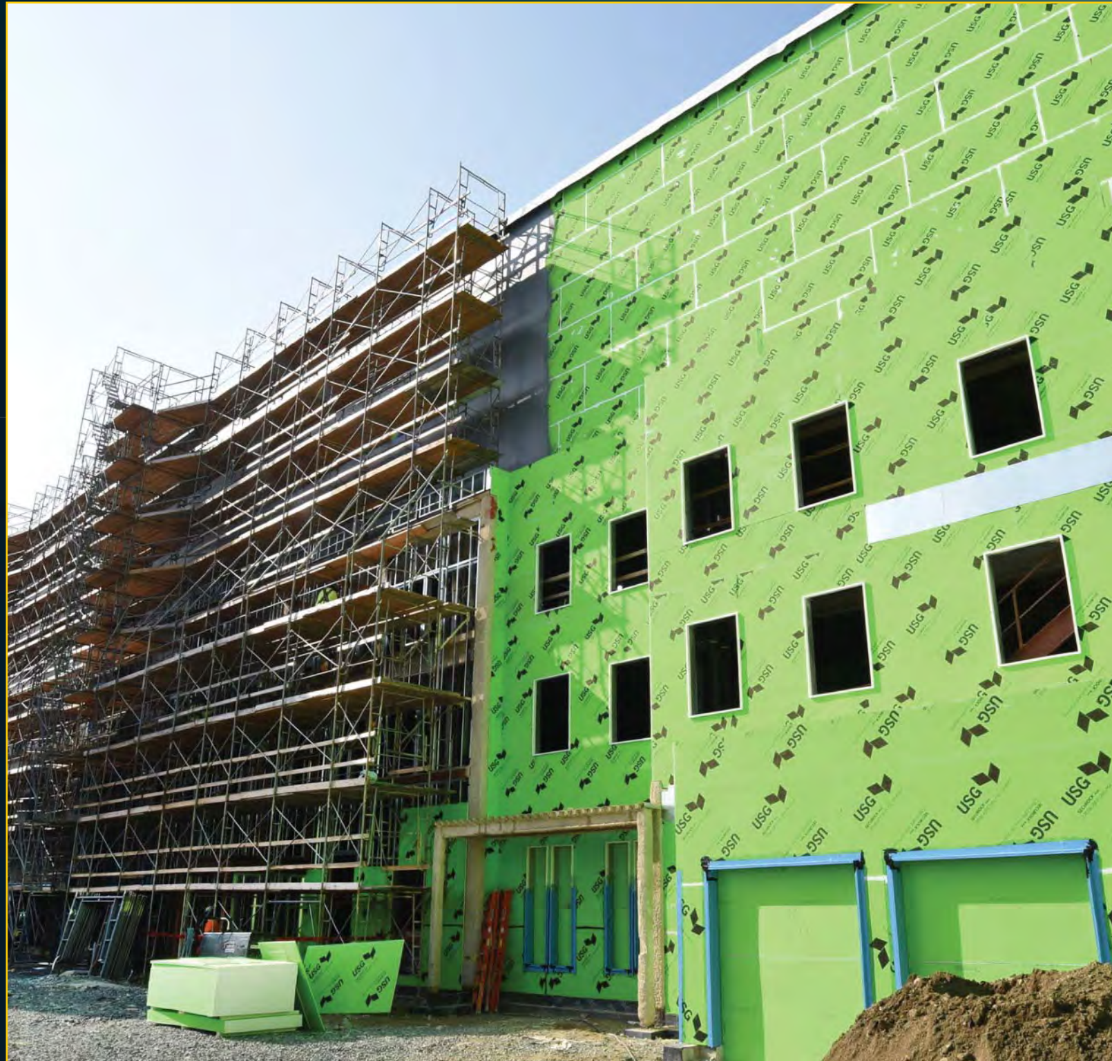
Entertainment Block Construction - August 31, 2017
