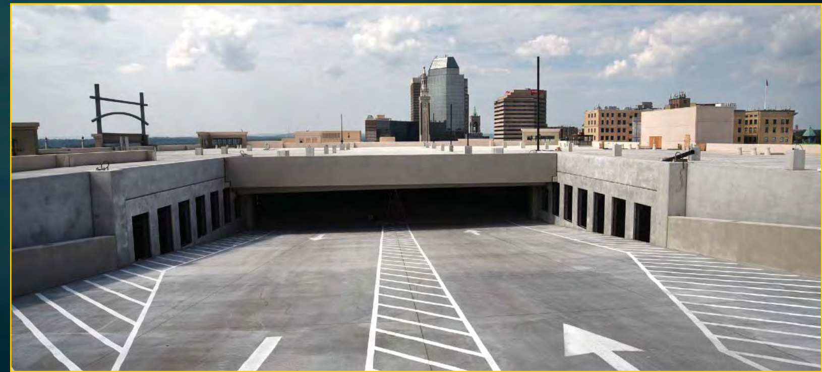
Garage Construction - August 21, 2017
