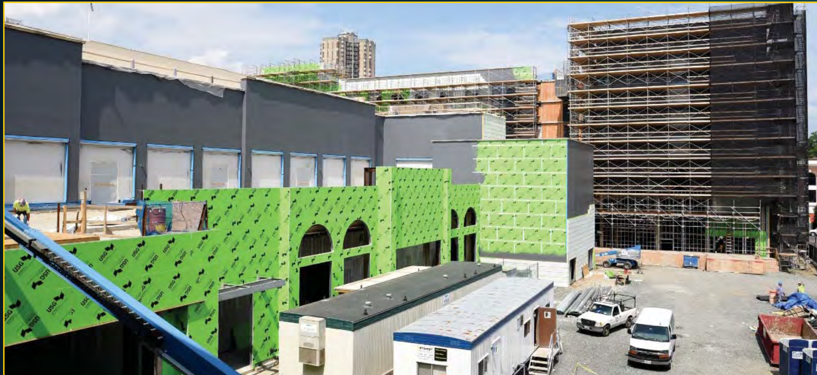
Podium Construction - August 21, 2017
