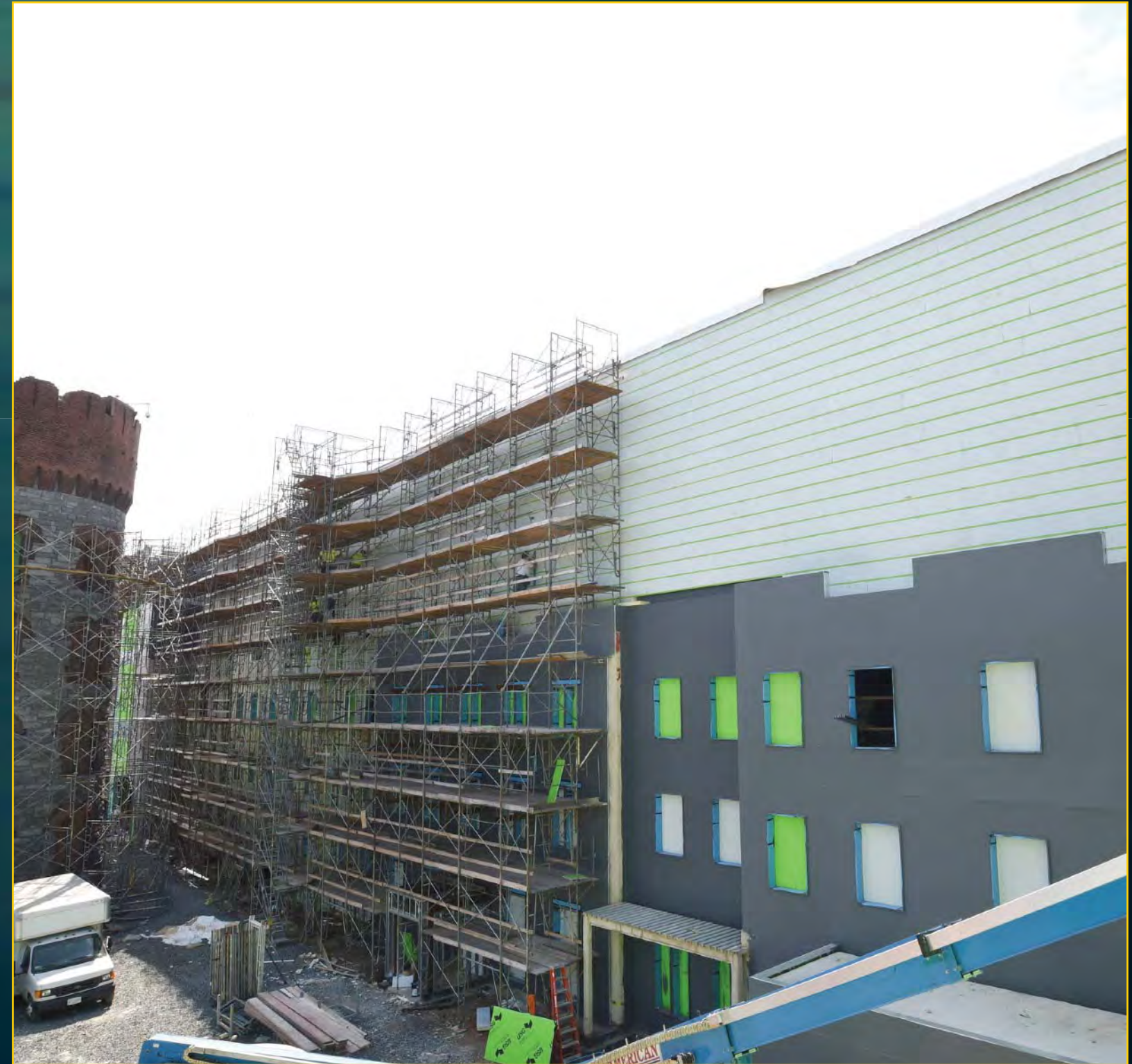
Entertainment Block Construction - September 13, 2017
