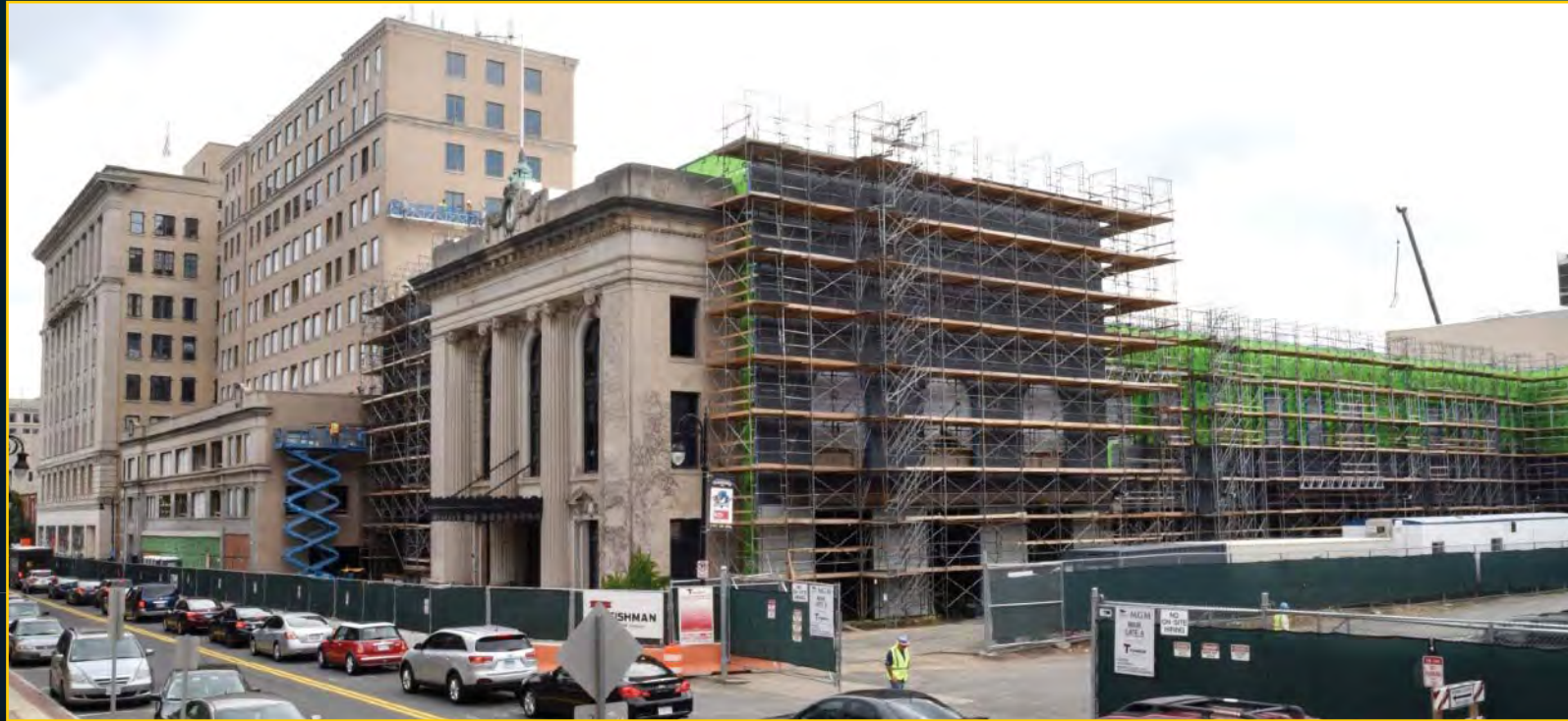
Podium Framing - July 18, 2017
