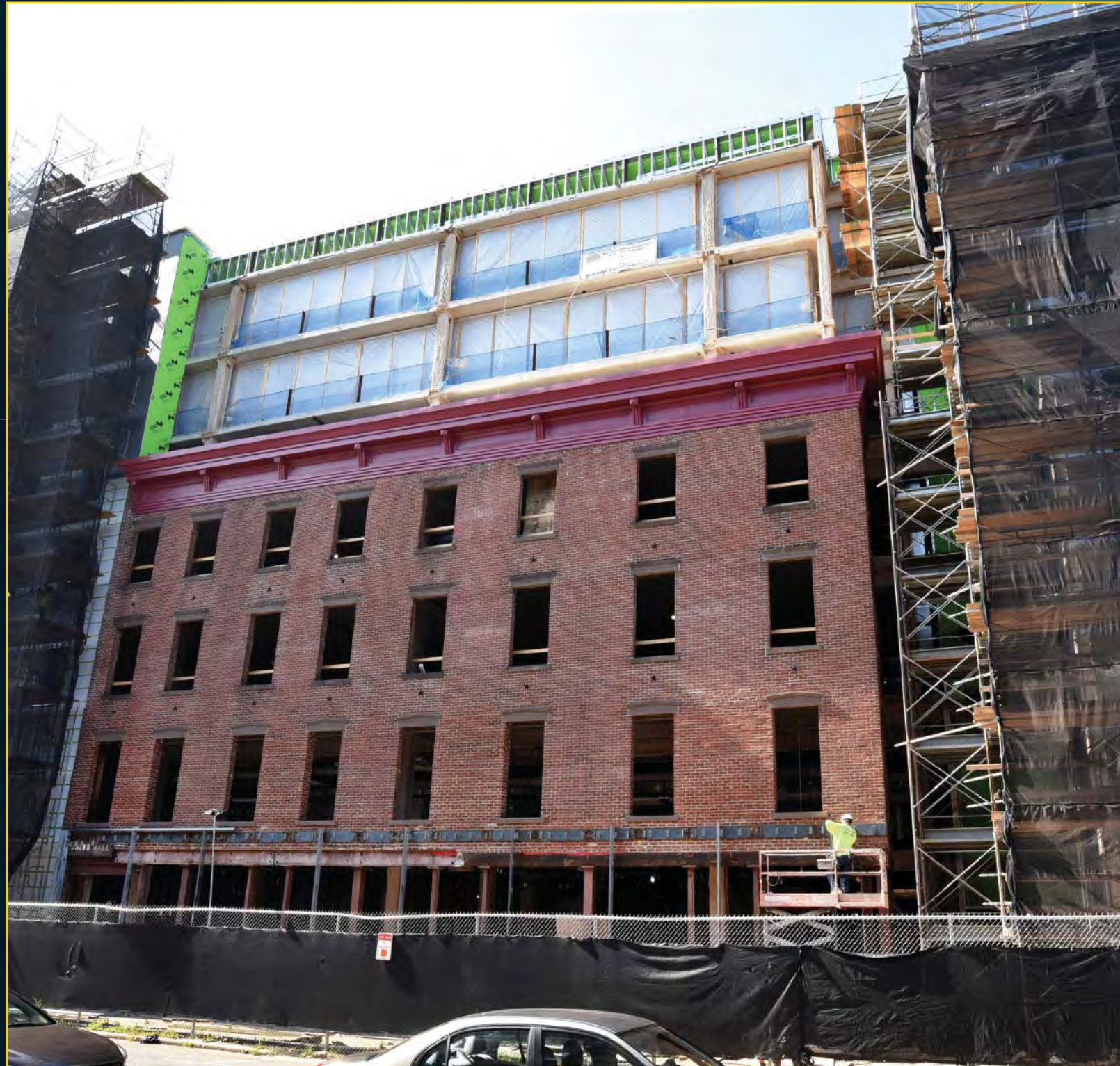
Union Chandler Construction - August 31, 2017
