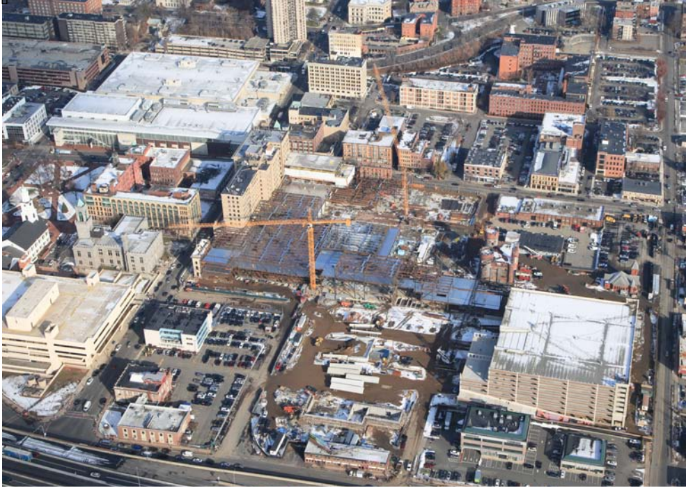
One Year Ago – December 16, 2016 View from River looking Northeast
