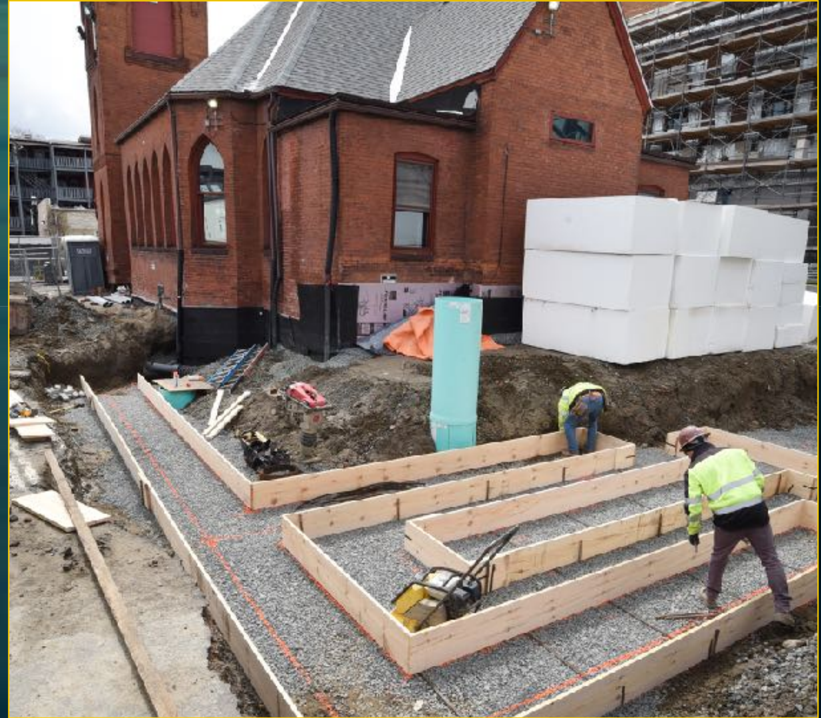
Church Exterior Construction
