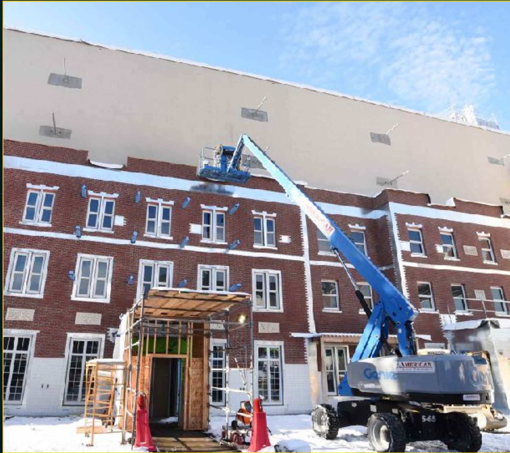
Entertainment Block Facade Construction
