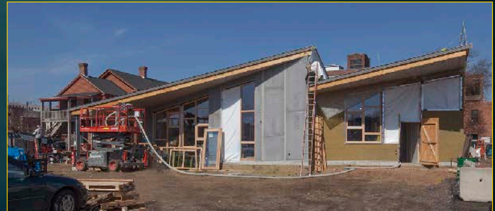
Early Childhood Center Construction
