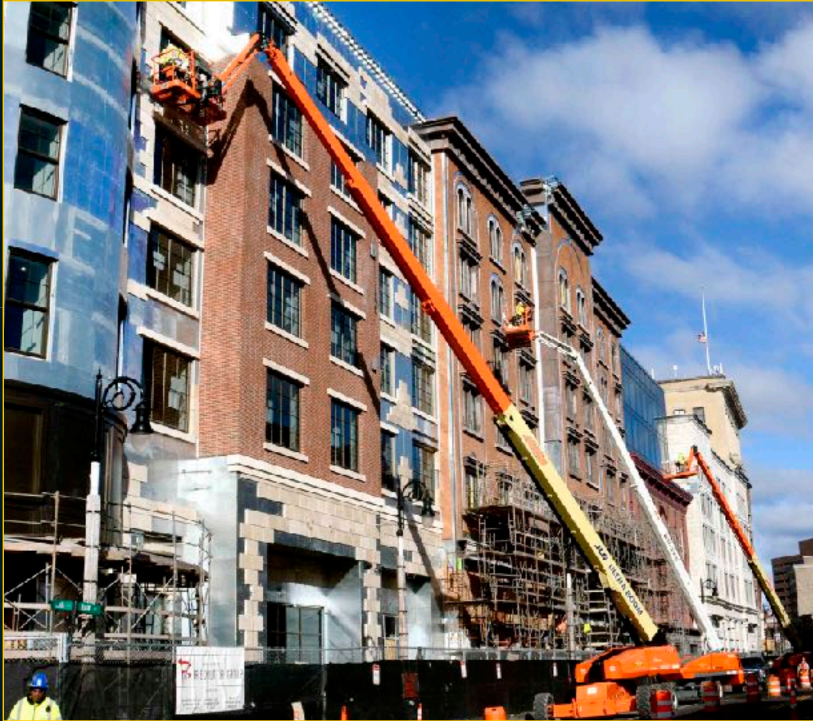
Main Street Facade Construction
