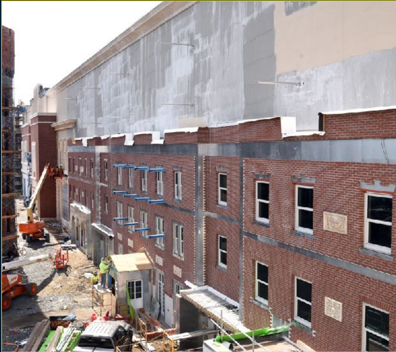
Entertainment Block Facade Construction
