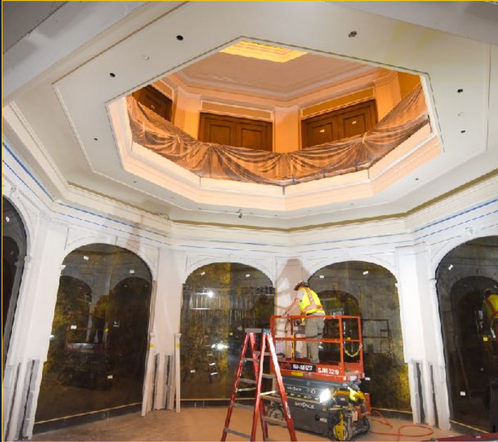
73 State Street Dome Construction
