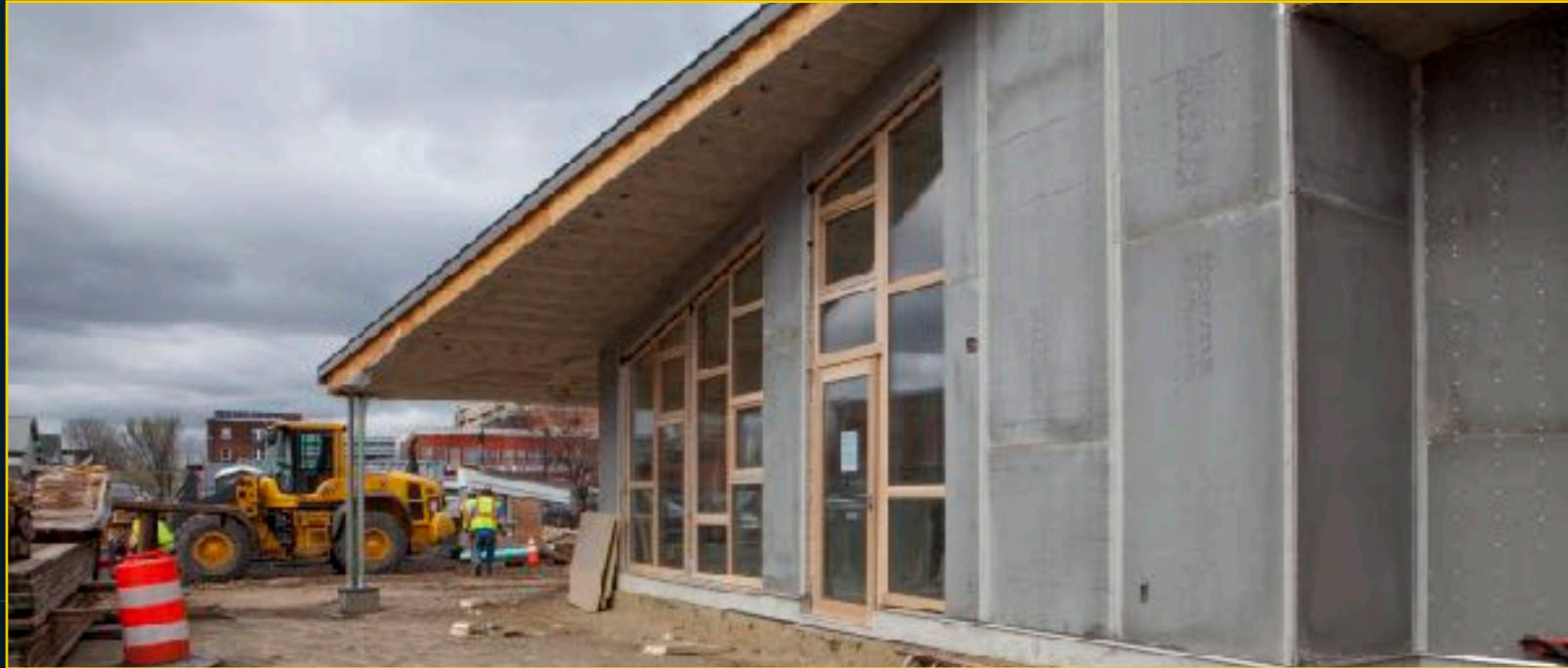
Early Childhood Center Construction
