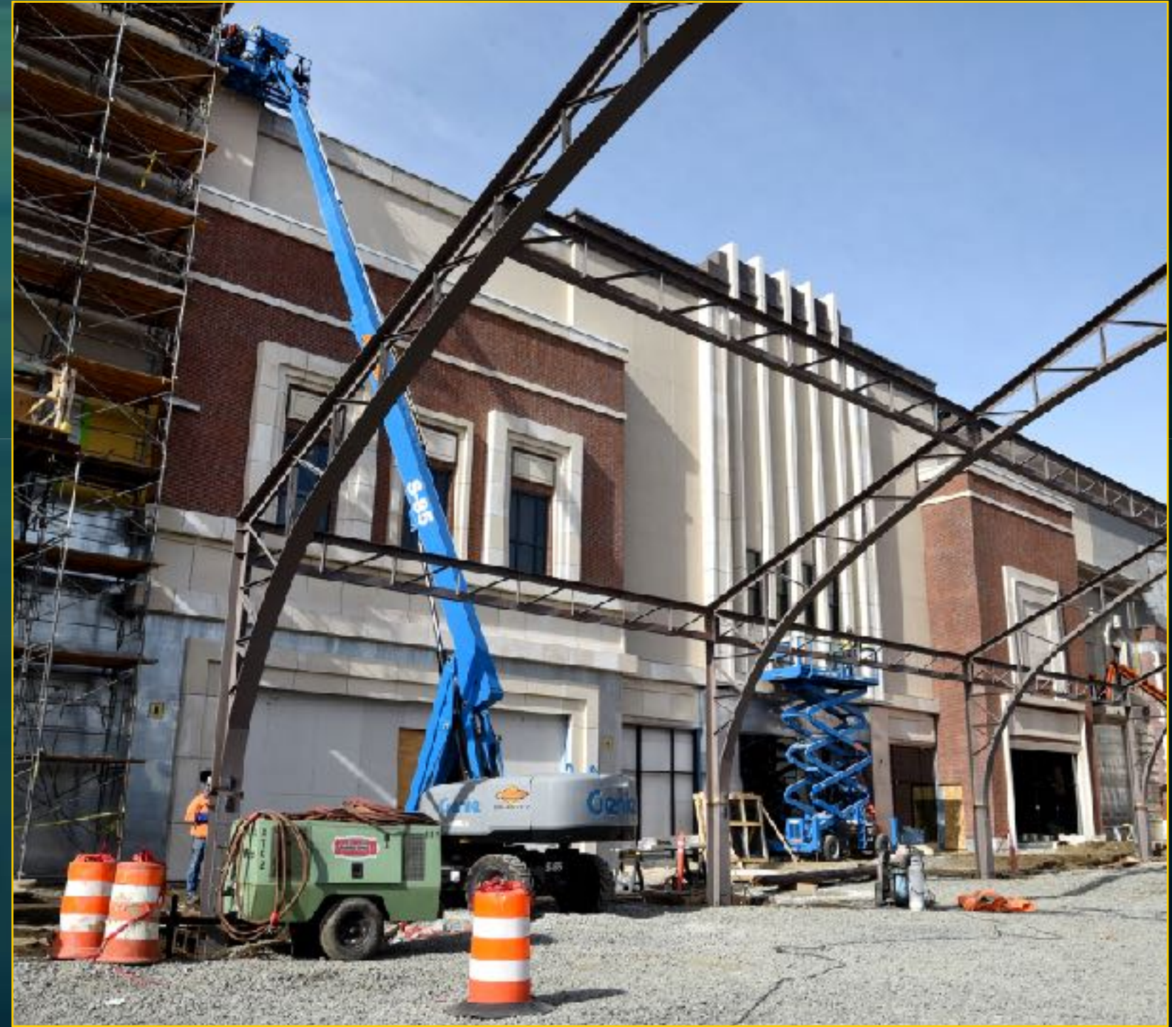
Entertainment Block Facade Construction
