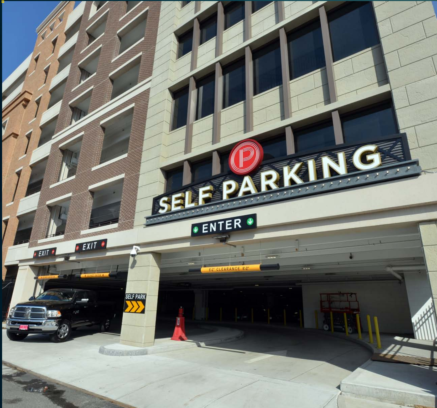
Parking Garage Signage - June 1, 2018
