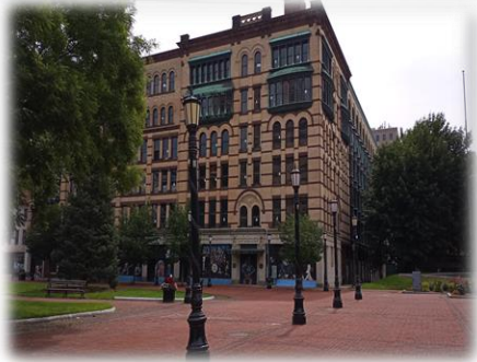
31 Elm – Work Has Begun!
