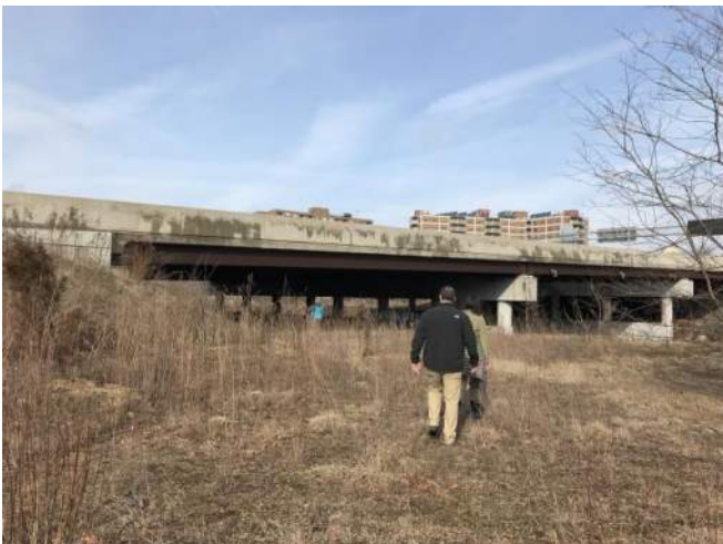
Figure 7. Segment B - Approach to I-93 overpass (south)
