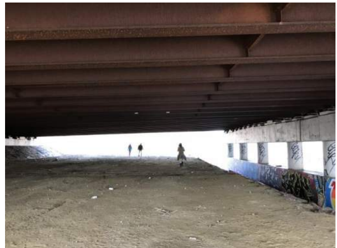
Figure 8. Segment B - Beneath I-93 Bridge
