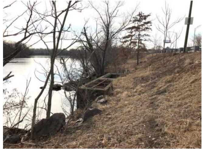
Figure 13. Segment C - Culvert concrete access structure
