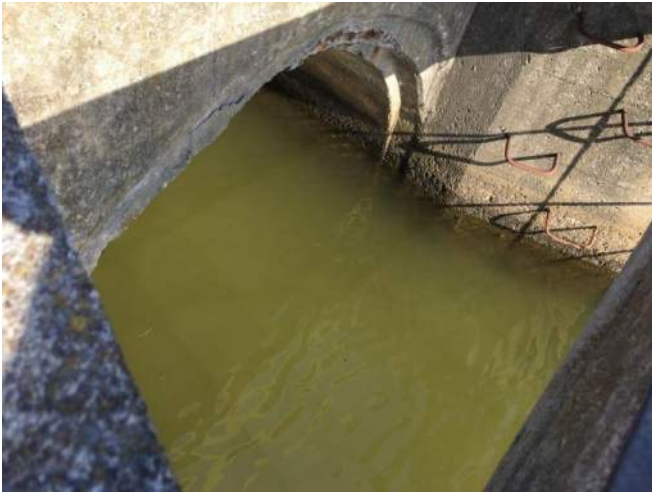
Figure 12. Segment C - Southern culvert opening
