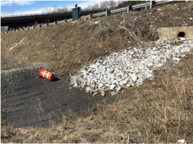
Figure 9. Segment B - Drainage basin adjacent to I-93
