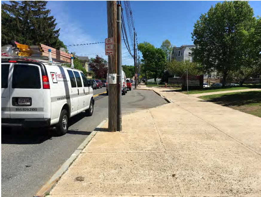
12 - Looking east on West Wyoming Avenue toward the pick-up/drop off area for the Lincoln School
