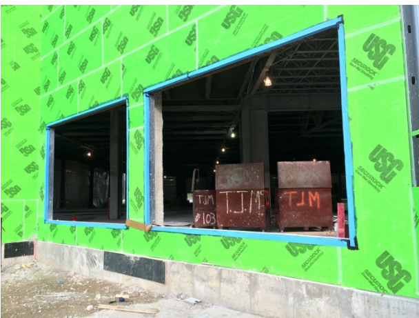
DETAILING OF AVB AT EXTERIOR WINDOWS
