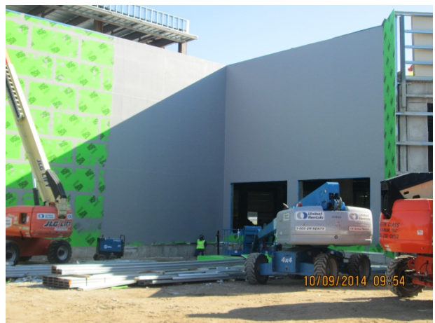
INSTALLATION OF AVB ON EXTERIOR WALLS
