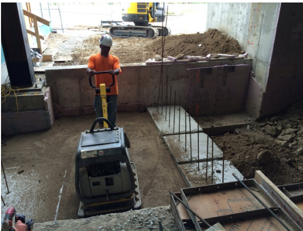
BACKFILLING AT STAIR 9 FOOTINGS
