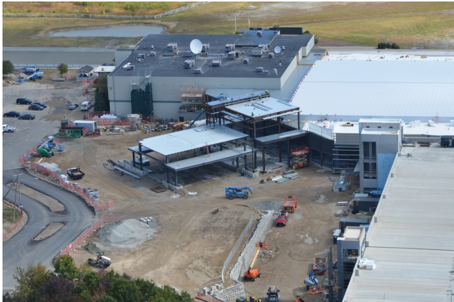
Aerial Photos Taken as of 9/22/14
