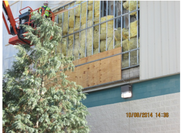
INSTALLATION WALL BLOCKING FOR SIGNAGE
