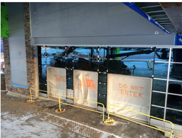
Curtain Wall and Main Entry at Porte Cochere
