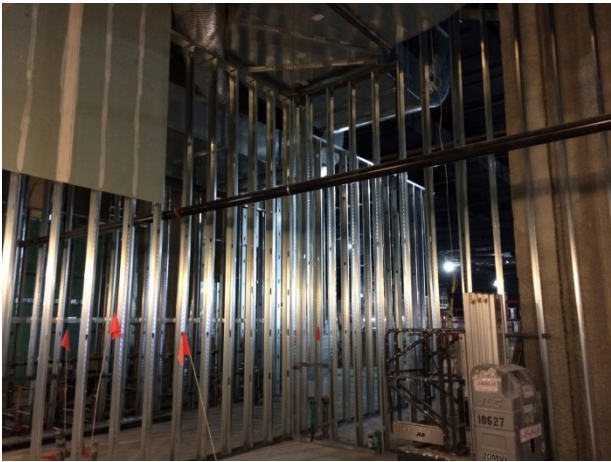
Overall Framing at East Side of Casino
