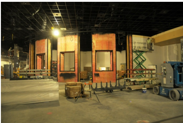
Exterior Work at Fluties Sports Bar
