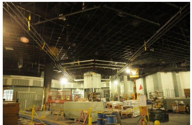
Framing for ceiling Chevrons Toward Casino
