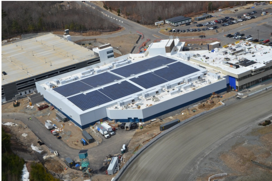
Aerial Photos Taken as of 4/6/15
