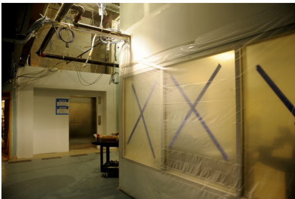
New Elevator Lobby at Track GM Office
