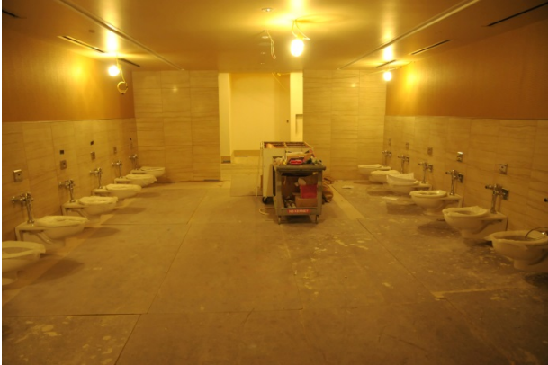
Women's Restroom Adjacent to Stage Area
