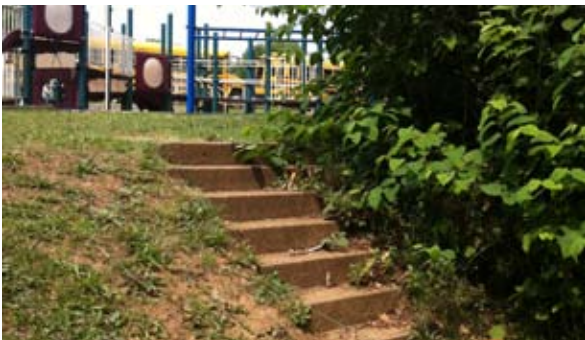
Stairs along the Park's slopes are reminiscent of the past site of Chinquapin Village.
