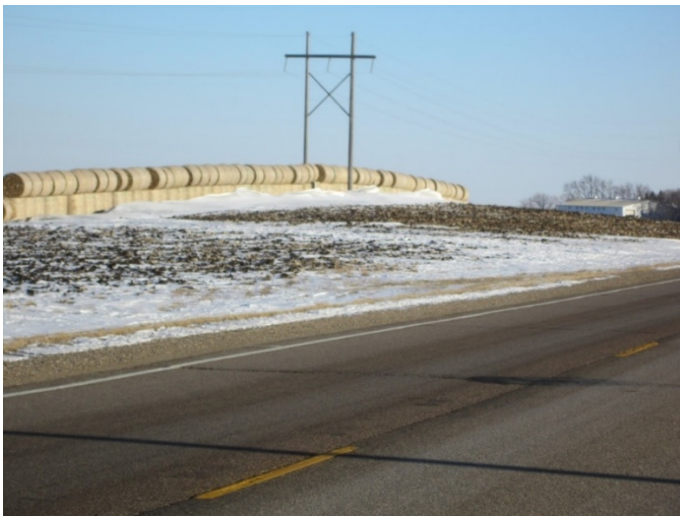
Figure 5. Stacked hay bales to serve as a snow fence along a MnDOT highway.
