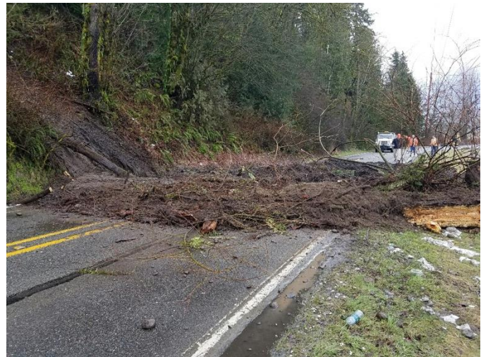
Figure 10. Mudslides in Puyallup (East Pioneer) in winter 2017 after heavy rains.
