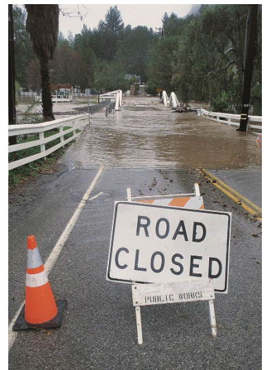
Flooded road. Source: Pierce County
