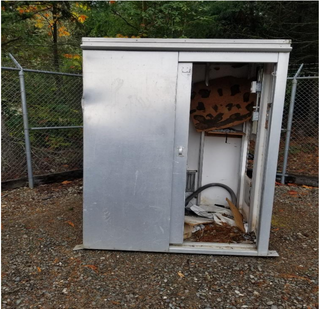
Aluminum building in the back of the Operations Center Yard.
