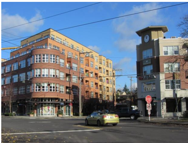
These buildings illustrate two of many ways to handle building corners especially when they are prominent: cut the corner off and add a taller element or extend the corner and step the building back, though they can be combined in other ways.
