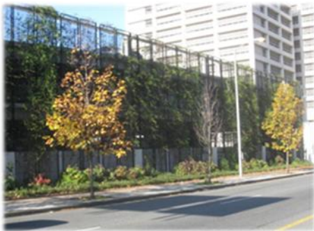
This screening uses both a Green Wall as well as the street trees to visually diminish the impact of the garage.
