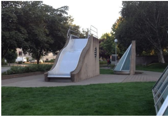
A slide tops a mechanical room for underground parking, a creative and multi-functional use of the structure. The multiple uses enhance its appearance and make it useable for more than just the mechanic.
