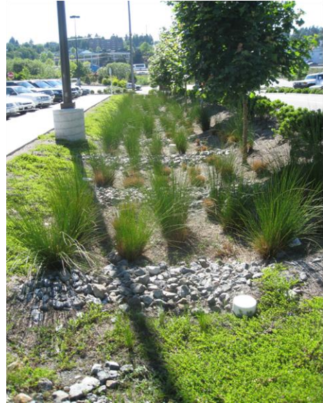
This rain garden is sloped so not only does it hold water but weirs have been used to slow the water's flow.
