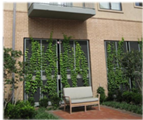
Garage openings have been screened with trellises and greenery that responds to the buildings architectural structure.
