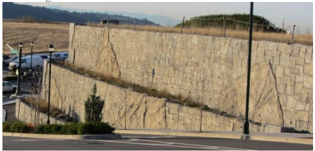
Though the wall materials are inappropriate, the terracing makes a tall wall more appropriately scaled for the adjacent pedestrian while providing key planting opportunities.
