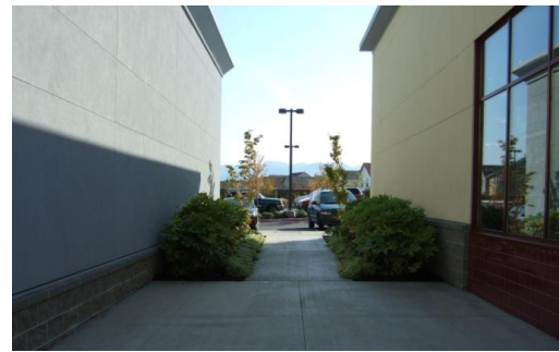
This example of a shared walkway from a sidewalk to parking behind shops, conflicts with many guidelines: the walls are blank, and the overall experience is bland and lifeless. However, the connection is direct and clear, there are planting beds on the last half of the walk which both improves the experience and leaves a wider area for potential future uses near the sidewalk such as café seating. Providing windows adjacent to the shared walkway also improves the experience.
