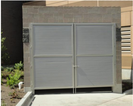
Tall, solid walls screen this waste enclosure. The materials are similar to the building it
