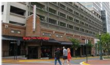
The street level of this garage has both active uses and Pedestrian Friendly design through the use of pedestrian scale materials, weather protection, windows, etc. The weather protection hides the garage from pedestrians alongside the building, and the trellis is an armature for a Green Wall, reducing the presence from other vantage points.
