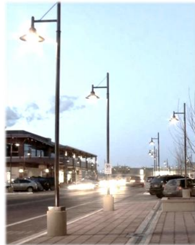
Though the fixtures are too tall, the bulbs are recessed to avoid a bright point source, blinding those driving or walking. The streetlights also form a clear edge between zones for driving and walking.
