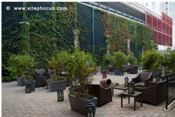
Adjacent to the garage is a plaza. The screens on the garage provide a framework for vines to screen the parking while accommodating natural ventilation and aural connections, improving the sense of safety. Also, architectural elements have been incorporated.
