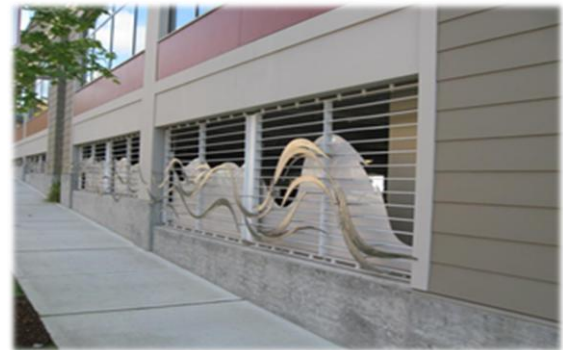
Artwork can be added to screen vehicles in structured parking while maintaining sufficient openings to allow for natural ventilation and good sightlines for security.
