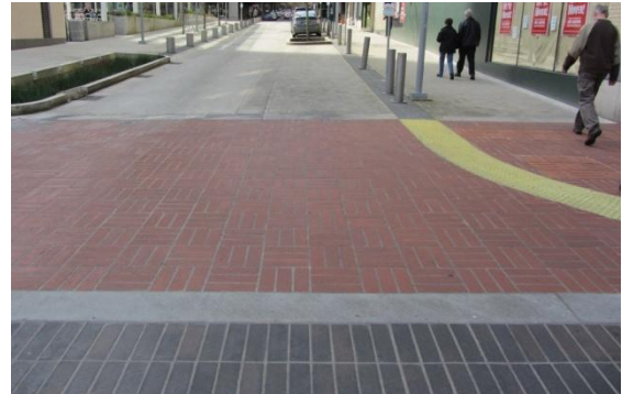
A wide variety of coordinated materials communicate various uses: the dark tiles in the foreground are for cars and mimic asphalt’s color while identifying that this is a special area; the brick colored tiles in the mid ground identify the pedestrian crossing; various patterns of concrete, in a single plane, identify the many types of uses. From left to right they are through traffic, parked cars and pedestrians.
