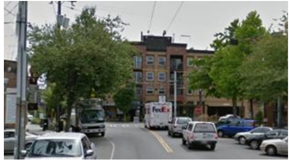
When streets ‘dog leg’ or ‘T’ and the view is terminated, carefully select what will be placed at the end of the axis, such as a park, plaza, building. In this case a building terminates the view and the architecture responds to the vista.
