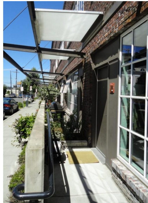
Due to the reuse of a historic building, the setback and front space is narrow; however, this entry illustrates the important components of semi-private outdoor space and residential entries: weather protection at the door, a clear edge defining the boundary of the public space, a bit of room to sit or barbecue, and watch the world go by.
