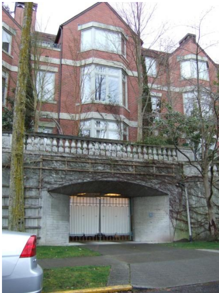
This residential garage is setback with splayed walls that reduce the garage’s presence while improving driver’s sightlines to oncoming pedestrians. Vines and trellises soften the walls.
