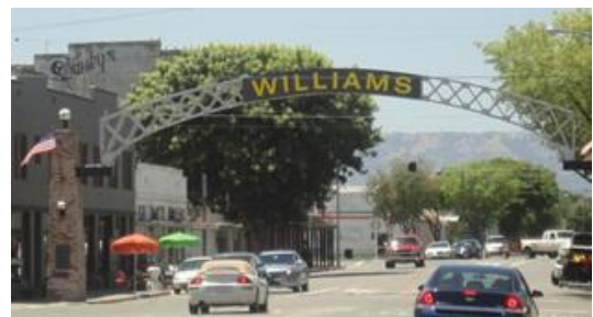
Markers do not have to be as literal as this one, but piers and other identifiers that mark entry to the Project and/or a Neighborhood can be important to creating memorable and identifiable places. Other elements may be used throughout the Project to achieve the same goal, rather than just marking entry points.
