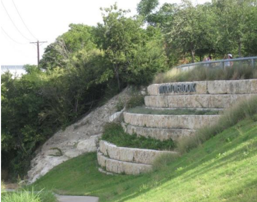
Large blocks of local stone terrace up, holding a steep hill while offering planting beds that soften the walls' mass. An overlook is located atop the wall.
