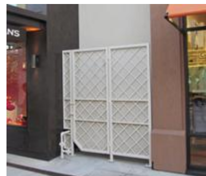
An example of an architectural screen tucked along a retail frontage, where buildings have to be ‘four sided.’
