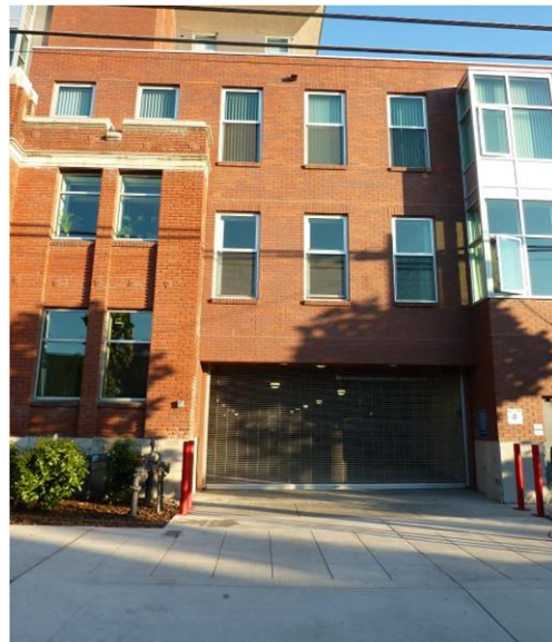
The building is designed with a series of projections that extend in front of the garage entry, minimizing its presence to a pedestrian using the sidewalk, while not obscuring its presence to the driver. Residential buildings such as this one may have gated garage entries.
