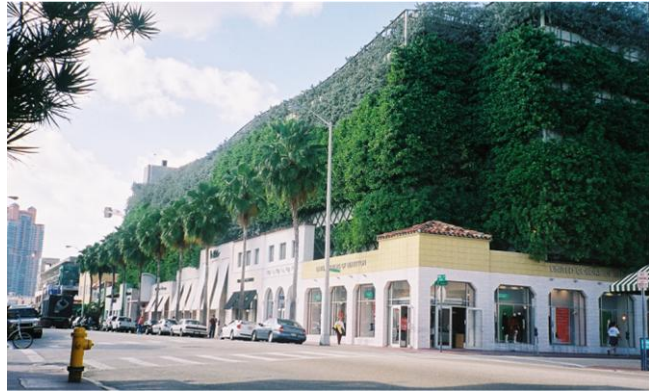
The ground floor retail appears to be built into a green hillside, which in fact is a densely screened parking garage.
