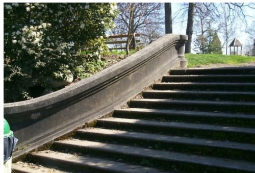
The design of a stair should further the character of the area. For instance, the wooden stair blends with the wooded hillside. Its steep rise, makes the overlook an important viewpoint and resting spot. The stair from a park is designed to reinforce the area's more urban character while gracefully transitioning up the slope using Landscape Steps and detailed sidewalls.
