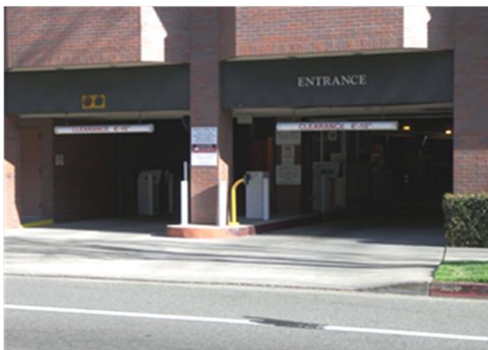
Elements of the building overhang the garage entries reducing the presence of the openings. In addition, by separating the entrance and exit, the post improves the pedestrian experience and decreases the impact of the automobile area.
