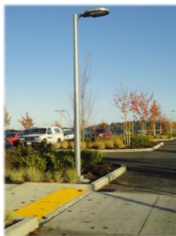
Lighting at a pedestrian crossing.
