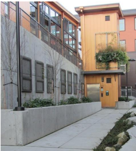
This wall has been terraced in such a way to place the pedestrian scale wall close to people and the taller wall further away. Trees, and trellises for growing vines, soften the taller wall.
