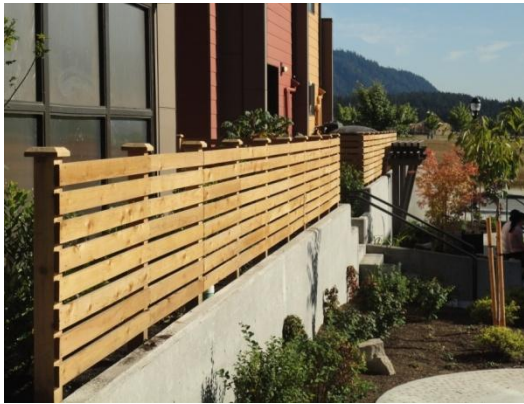
Where fences are needed atop tall walls, use a fence design that compliments and lightens the wall, rather than making it more massive.
