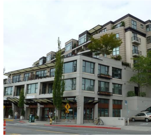
This mixed use building includes accents at the individual business entries on the ground floor. Numerous windows, weather protection, and balconies encroach into and engage with the sidewalk, making the street more interesting for pedestrians.
