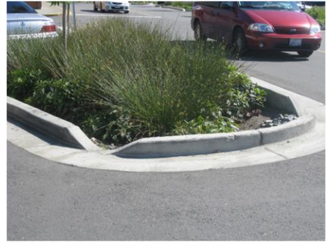
Planting in parking lots should be interesting and may be multi-functional where possible, such as this one used for a rain garden.
