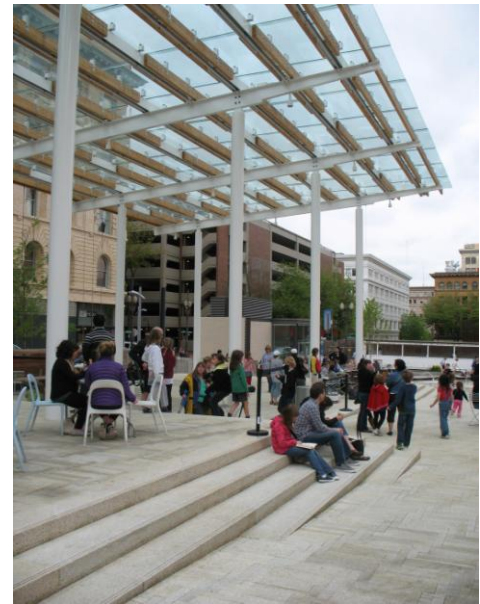
Weather protection can be provided in some Community Spaces. This may come from freestanding structures, such as this pavillion which can also be used after dark, or less formal options such as a pergola.
