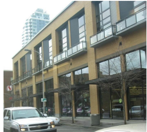
This building exemplifies many of the guidelines for Village Center buildings: the street level has large windows for the retail while the windows on the residential level are finer grained, communicating the different uses inside. The street-level has ground level ‘modules’ similar to traditional main street buildings. There’s weather protection for the pedestrians and balconies for the residents. The entries that are shown are not well expressed however.
