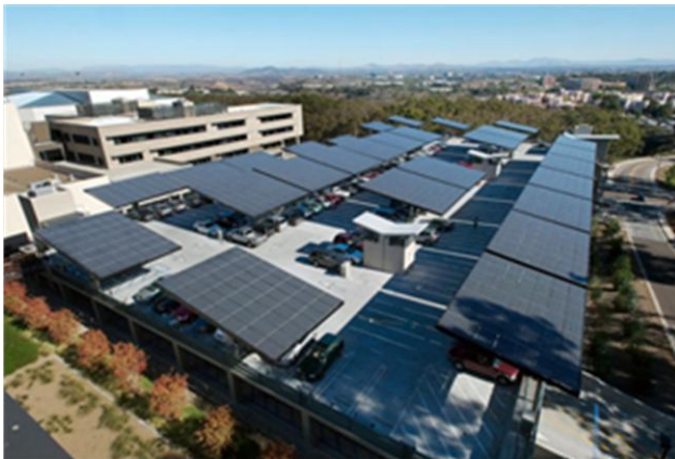
Screening and shading of garage roofs can be provided by solar panels.
