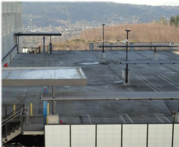
The rooftop lighting of this parking garage is placed central to both give good distribution and to keep the light from spilling to areas other than the roof.
