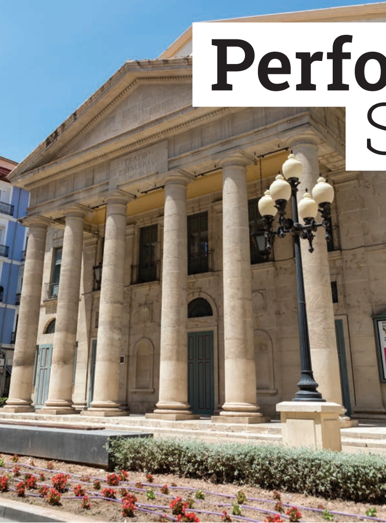
Main Theatre in Alicante
