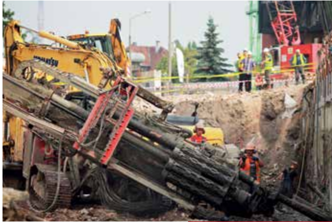
Installing tiebacks to stabilize the walls of the dry pit
