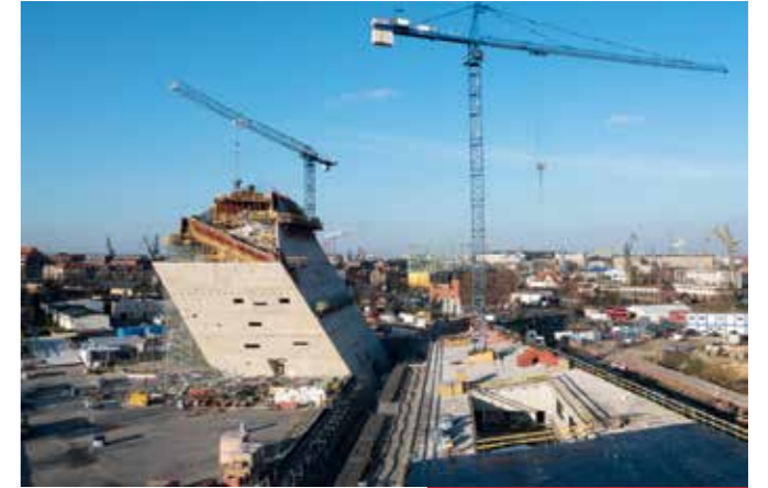
Laying the structural ceiling and constructing the tower
