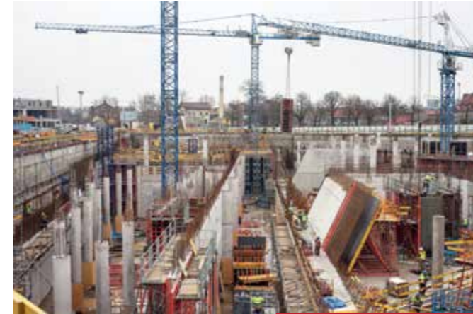
Forming, reinforcing and concreting walls, posts and ceilings
