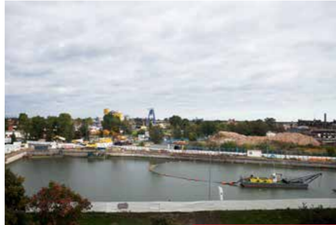
Deepening the pit with suction excavators
