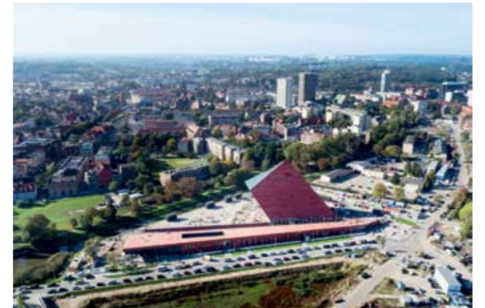
Museum building covered with red lining
