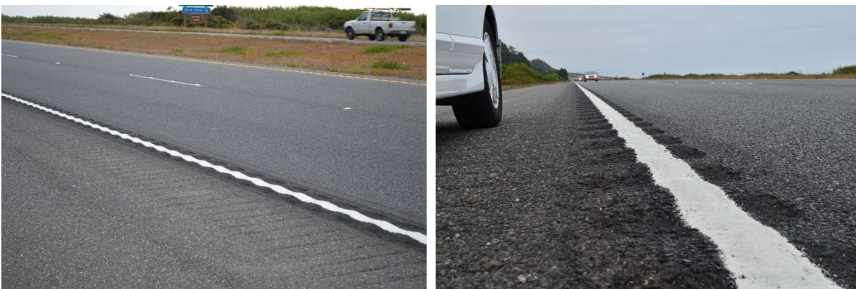
Figure B-3: Photographs of mumble strips installed on U.S. Highway 101
