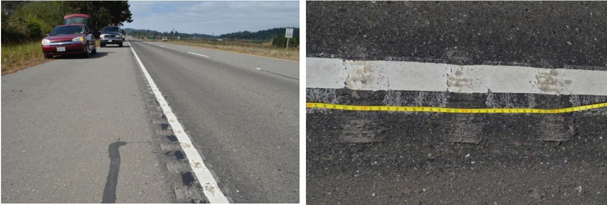
Figure B-2: Photographs of ground rumble strips on State Route 299
