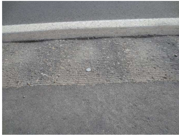
c) Shoulder 14-inch closeup
