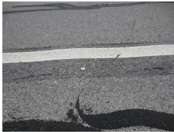
c) Shoulder 24-inch closeup
