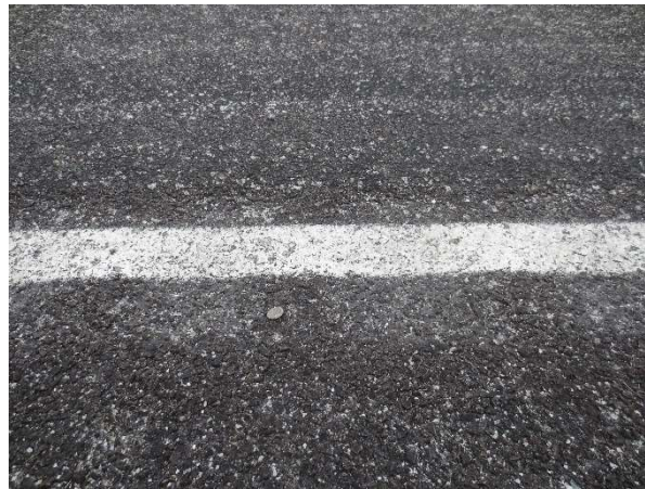
c) Shoulder 12-inch closeup
