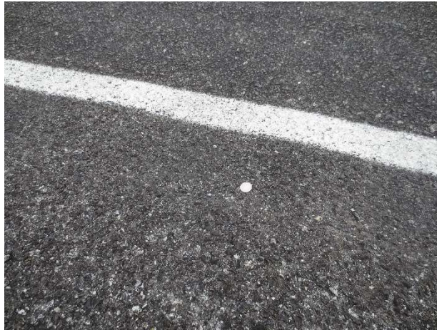
c) Shoulder 18-inch closeup
