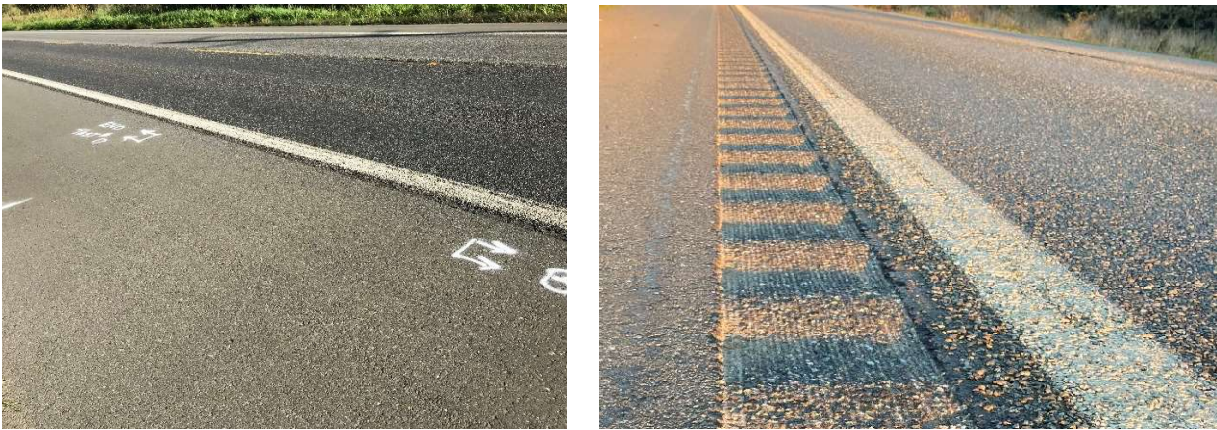
Figure D-8: Pavement surfaces prior to and after sinusoidal strip installation
