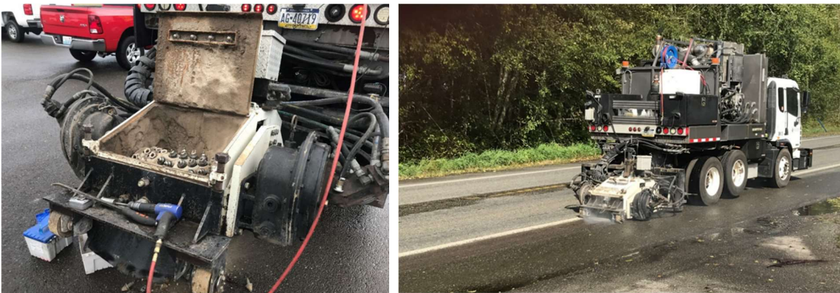
Figure D-2: Milling head and milling operation
