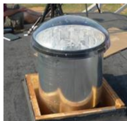
Figure 6: Velux Sun Tunnel Installed
