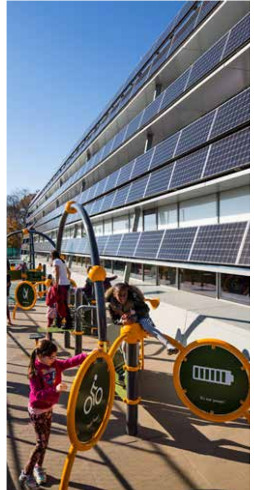
15. Kathleen Grimm School, Solar Panels, Interior, and Gym. Credit: NYC School Construction Authority.
