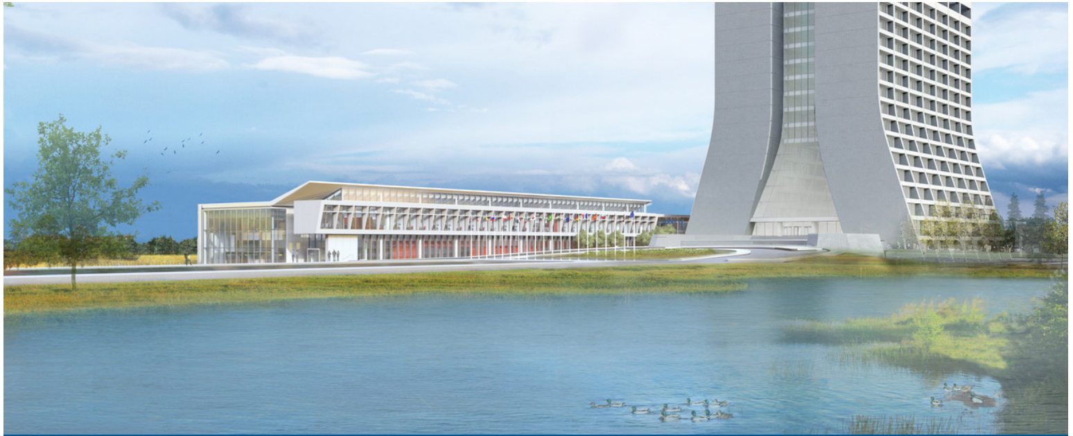
The Integrated Engineering Research Center will be built to the northeast of Wilson Hall and connect to the lab's 16-story office building. Design by Perkins + Will.
