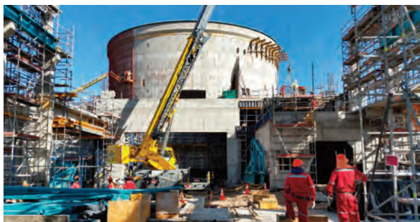
LSST under construction
