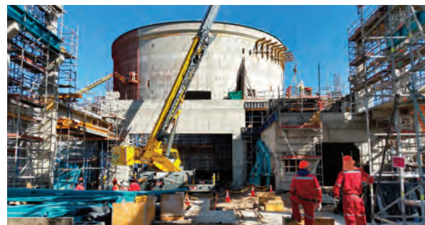
LSST under construction
