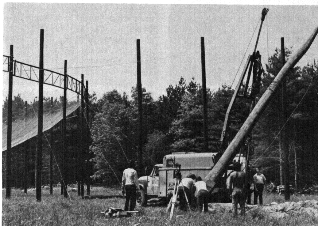
Students raise a 70-foot pole for the feed support structure of the fourth antenna for the Five Colleges Radio Astronomy Observatory. The first antenna, completed and in operation, can be seen at left. (Photo NSF)
