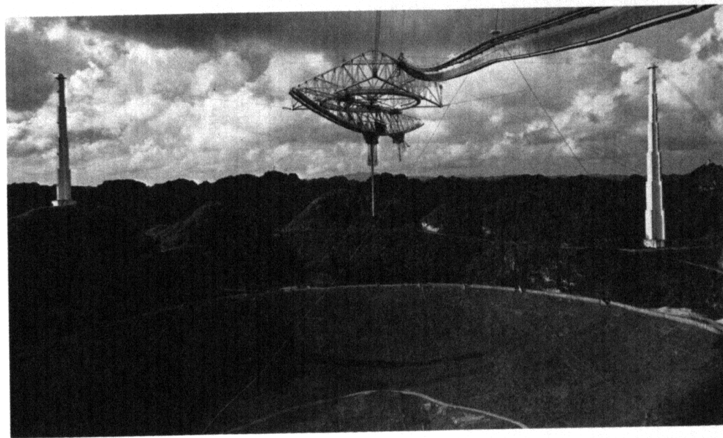
This view of the Arecibo installation shows two of the three towers supporting the feed support structure 435 feet above the spherical mesh reflector. (Photo Cornell University)
