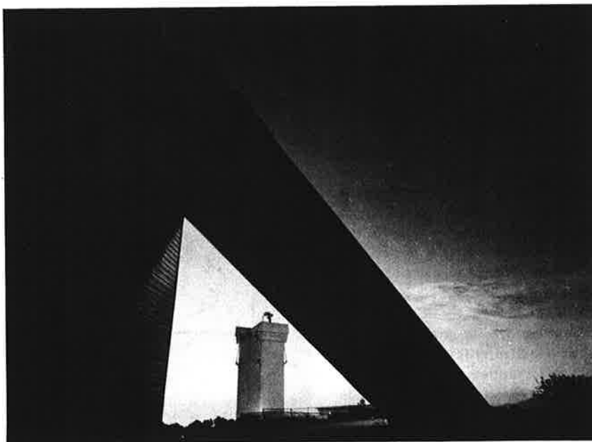
Solar telescopes. Two of the instruments at Kitt Peak National Observatory are devoted primarily to solar research. The triangular McMath telescope is the largest solar telescope in the world; the vacuum solar telescope in the rear has a vertical vacuum tank that isolates the light beam from disturbance by local air currents.
