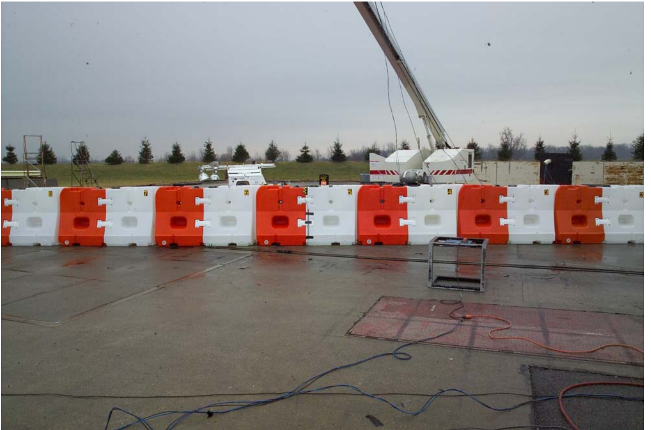
Figure A-38 Pre-Test Channelizing Barricade Impact Side Overall View
