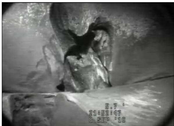
Figure 4.9.9. Erosion in the BOP.
