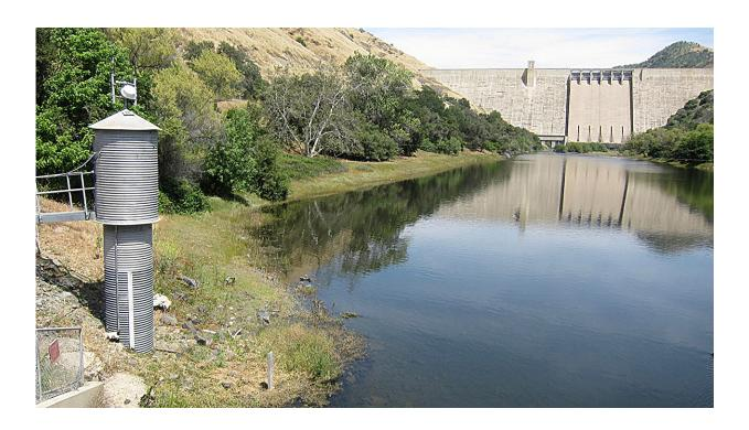
A United States Geological Survey stream gauge measures and records the level of California's Kings River near the Pine Flat Dam in the Central Valley. Credit: University of California - Berkeley
