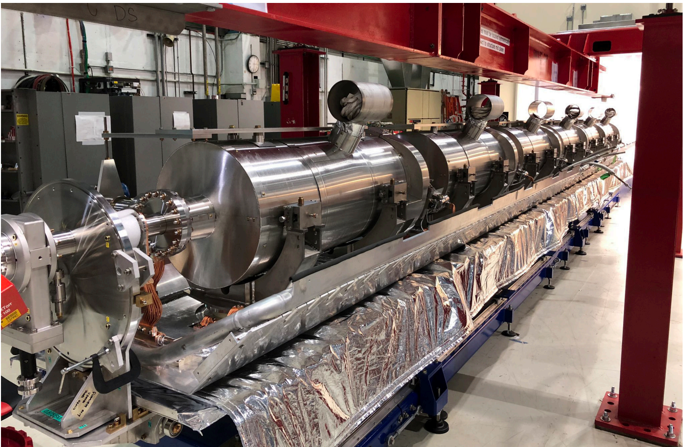
The prototype HB650 cryomodule during assembly, after achieving an important milestone of the string being lowered and mated to the strongback. Photo credit: Charles Grimm
