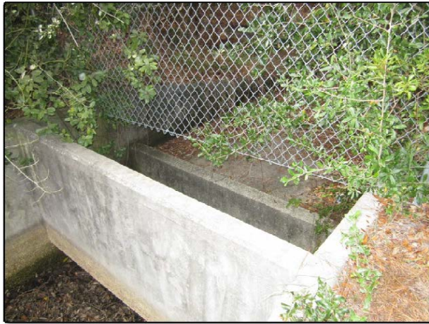
Photograph #1 – Existing [redacted] Subdivision control structure (upstream view).
