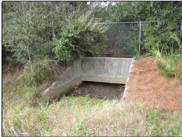
Photograph #2 – Existing [redacted] Subdivision control structure (downstream view).
