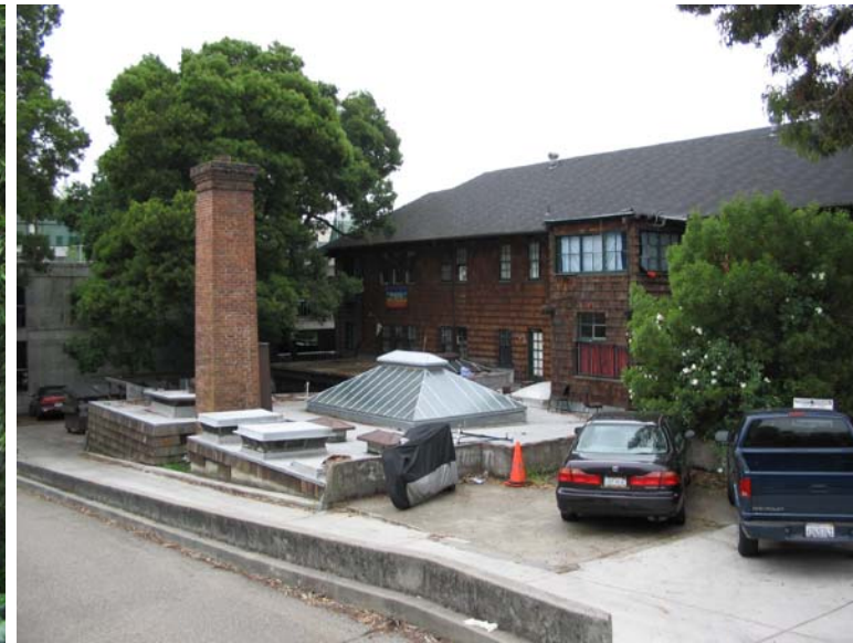
i : Cloyne Court parking ramp / parking / single story component and main building. Existing parking structure beyond.
