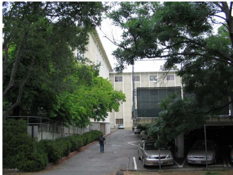
d : existing parking behind Kroeber Hall, exit to service drive.
