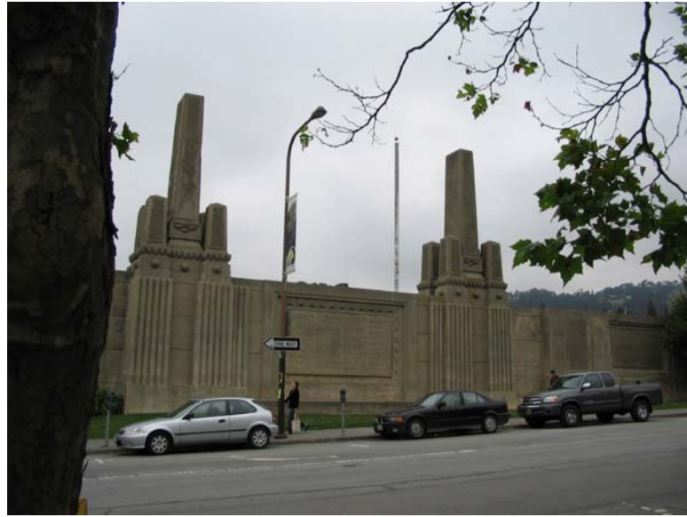
a : Edwards Track Stadium across Bancroft Way.
