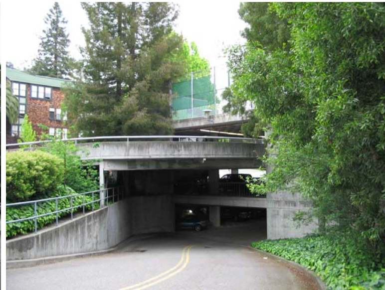
h : bottom of ramp (from Ridge) to lowest level of existing parking structure.
