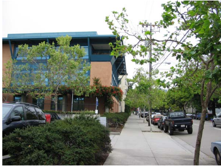
c : Tang Center from Durant Avenue.
