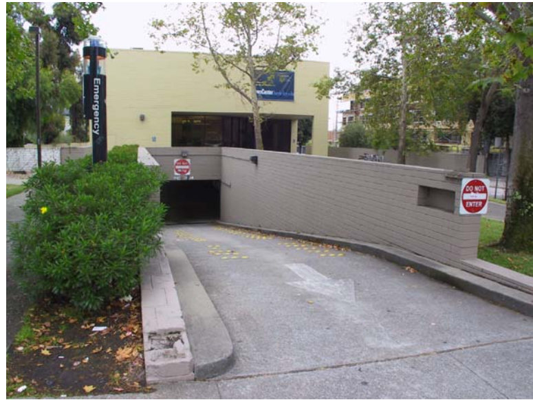
e : Office of Public Affairs Building with parking below, exit ramp to Bancroft (entry ramp on Durant).
