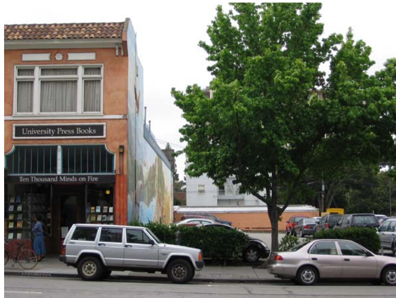
j : commercial building with property-line mural on adjacent lot.
