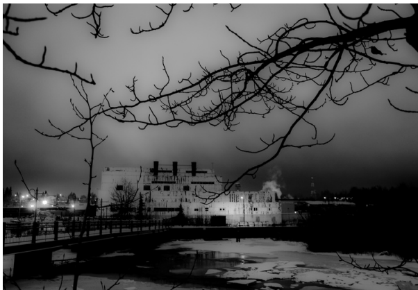
“Power House II”
