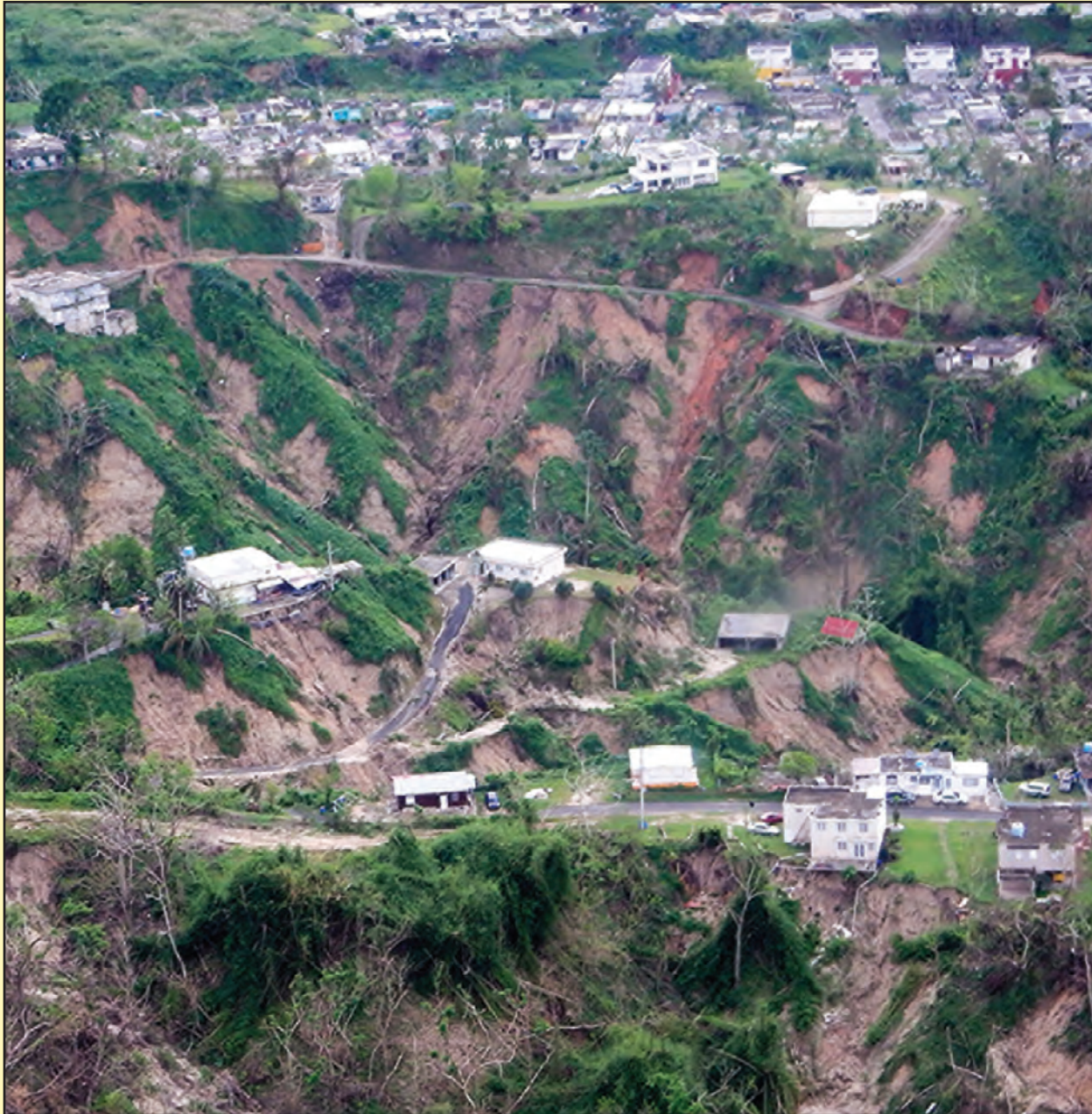
An aerial view of landslide damage after Hurricane Maria in Utuado municipality, Puerto Rico. Photograph by Erin Bessette-Kirton, USGS.
