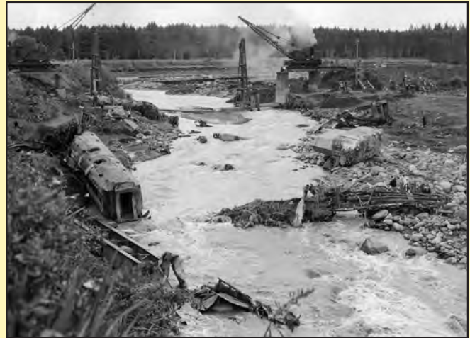
In 1953, a large mud flow was created in New Zealand when a volcano lake held back by a tephra dam collapsed. This mud flow destroyed a railway bridge, causing a passenger train to derail into the river and killing 151 people on board. Photograph courtesy of Archives New Zealand Te Rua Mahara o te Kāwanatanga and licensed under the Creative Commons Attribution 2.0 Generic (CC BY 2.0; https://creativecommons.org/licenses/by/2.0/ ).
