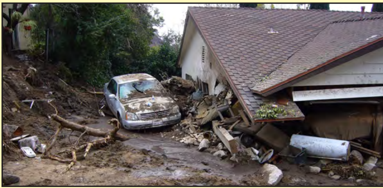
House damaged by debris flows created after a 2010 rainstorm. The drainage basin above this home in Los Angeles County was burned in 2009 by the Station Fire. Photograph by Susan Cannon, USGS.
