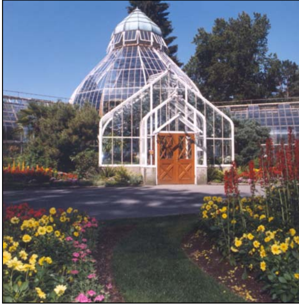
The W.W. Seymour Botanical Conservatory is one of the facilities owned and operated Metro Parks Tacoma.
