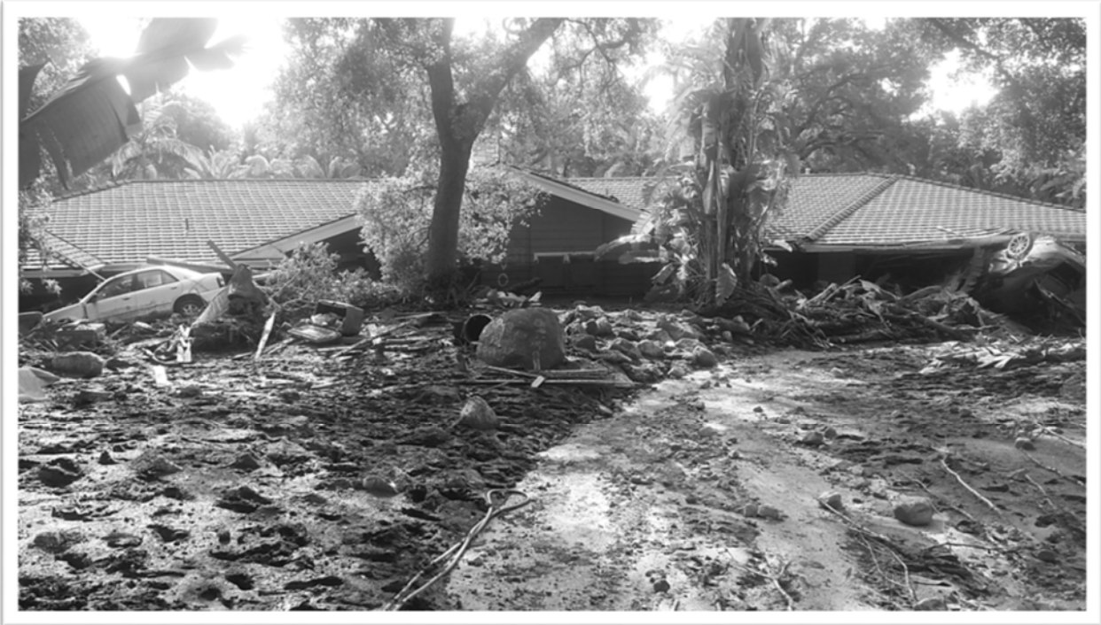
Home impacted by the January 9, 2018, debris flow in Santa Barbara County after the 2017 Thomas Fire (Credit: California Geological Survey)
