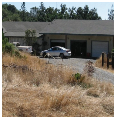
DEFENSIBLE SPACE NONCOMPLIANT
