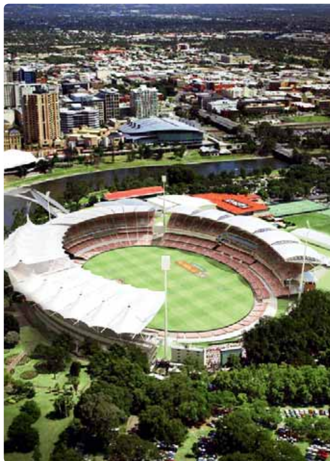
New home: From 2014, all premiership matches in Adelaide are poised to move from AAMI Stadium to the Adelaide Oval, which will be transformed into a 50,000-seat, world-class stadium (see artist's impression above).
